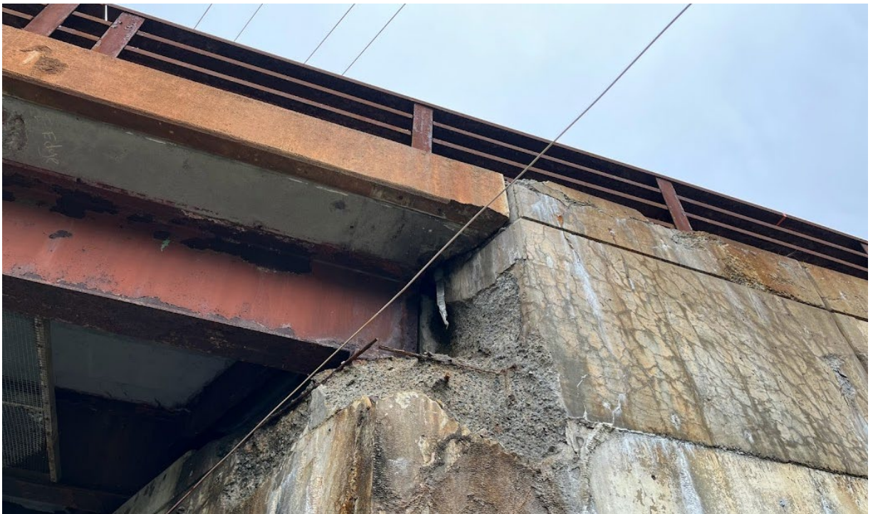
Photo 2: View of concrete decay due to drainpipe storm water discharge, underneath expansion joint. Evidence of bat presence was not found in expansion joints, cracks in concrete, or spaces between concrete walls. Facing Northwest.
