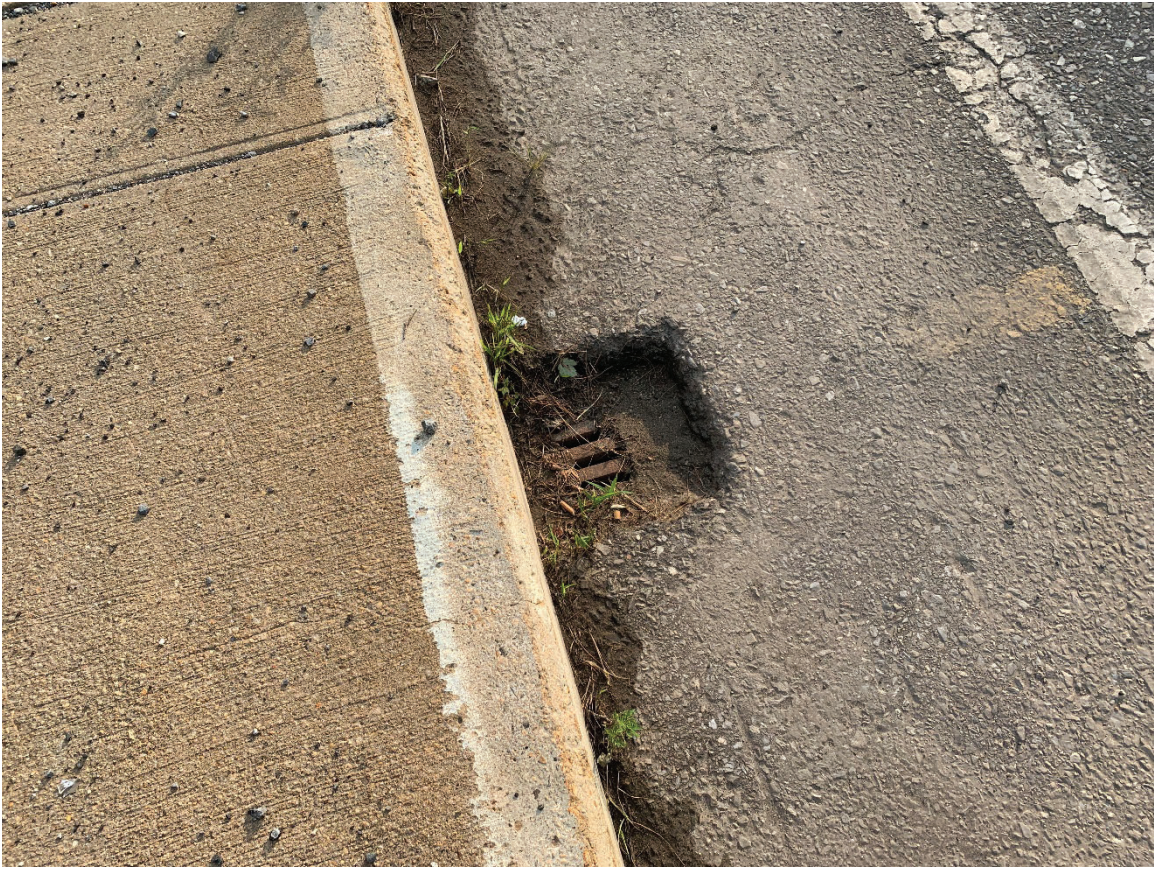
This is the general context of a bridge scupper on the Palmer Road Bridge over the Ware River.
