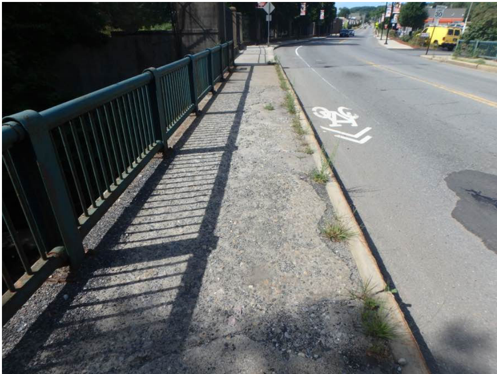
Photo 12: Heavy scaling to the East sidewalk, span #1.
