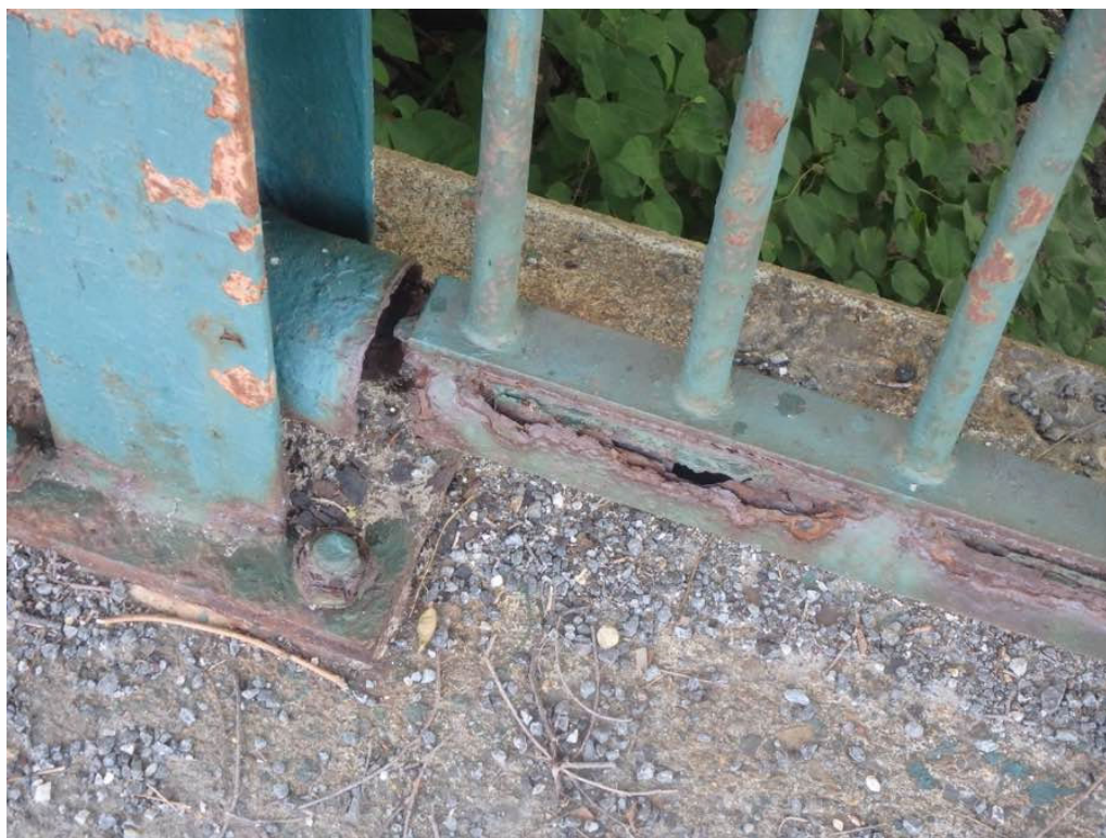
Photo 15: 100% section loss to the bottom rail of the East bridge rail at the North end.
