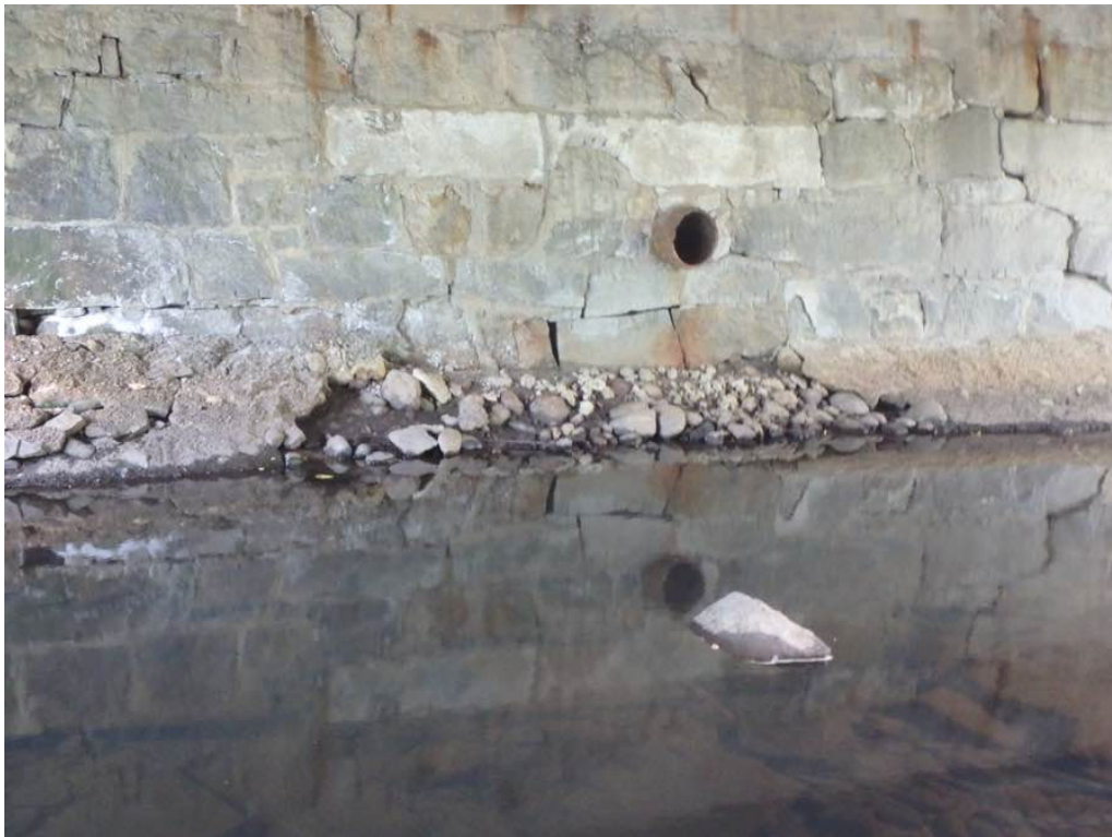
Photo 32: Missing scour protection at the North breastwall.
