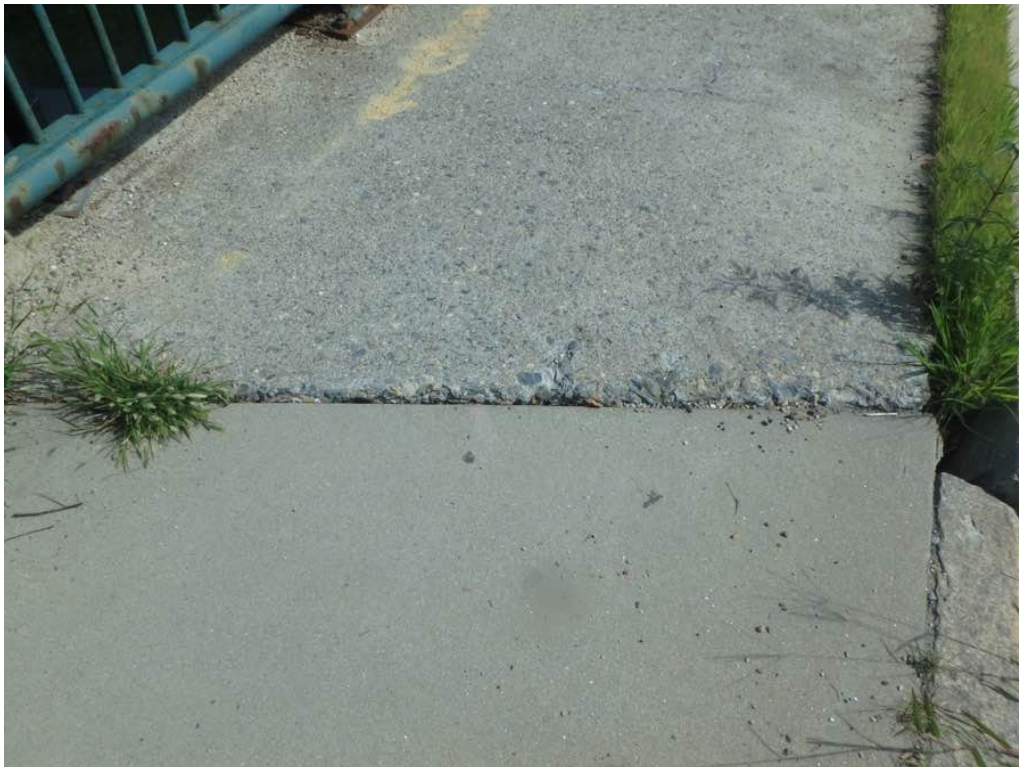
Photo 20: Southwest approach sidewalk settlement.
