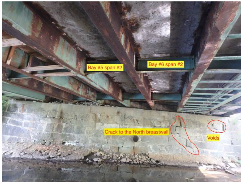
Photo 7: Bays #5 and #6 of span #2. Note crack and voids to the North breastwall.
