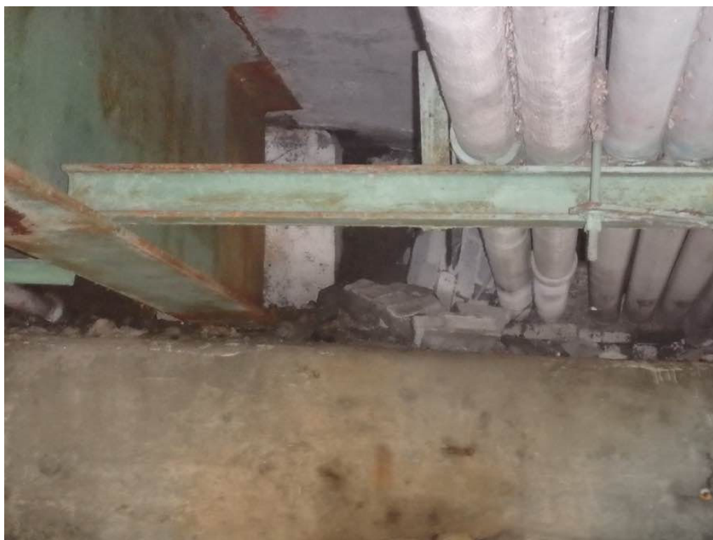
Photo 30: Collapsed brick around utility at the North end of bay #8 in span #2.
