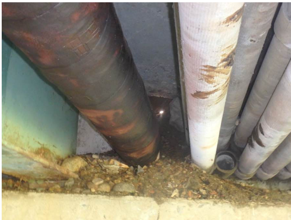
Photo 29: Fill from utility cutout at the South end of bay #1 in span #1. Note daylight.
