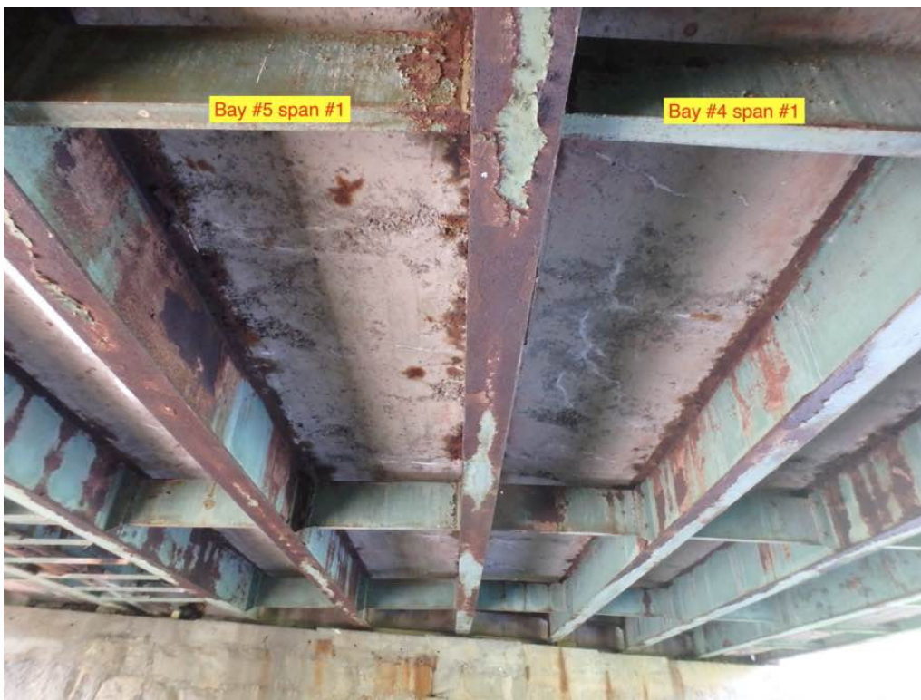
Photo 5: Bays #4 and #5 of span #1.
