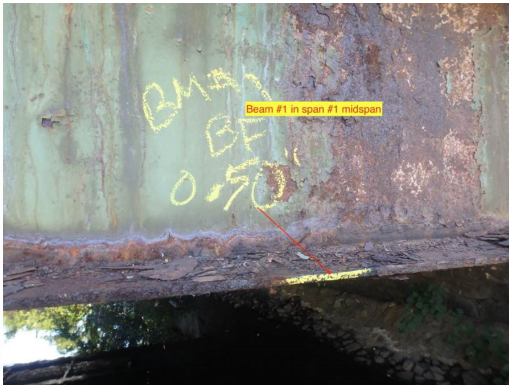
Photo 21: Beam #1 in span #1 midspan.
