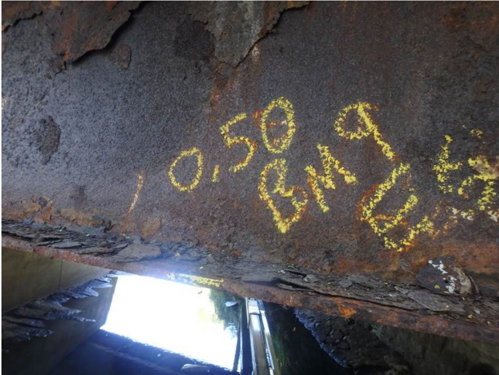
Photo 25: Beam #9 in span #2 near midspan.
