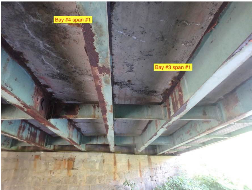
Photo 4: Bays #3 and #4 of span #1.
