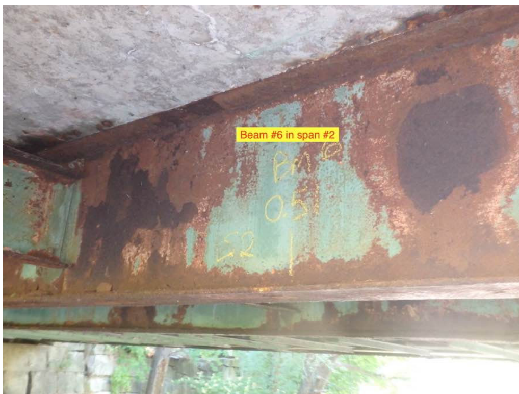
Photo 24: Beam #6 in span #2 near midspan.
