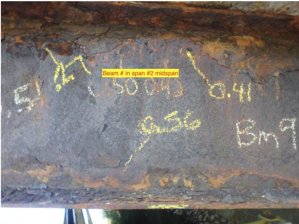
Photo 26: Beam #9 in span #2 near midspan.
