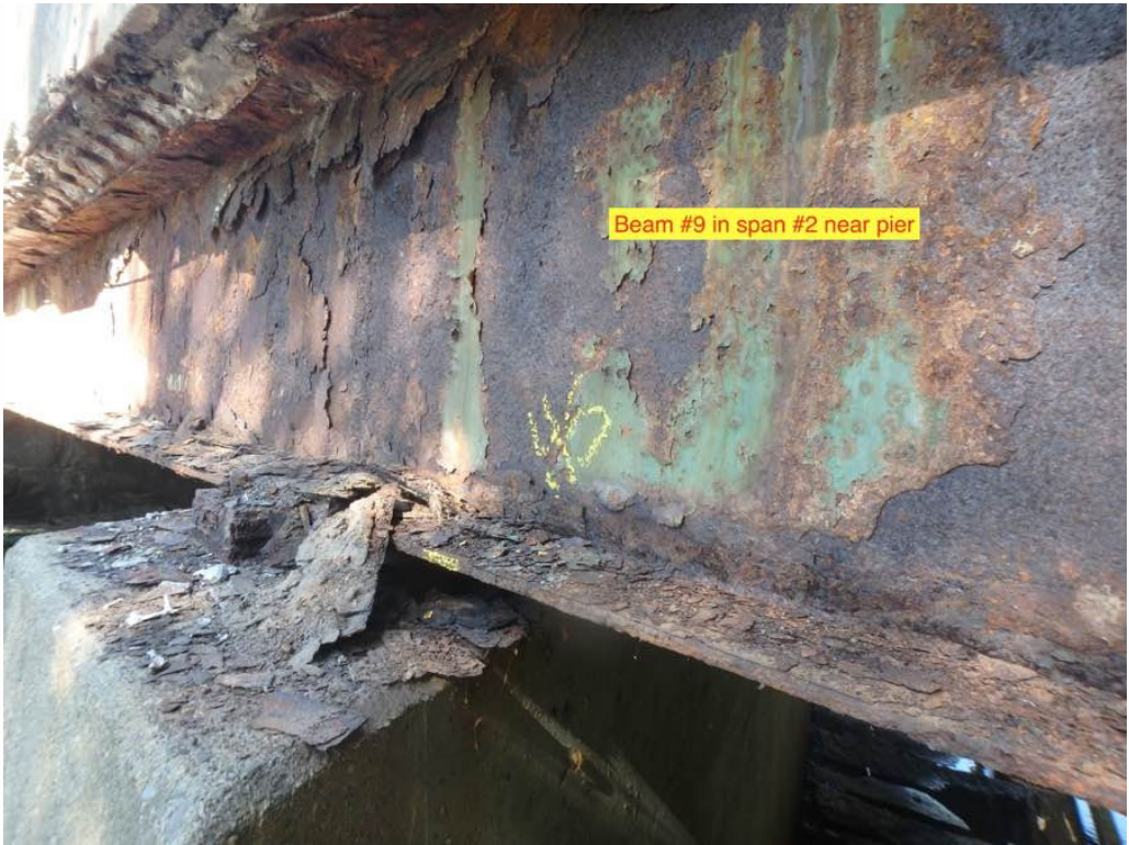
Photo 27: Beam #9 in span #2 near pier.
