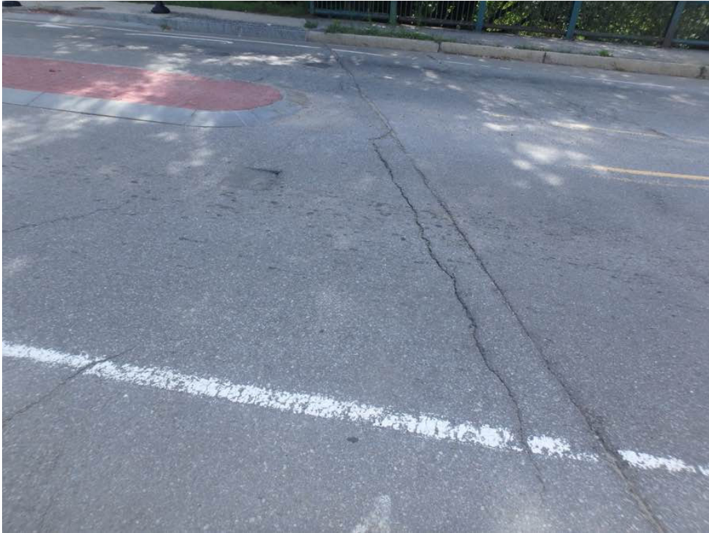
Photo 19: North approach to deck transition.
