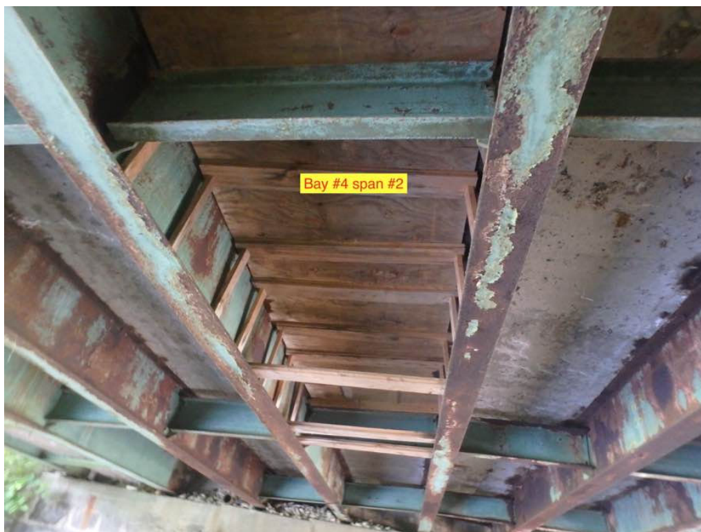
Photo 8: Bays #4 of span #2.
