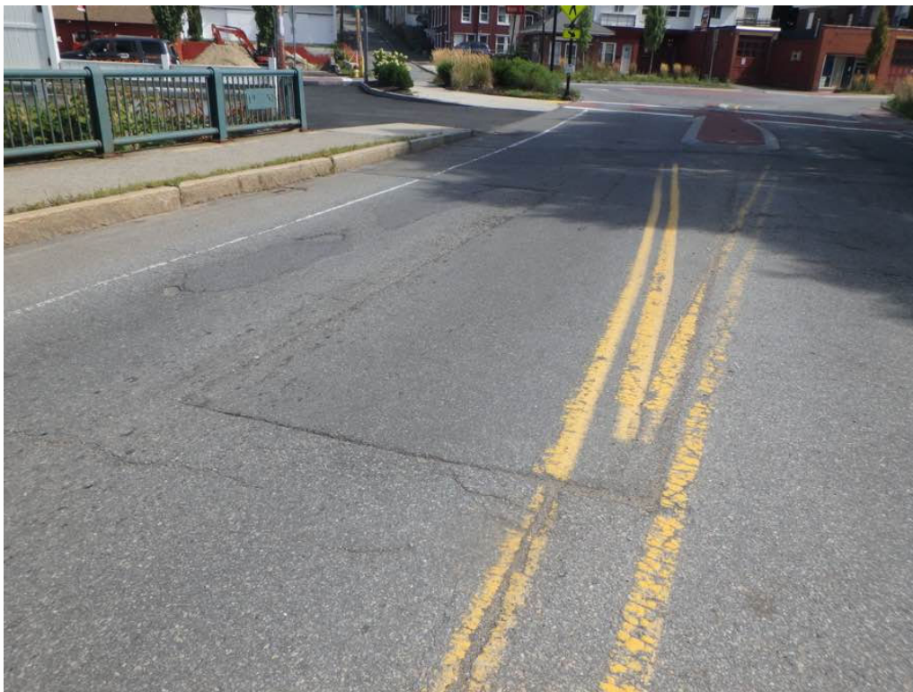
Photo 1: Repair in the Southbound lane at the North end.
