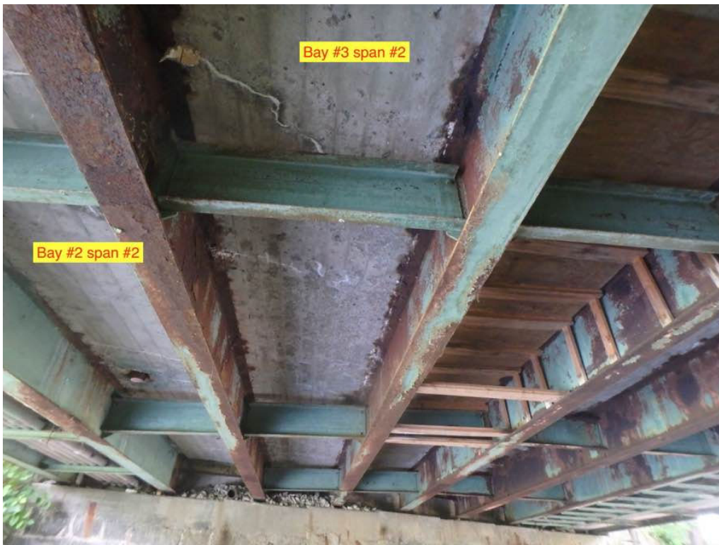
Photo 6: Bays #2 and #3 of span #2. Note scupper drain in bay #2.
