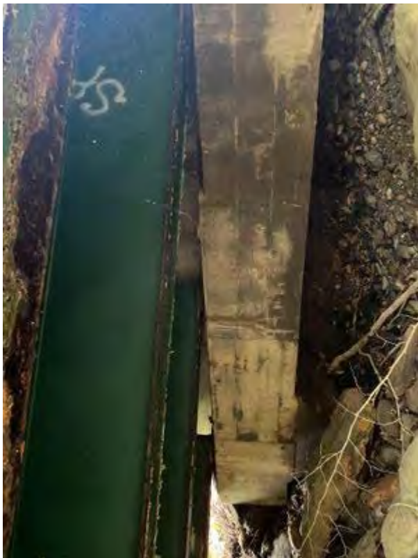
Figure D-61. Project 608858; Segment A – underside of bridge.
