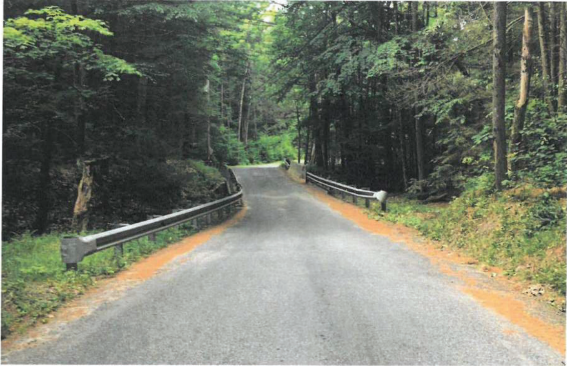
View of bridge facing south
