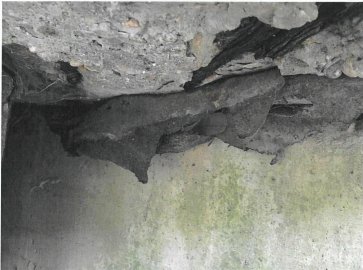
Views of black tar paper at joints along bridge deck
