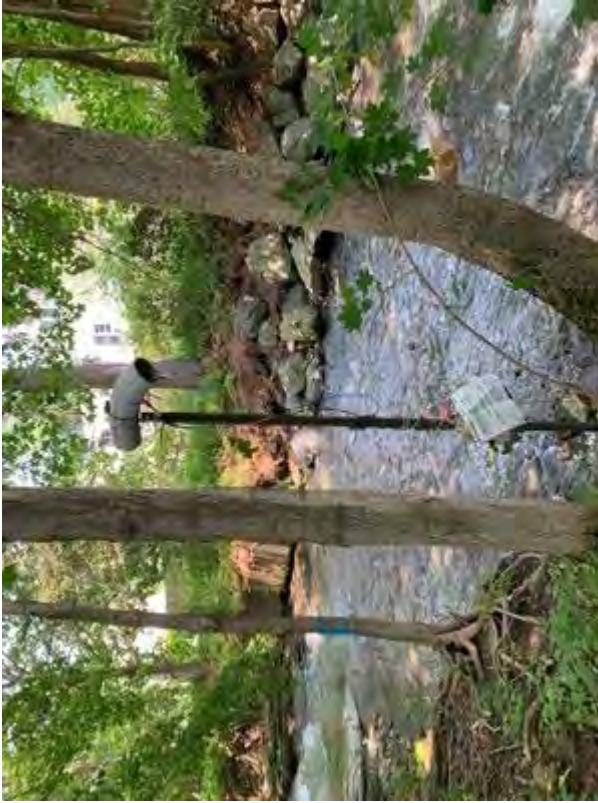
Figure D-74. Project 609072; Segment A – facing east.
