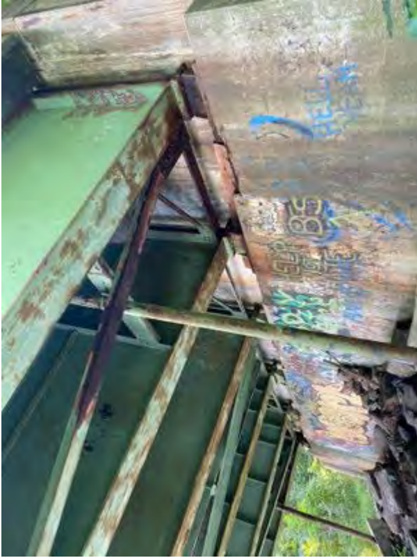
Figure D-120. Project 610857; Segment C – bridge abutment.
