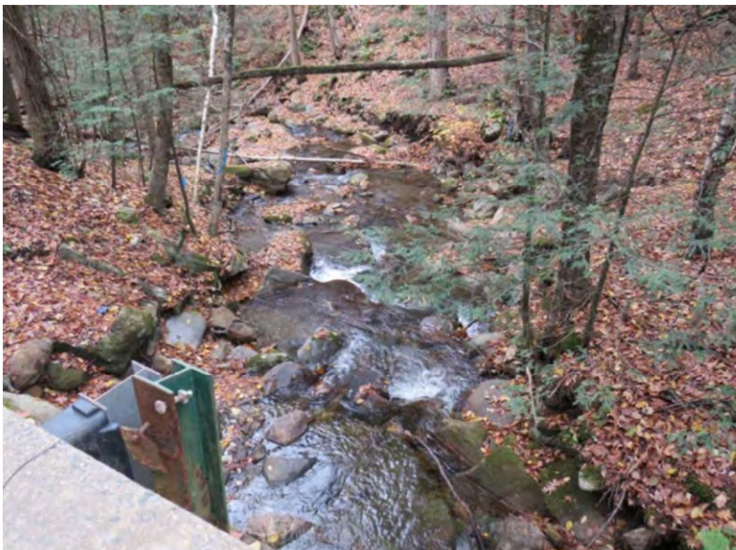
Figure B: Downstream of the Bridge
