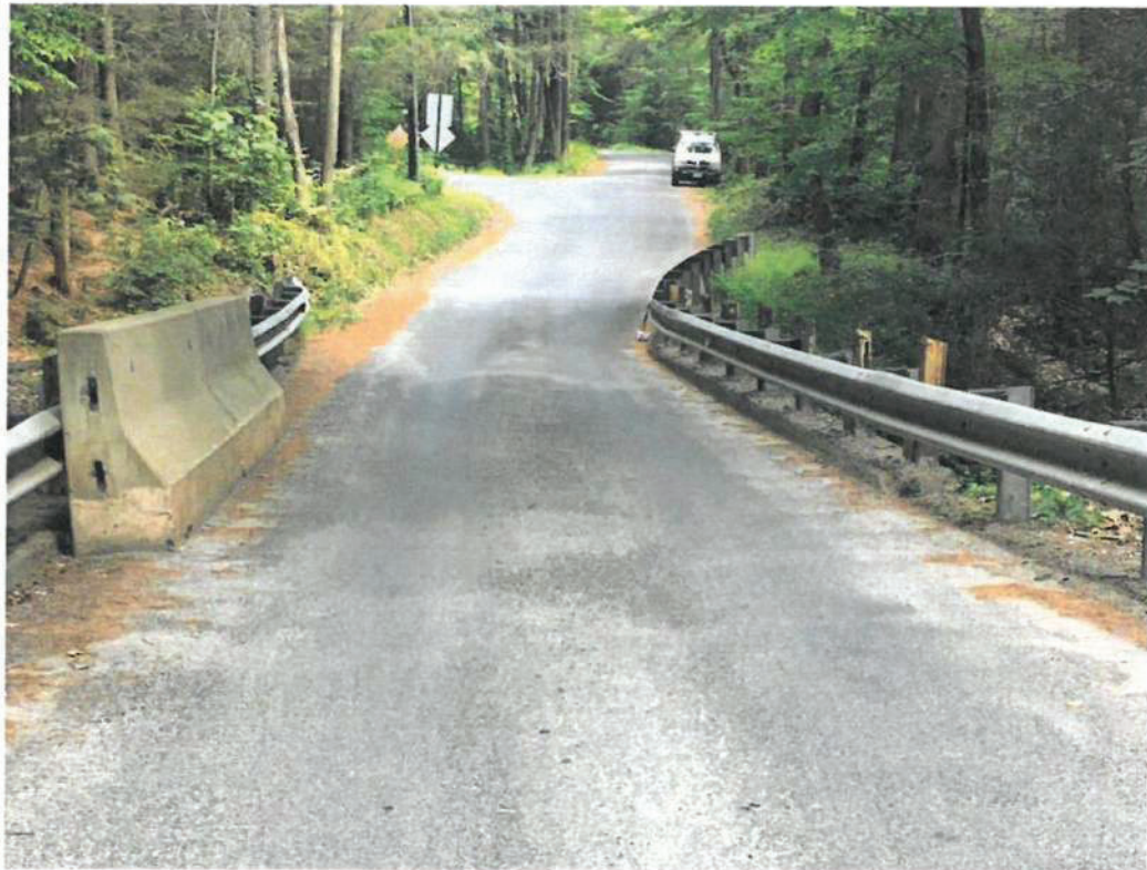
View of bridge facing north
