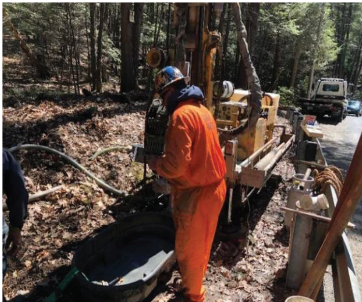
Photo 3 - View of boring BB-3 being drilled
