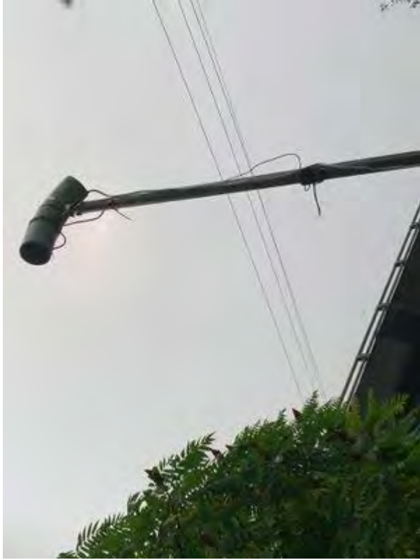
Figure D-106. Project 610857, Segment B – facing east.
