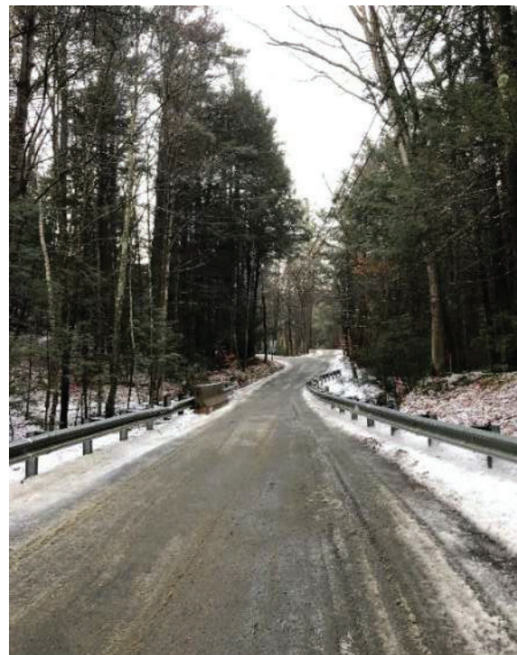
Photo 1 – View of bridge looking north
