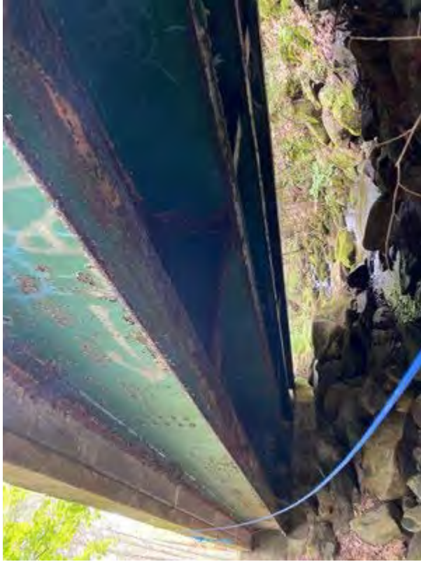
Figure D-62. Project 608858; Segment A – bridge support.
