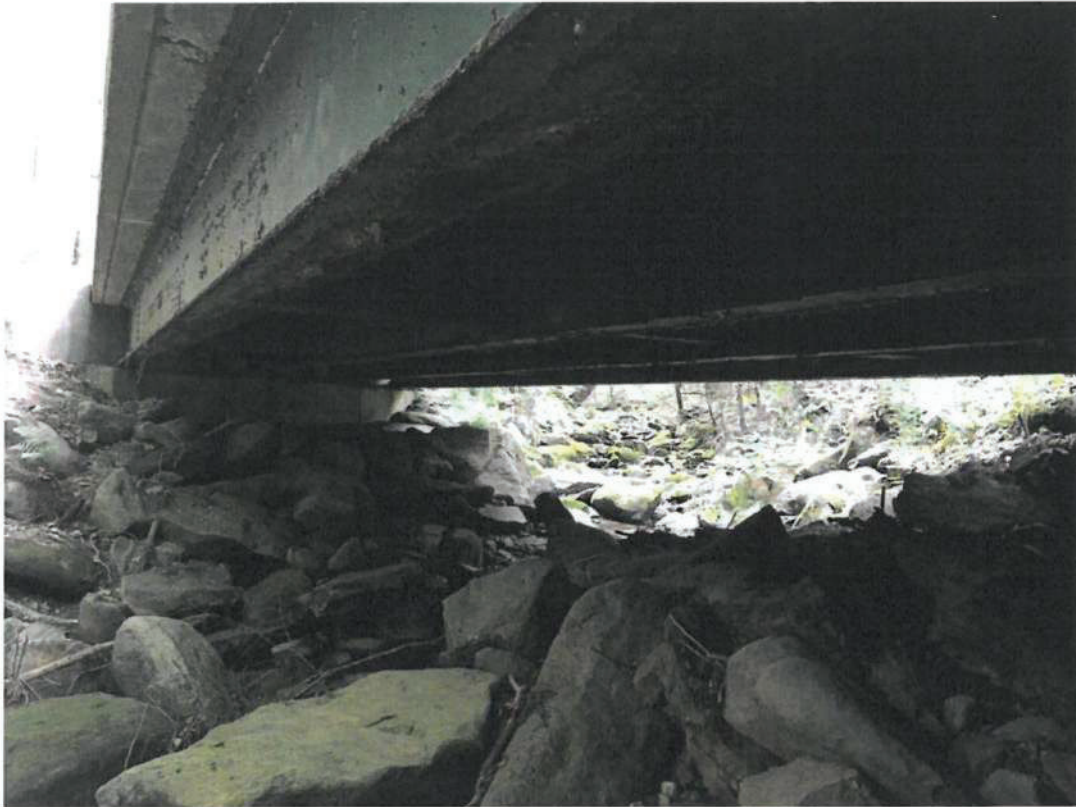
View of riprap beneath bridge
