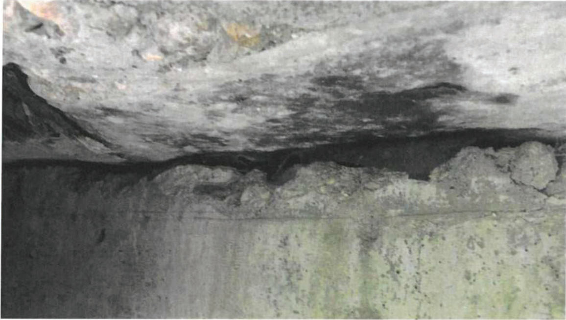
Views of black tar paper at joints along bridge deck
