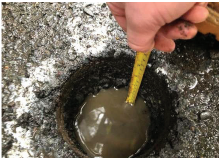
Photo 4 - View of pavement core hole
