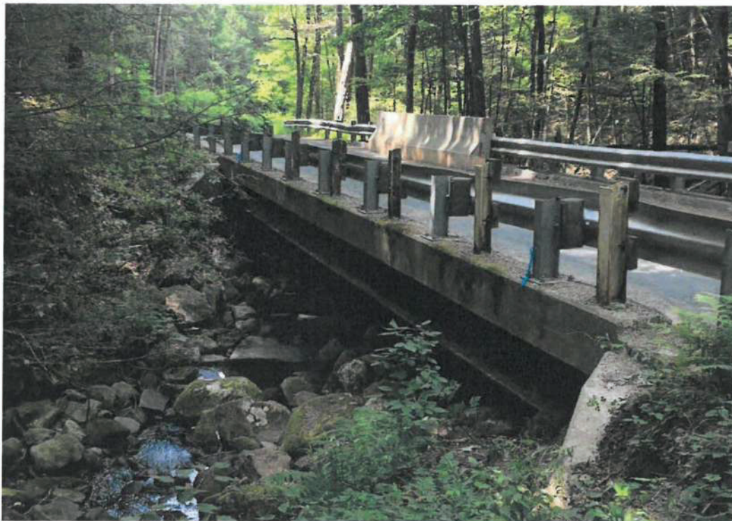
View of easterly elevation of bridge, facing southwest
