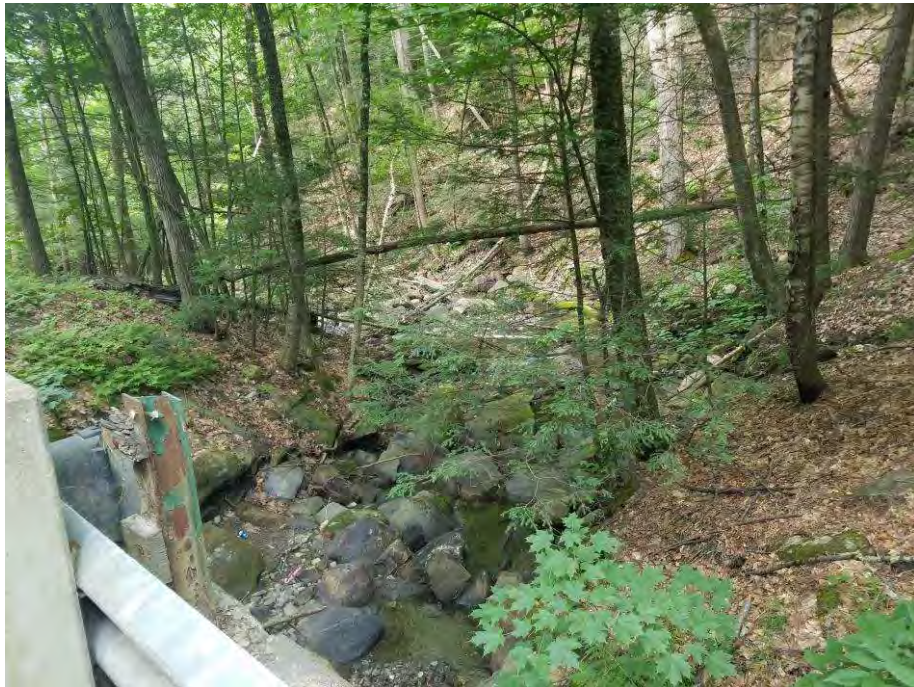
Looking west along the river from the bridge on East Oxbow Road.
