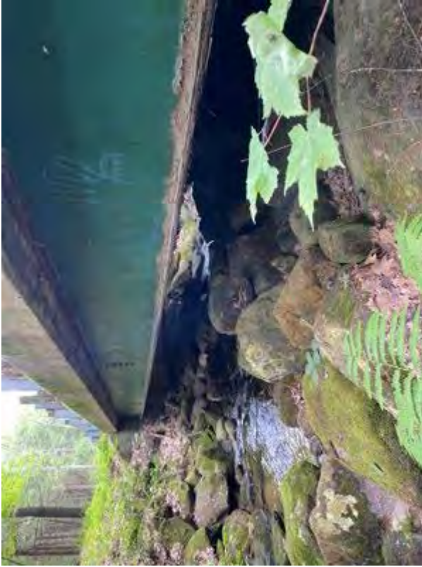
Figure D-70. Project 608858; Segment B – bridge.
