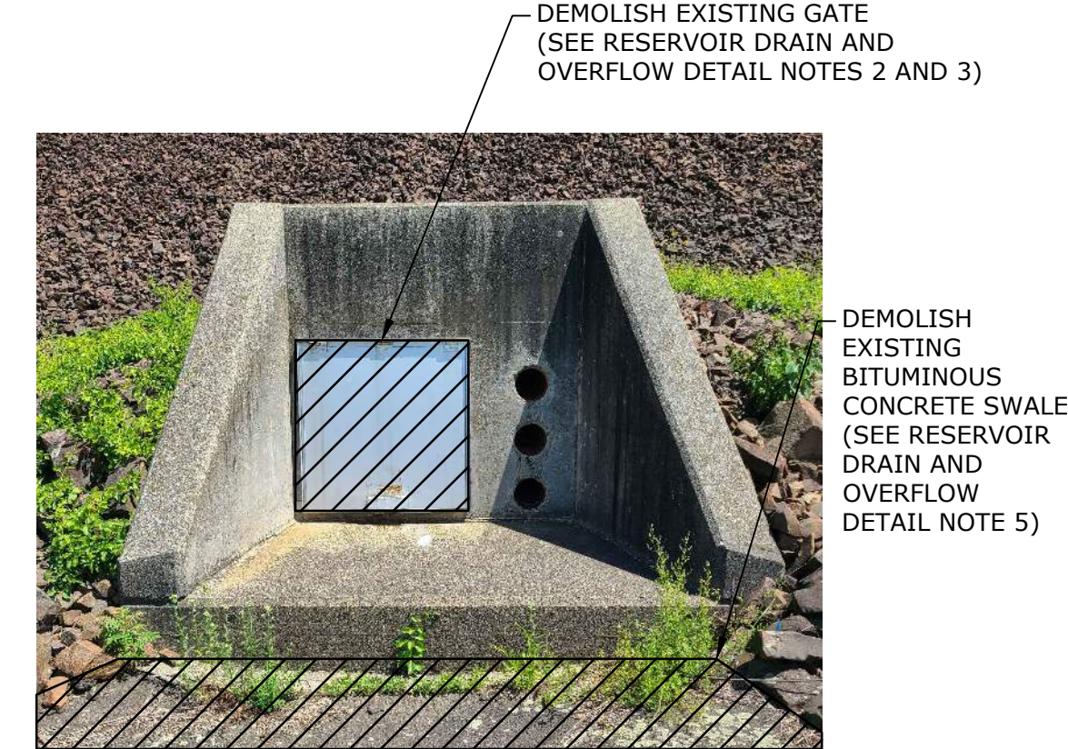
RESERVOIR NO. 4 EXISTING CONCRETE HEADWALL PHOTO
