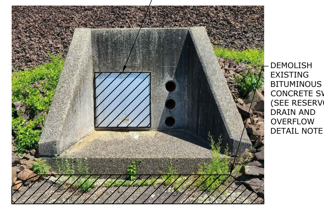
RESERVOIR NO. 4 EXISTING CONCRETE HEADWALL PHOTO
