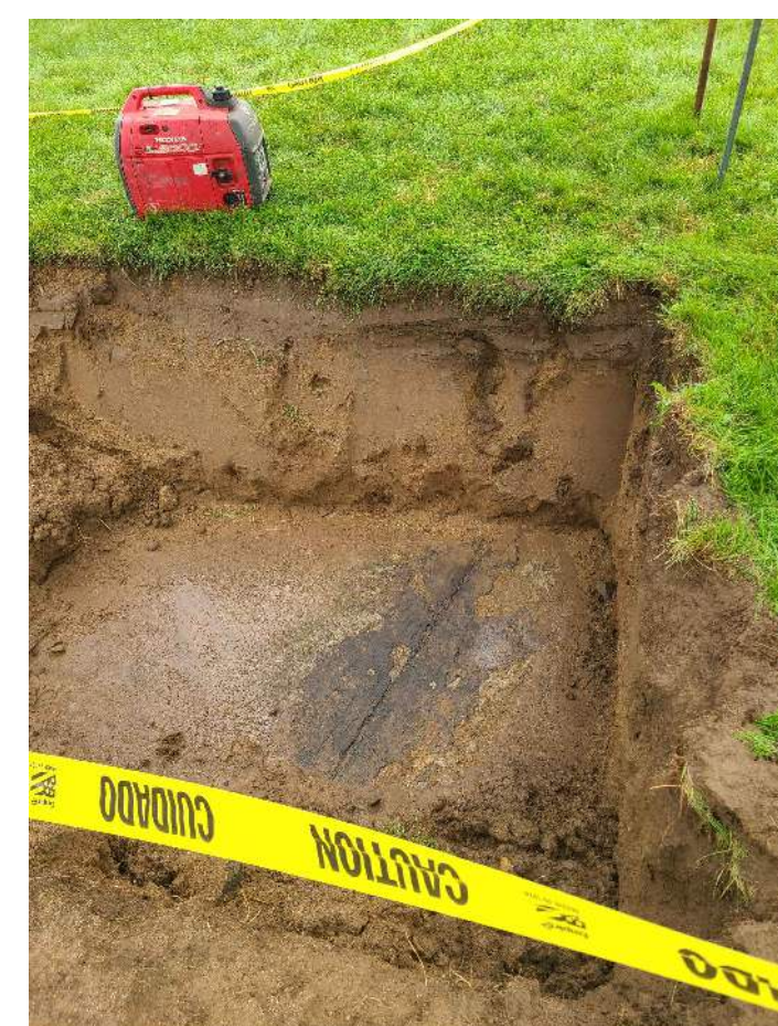
TEST PIT OF EXPANSION JOINT PERFORMED BY TIGHE & BOND PHOTO
