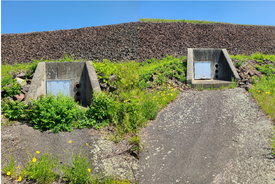
Overflowheadwalls to reservoir 4 and 3
