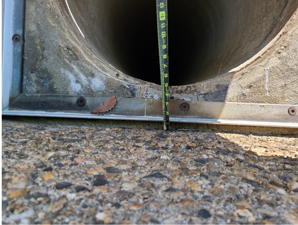
Overflowheadwall to reservoir 3
