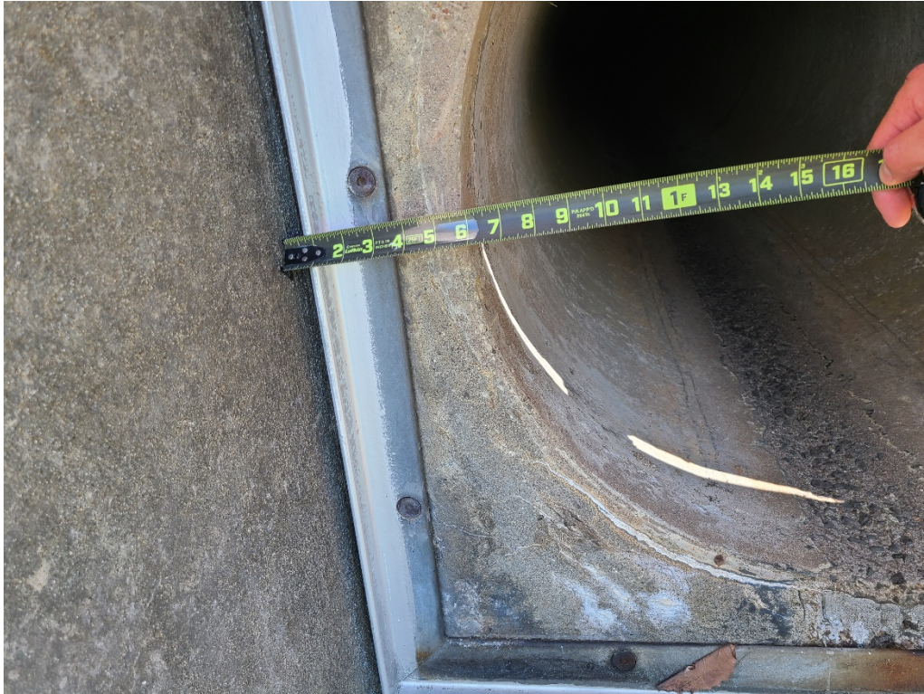
Overflowheadwall to reservoir 3
