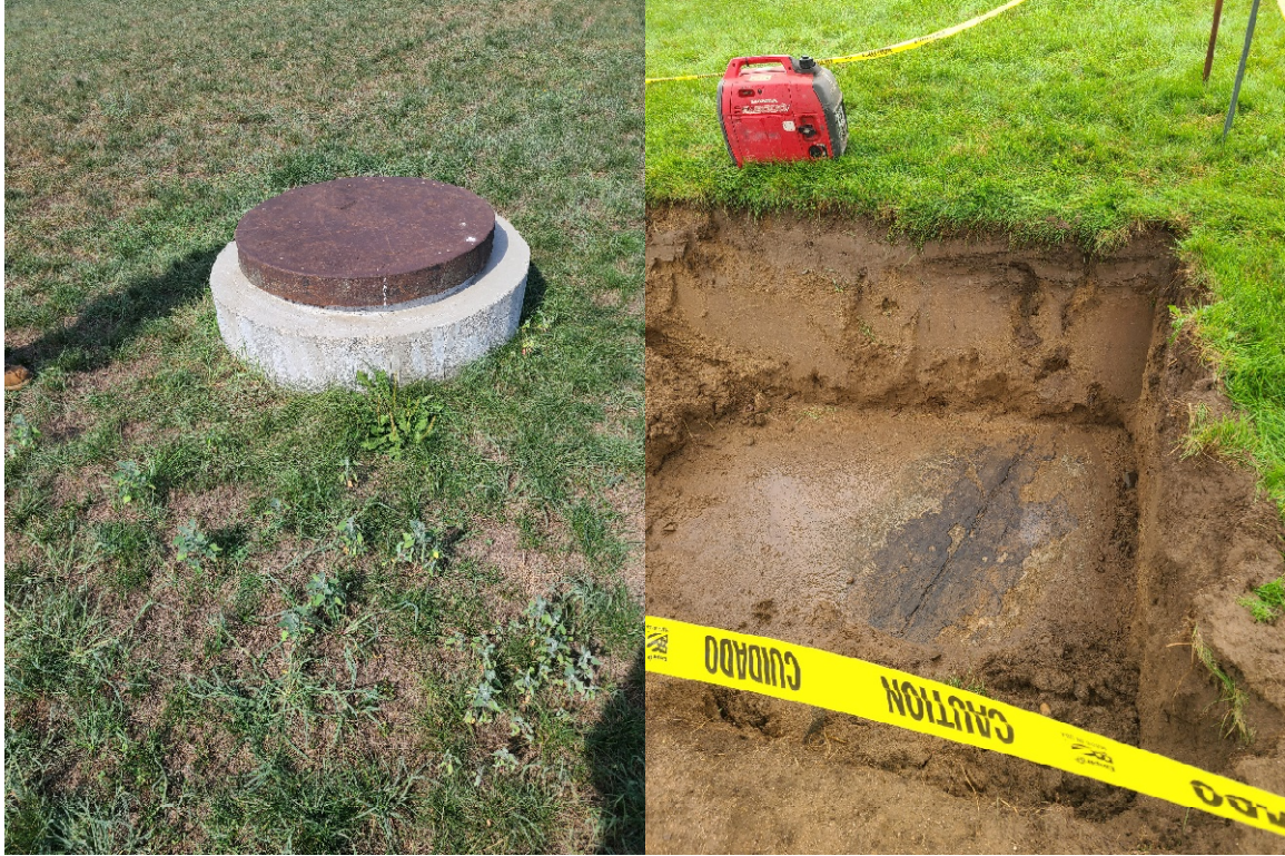
Access manhole on reservoir and existing reservoir expansion joint
