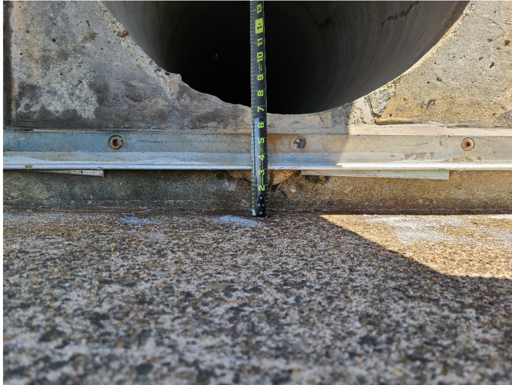
Overflowheadwall to reservoir 4
