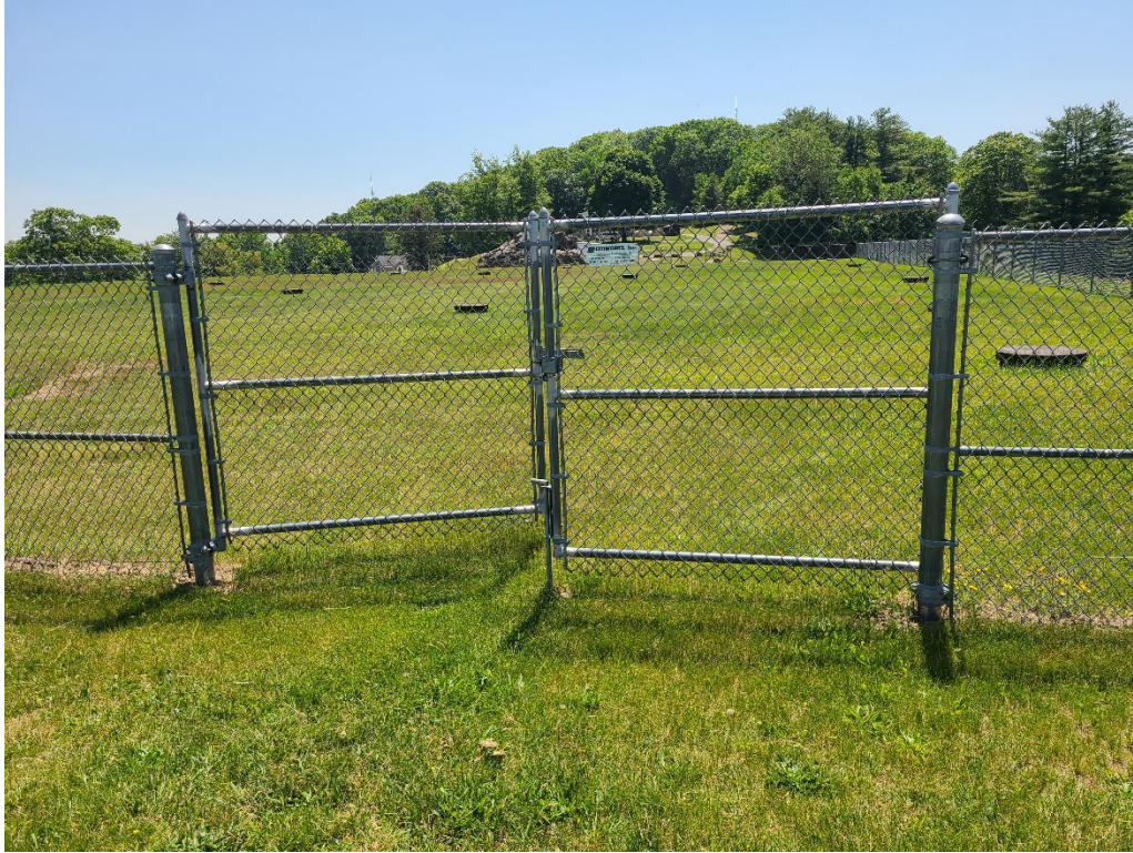
Chain link fence on reservoir 2
