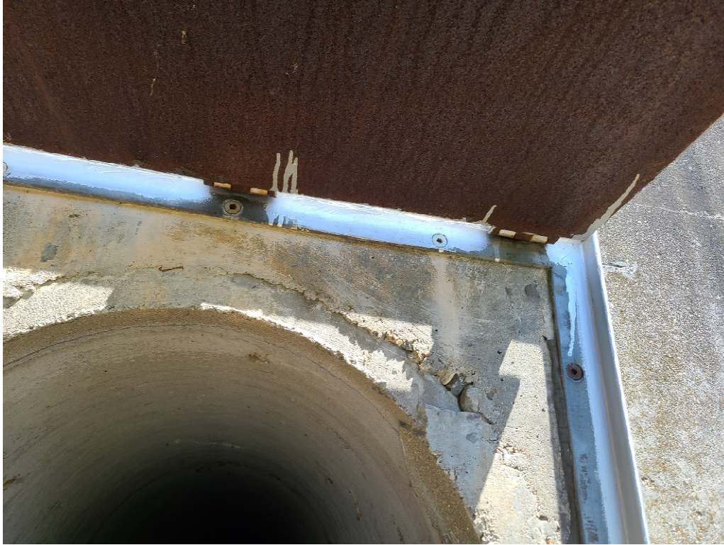
Overflowheadwall to reservoir 4
