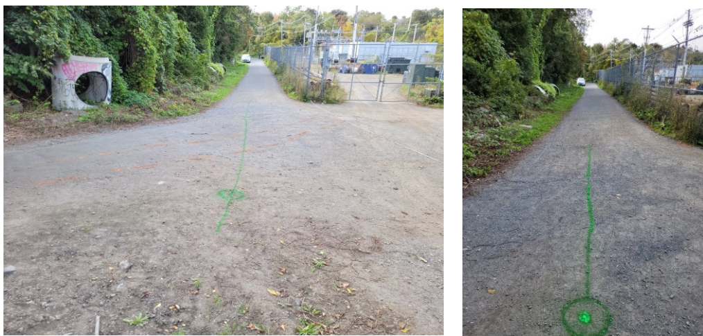
Figure 6: Photograph of Field markings- green sewer/orange electric duct (facing south)
