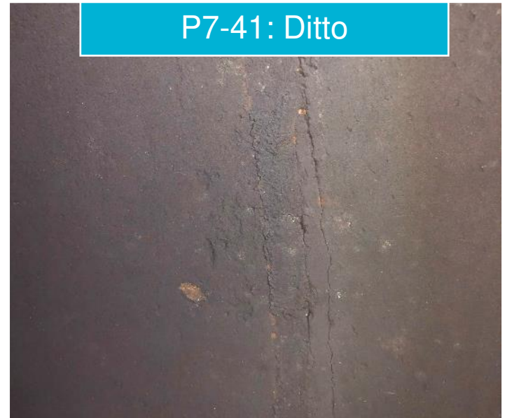
P7-41: Circumferential Cracks 10:30-12:00; 4:30-5:30; 2:00-3:00
