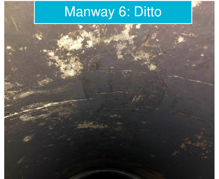
Manway 6: Boiler-Type, Corroded. No major cracks but faint mortar crack around opening. Couple of circumferential hairline cracks near manhole opening, autogenous healing visible.
