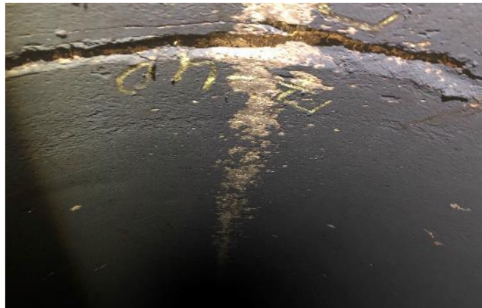
P7-41: Circumferential Cracks 10:30-12:00; 4:30-5:30; 2:00-3:00
