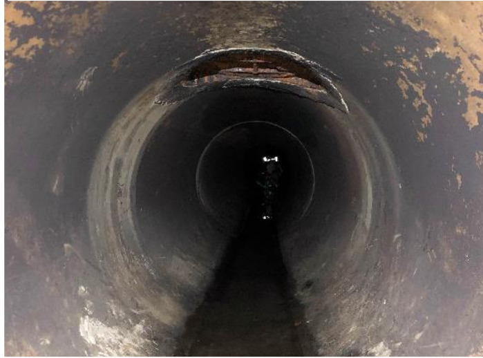
Manway 5: Boiler-Type, Corroded, No Cracks
