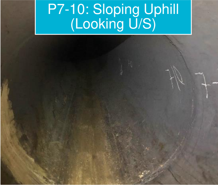
Black Streak Along 6:00 at Steep Section
