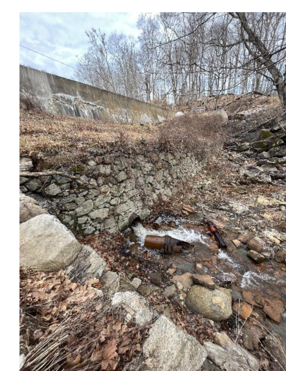
PHOTO 3 LOW-LEVEL OUTLET PIPE
