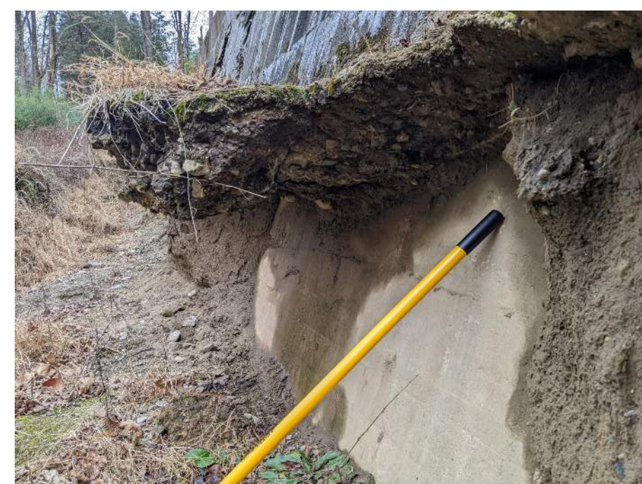
PHOTO 1 EROSION AT CONC. DAM DOWNSTREAM FACE
