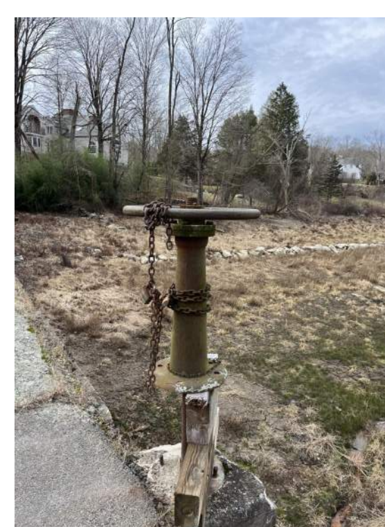
PHOTO 2 LOW-LEVEL OUTLET GATE OPERATOR
