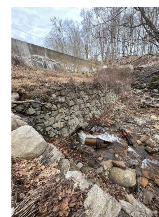
PHOTO 3 LOW-LEVEL OUTLET PIPE
