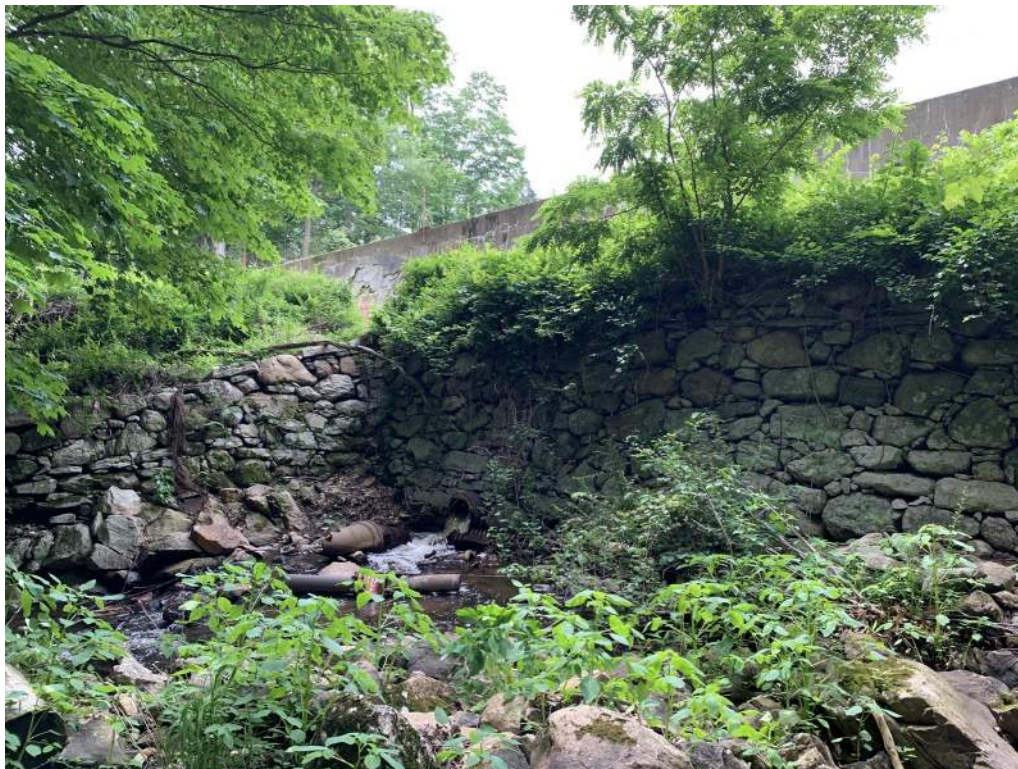
Photograph 16 – Low-level outlet from downstream.
