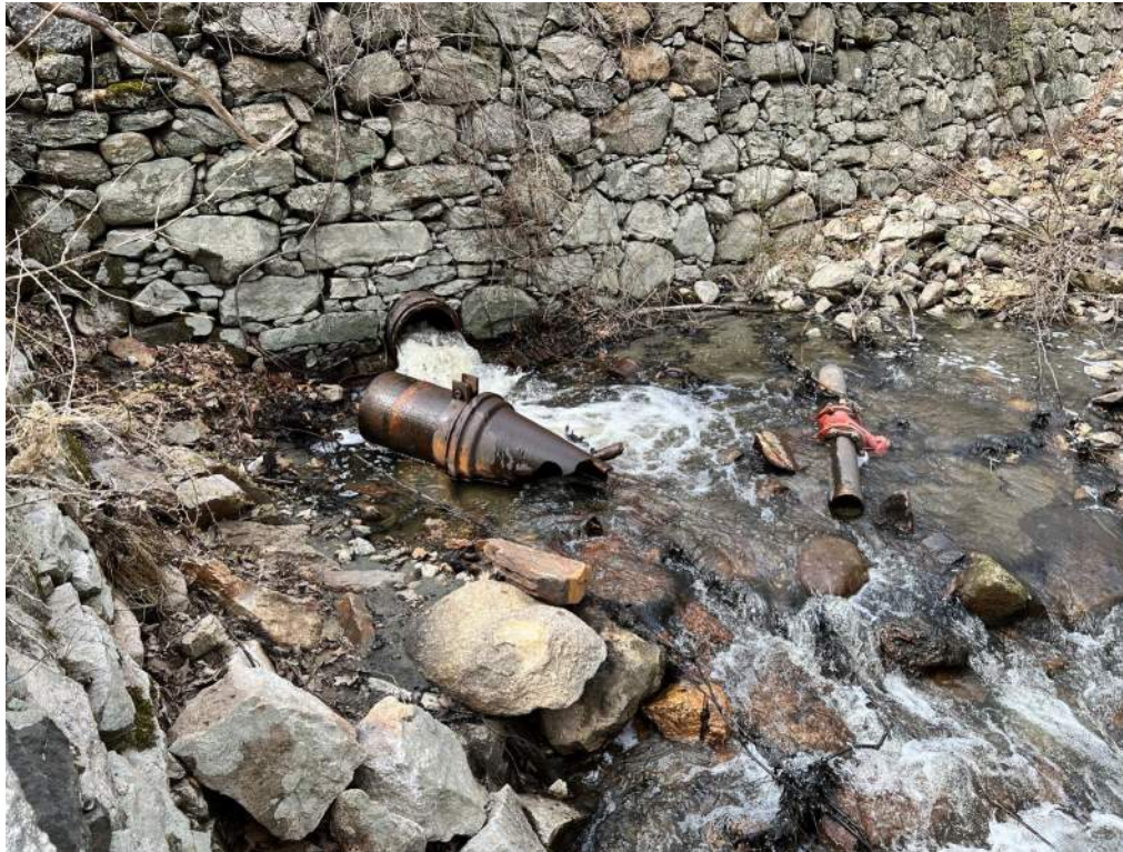
Photograph 16 – Low-level outlet from downstream.
