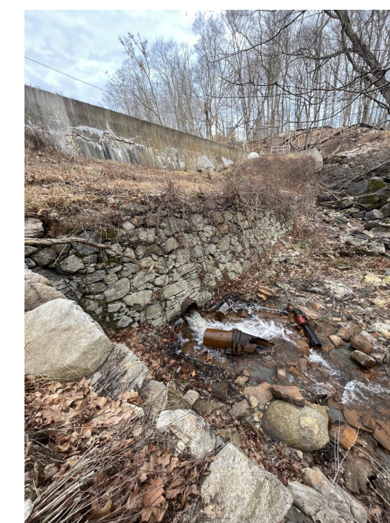
PHOTO 3 LOW-LEVEL OUTLET PIPE
