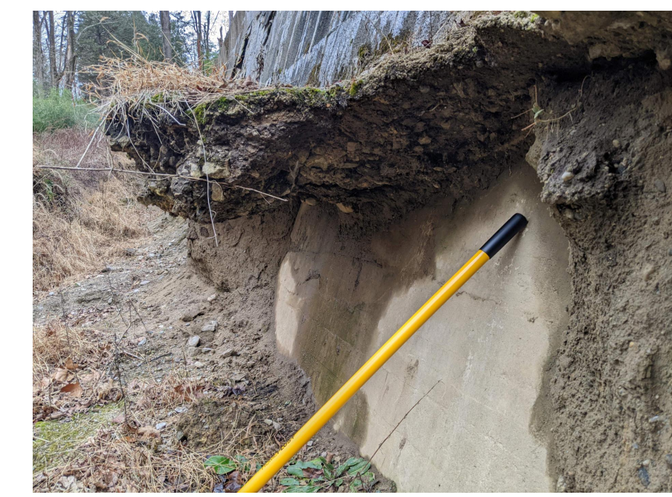
PHOTO 1 EROSION AT CONC. DAM DOWNSTREAM FACE
