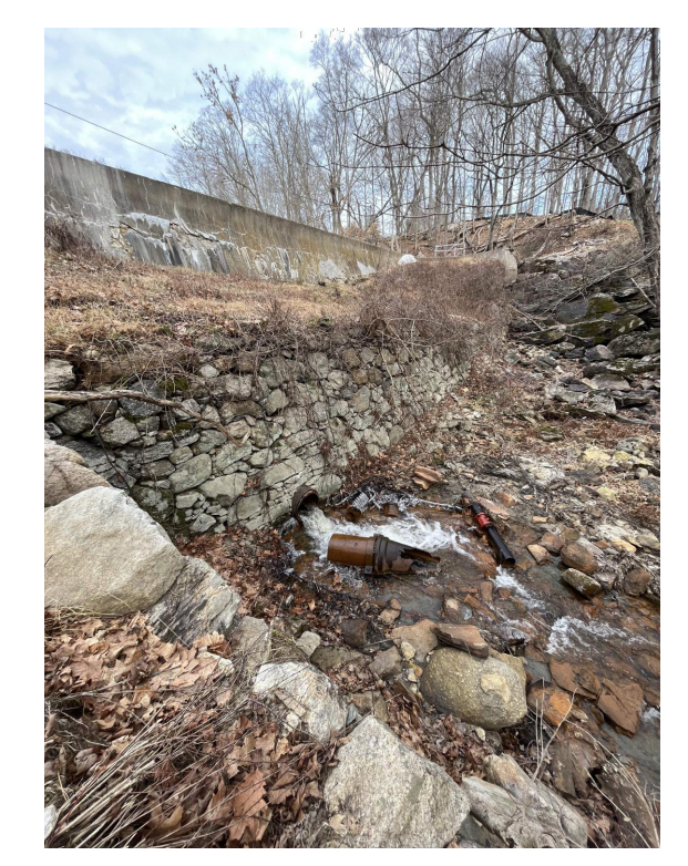
PHOTO 3 LOW-LEVEL OUTLET PIPE
