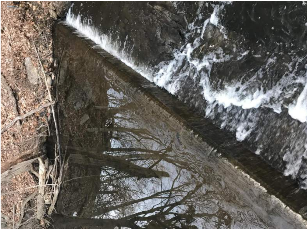
Photograph 12 – Primary spillway weir (flowing) from dam crest.
