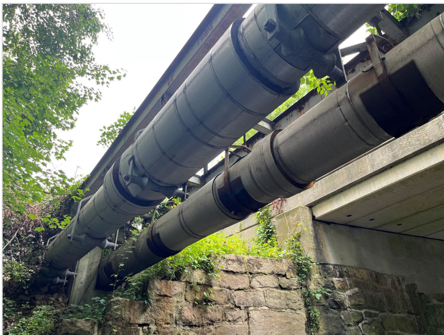
Photograph 5 – Underside looking South.
