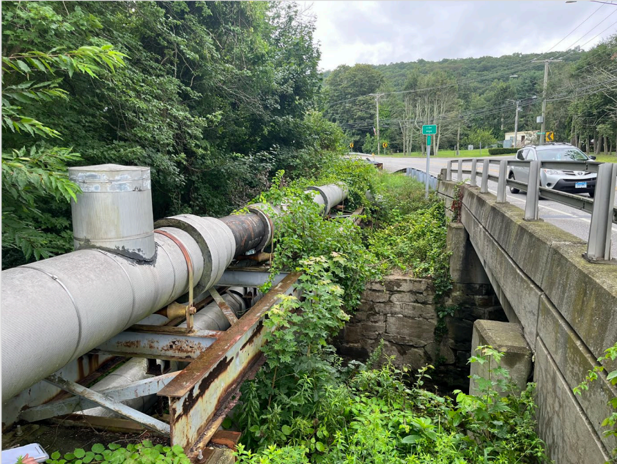
Photograph 1 – West side looking South.
