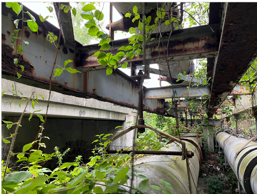
Photograph 9 – Underside looking North
