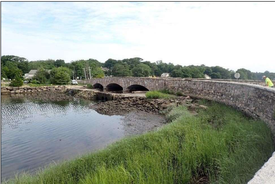
Photo 8: Wetland Area at Left Abutment
