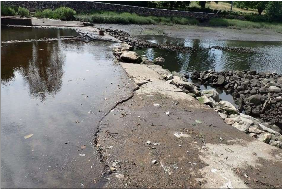
Photo 2: Spillway Crest from Right Abutment
