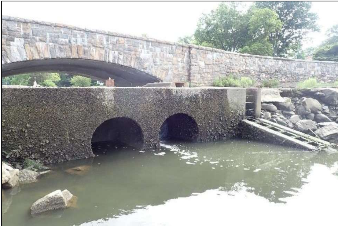
Photo 9: Downstream face of tide gates
