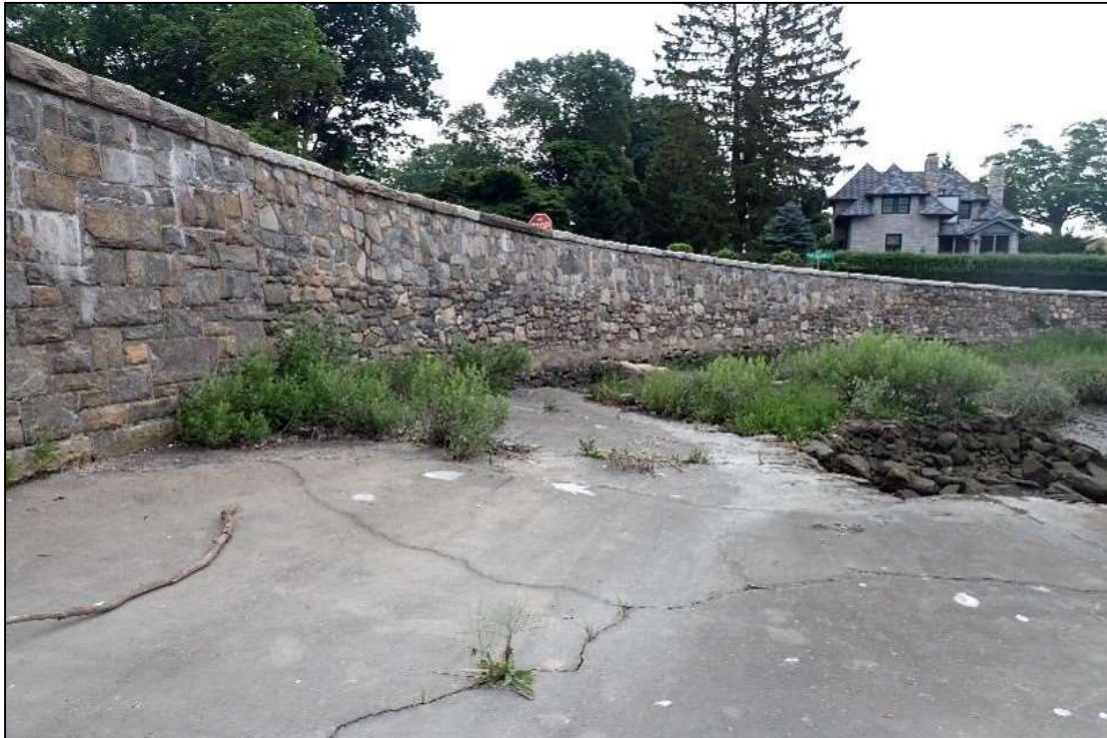
Photo 3: Downstream View of Left Abutment
