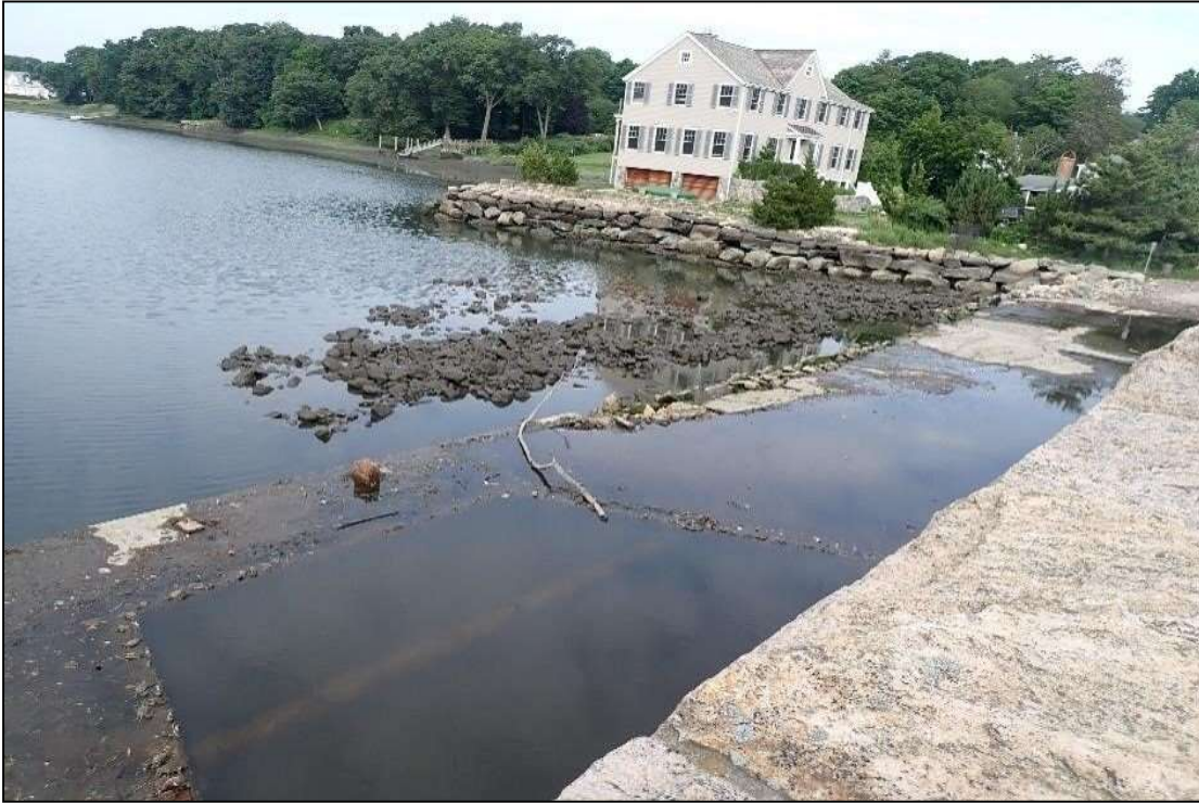
Photo 1: Spillway Crest from Left Side of Rings End Road Bridge
