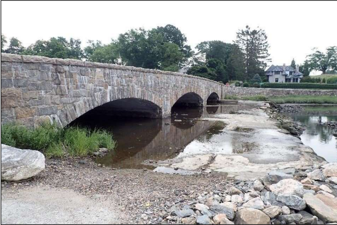
Photo 7: Downstream Overview of Bridge from Right Abutment
