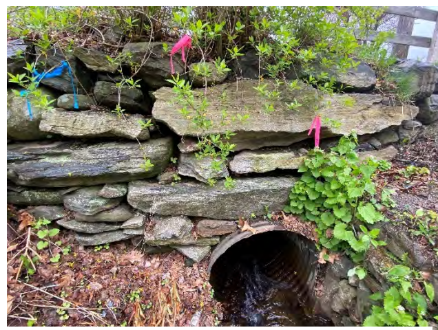
Photo 2: Upstream of Park Street Culvert Crossing
