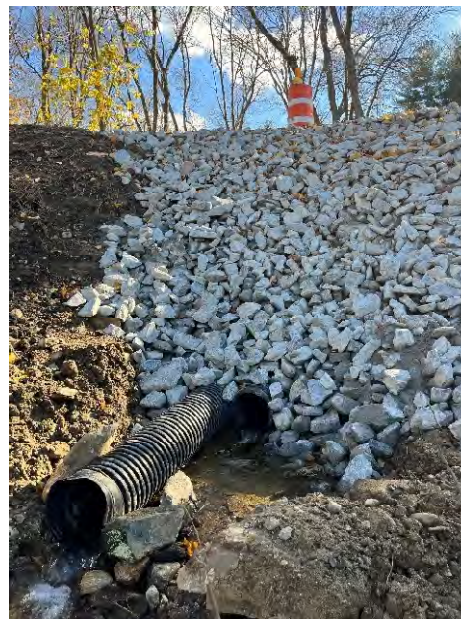
Photo 1: Downstream of Brigham Culvert Crossing
