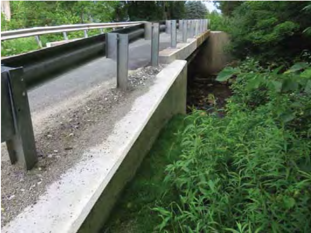
Photo 8: Repair of the southeast wingwall and rail base.
