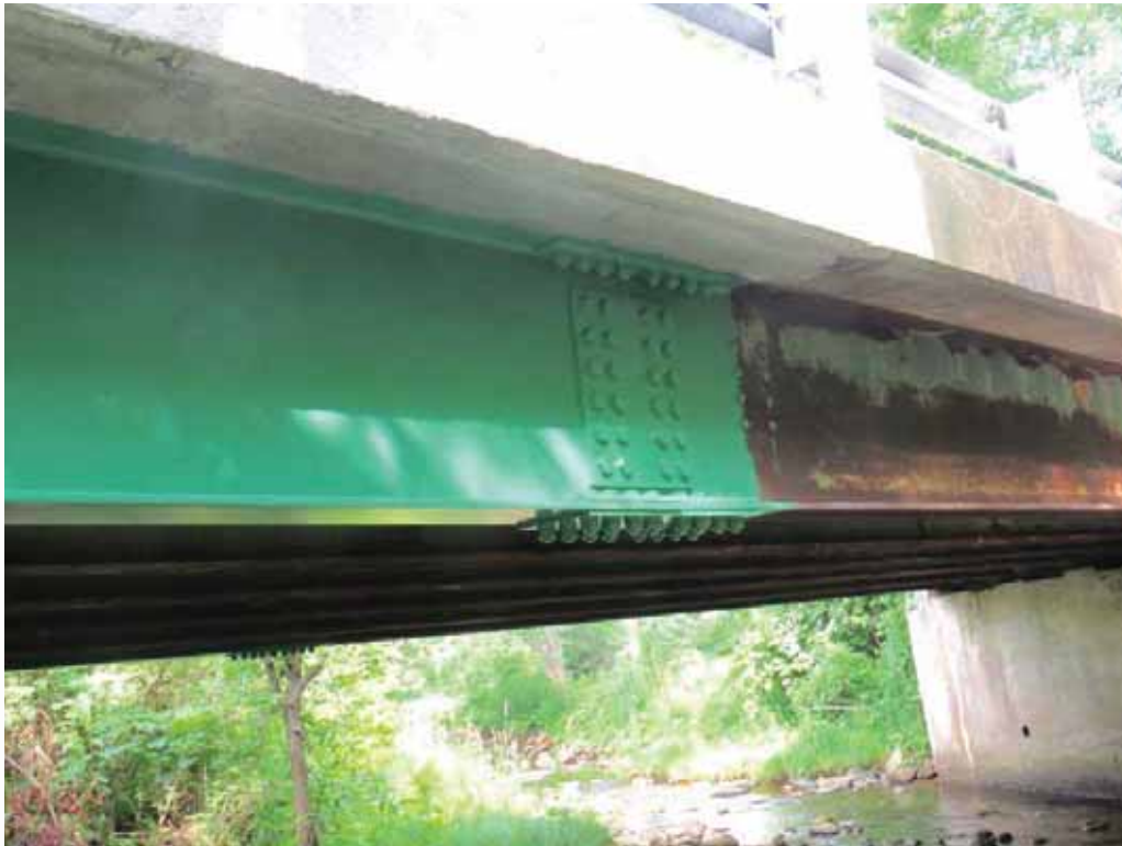
Photo 3: Beam 1, east elevation, new beam section and splice plates.
