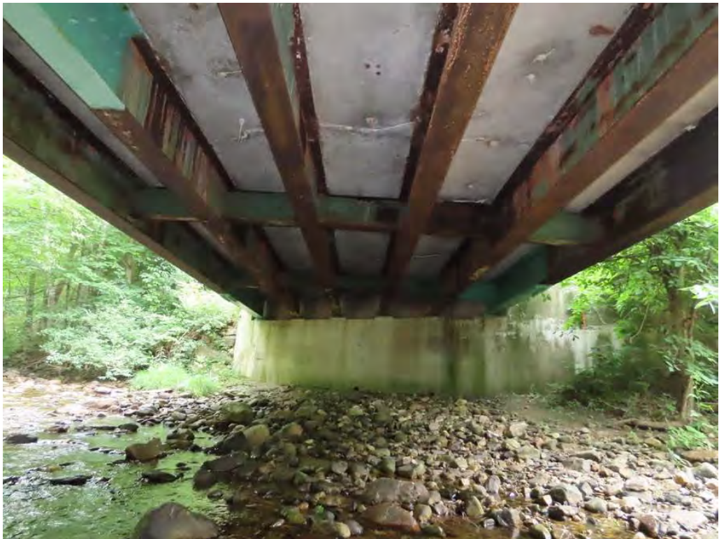
Photo 2: General underside view, looking south.
