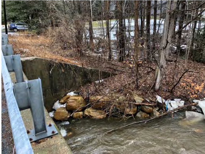
Photo 3 – View of the northeast wingwall and rip-rap riverbank protection.
