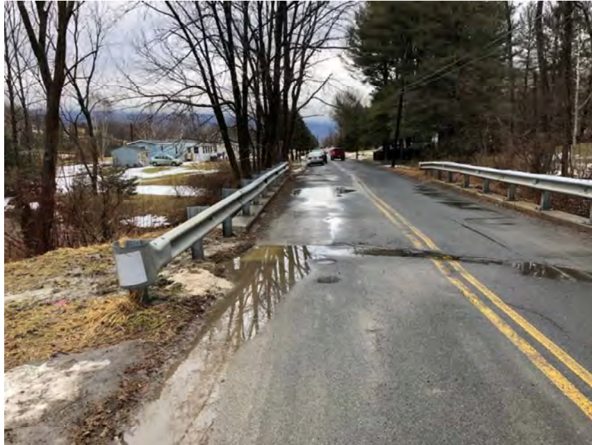
Photo 1 – View of bridge looking north from behind the south abutment.
