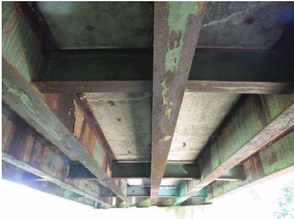
Photo 2: General underside view, looking north.
