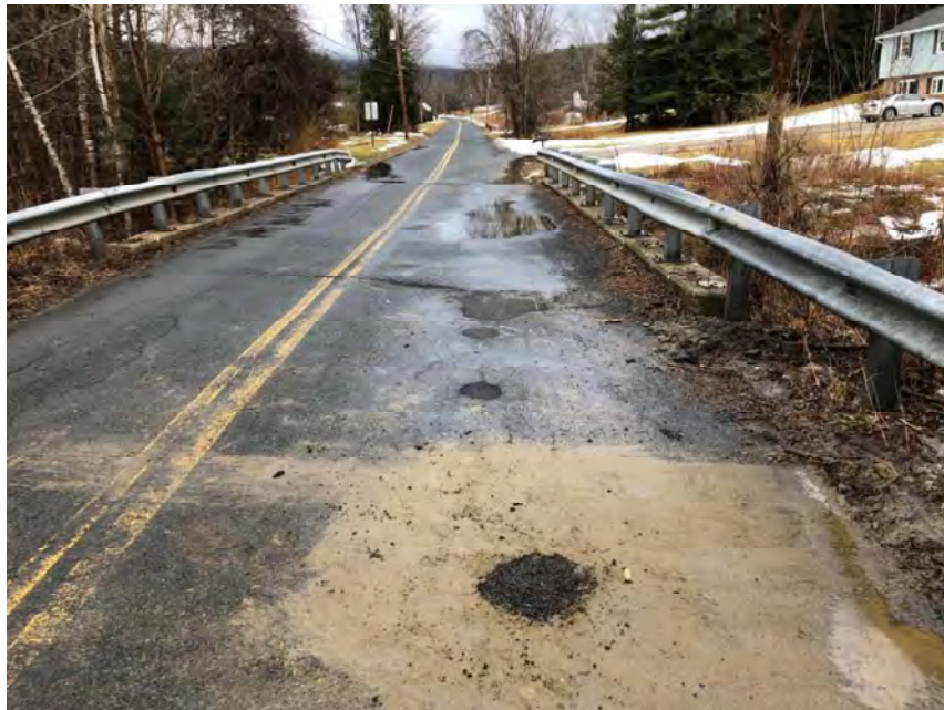
Photo 2 – View of bridge looking south from behind the north abutment.
