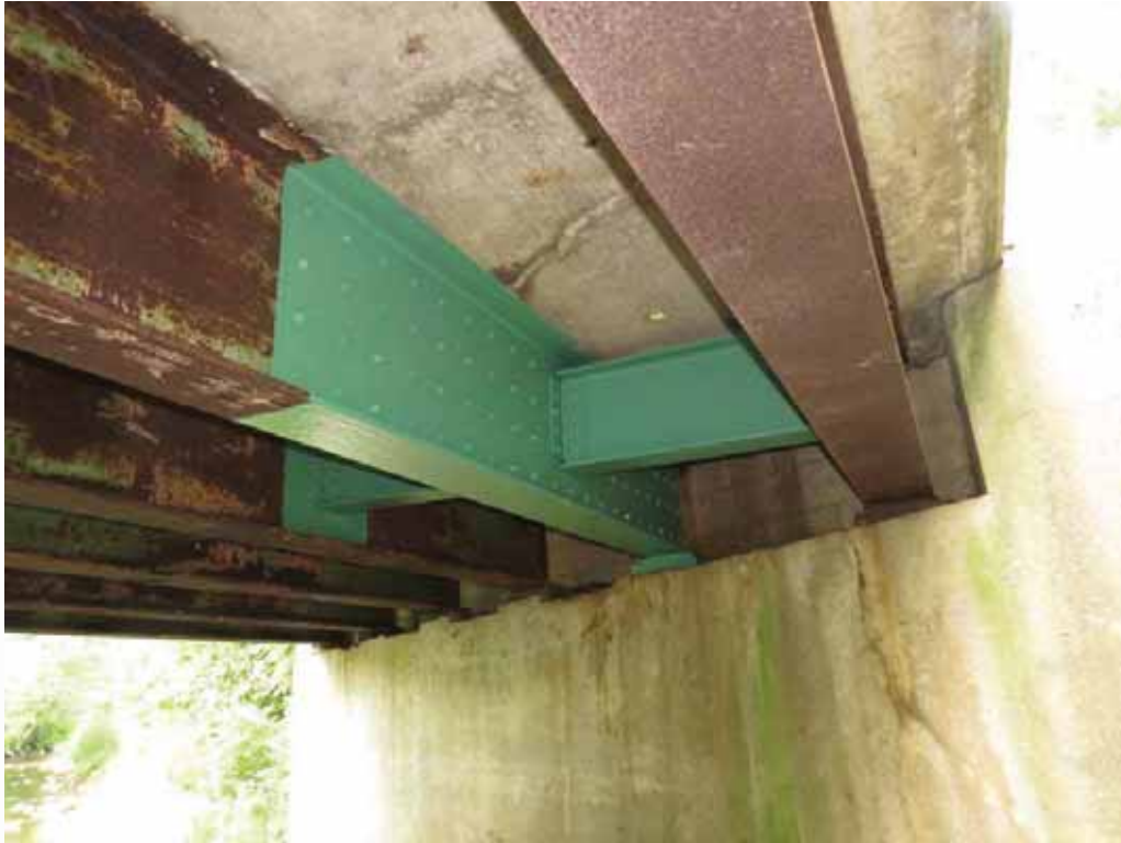
Photo 5: Beam 2, north end, web repair plating and new intermediate diaphragms.
