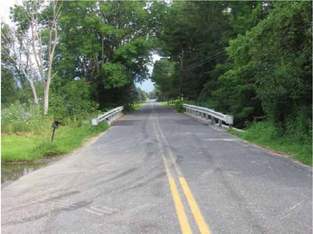
Photo 1: General topside looking north.
