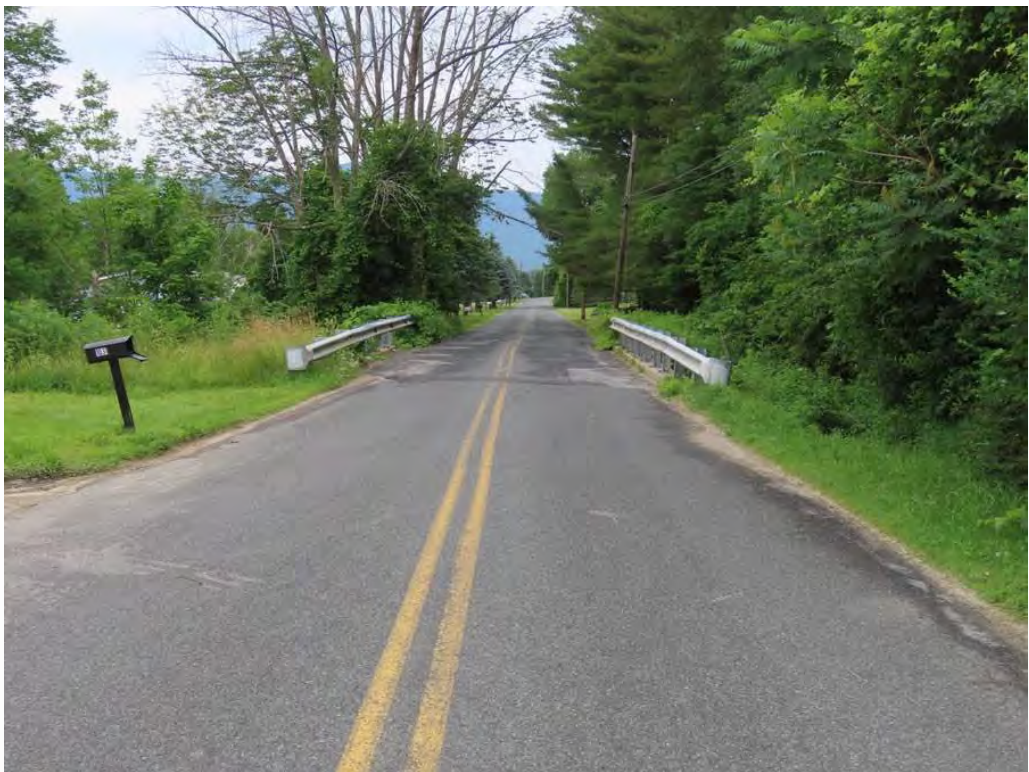
Photo 1: General topside view, looking north.
