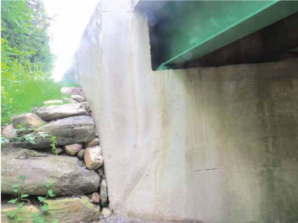
Photo 7: Repair of the southeast abutment corner and wingwall.
