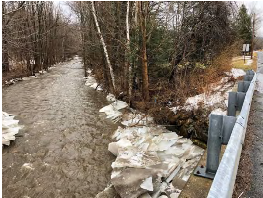
Photo 4 – View of the southeast wingwall and rip-rap riverbank protection.
