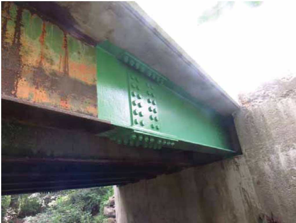
Photo 4: Beam 6, west elevation, new beam section and splice plates.
