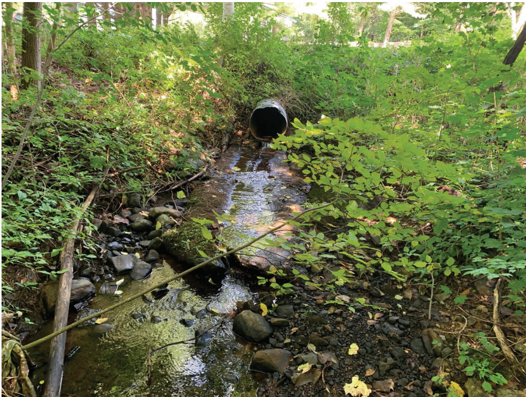
Photo 2: Culvert where intermittent stream originates from.
