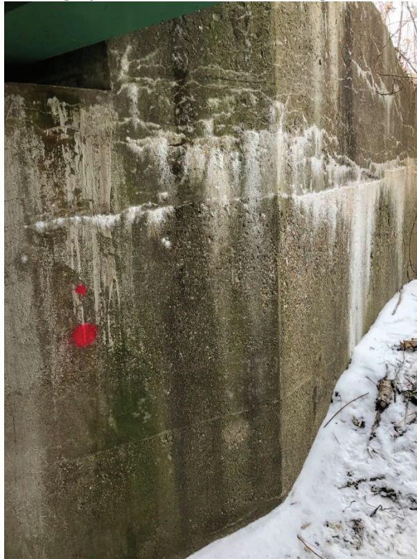
Photograph 4: Abutment deterioration
