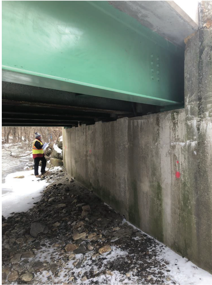
Photograph 5: Abutment Deterioration
