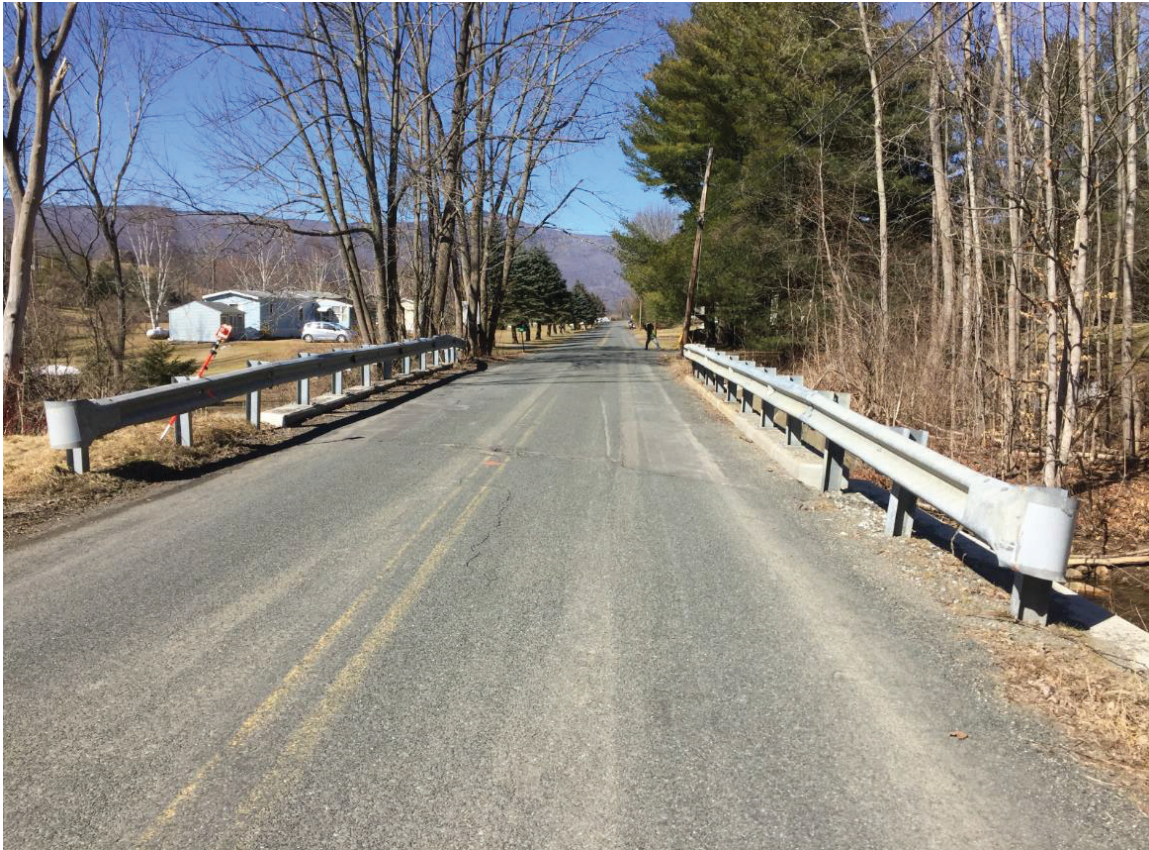
Photograph #3: Sand Mill Road facing northeast
