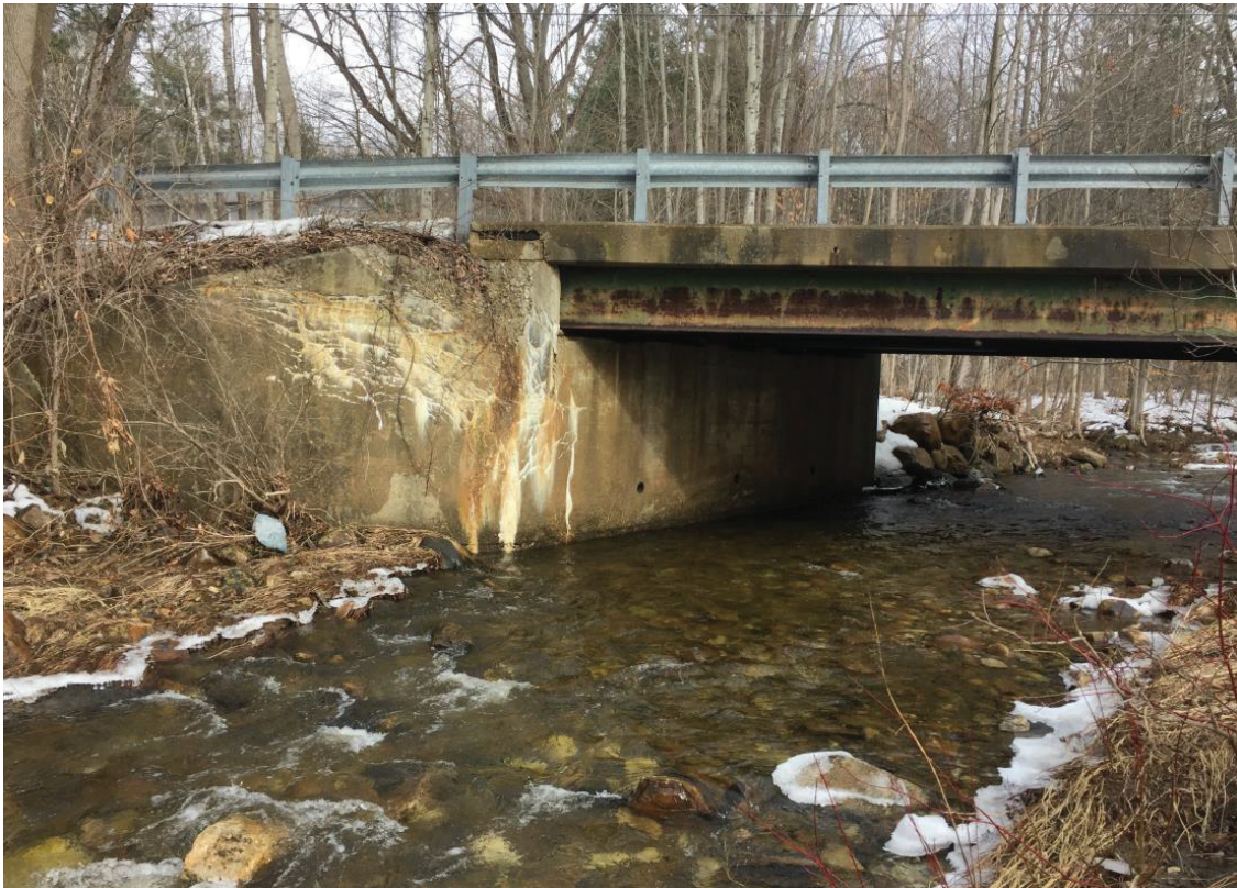
Photograph #2: Sand Mill Road Bridge from northwest
