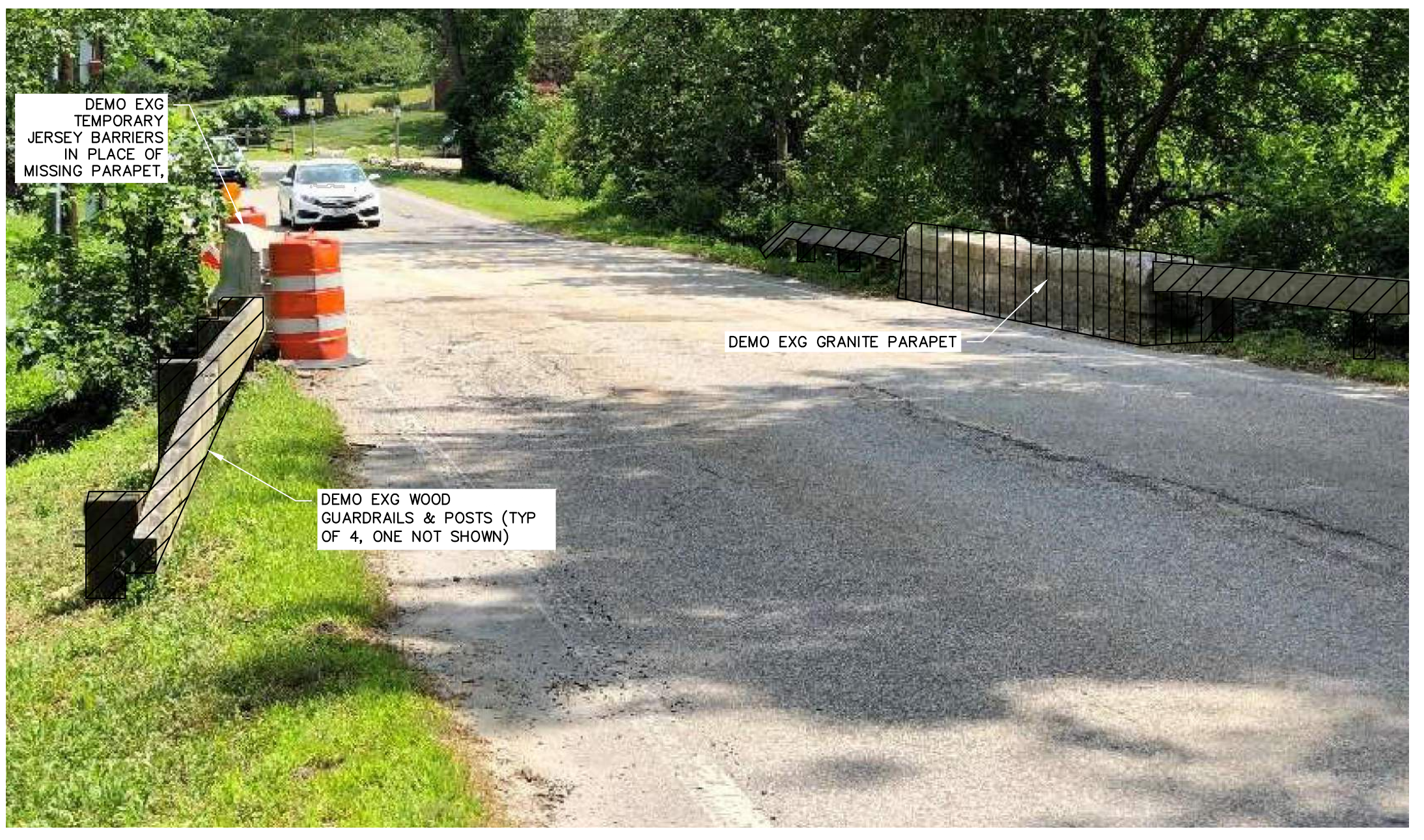
PHOTO 1: EXISTING CONDITIONS - WAYSIDE BRIDGE LOOKING SOUTH
