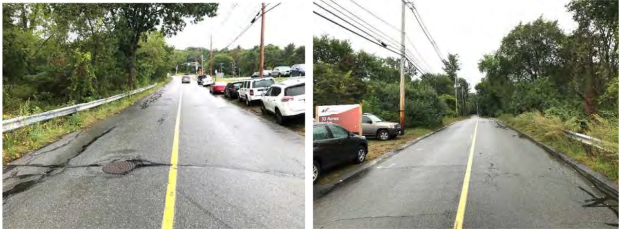
LEFT- Looking west from STA 29+00 the overflow commuter parking on the north side of Foster St is visible. RIGHT- Looking east from STA 29+00 the overflow commuter parking on the north side of Foster St is visible.
