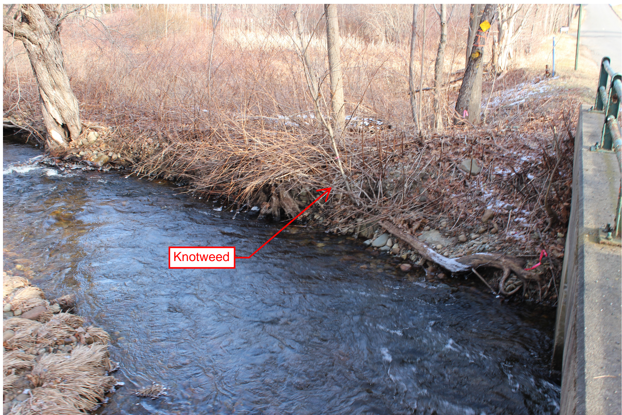
View of the northeast embankment downstream of the bridge, looking Northeast.
