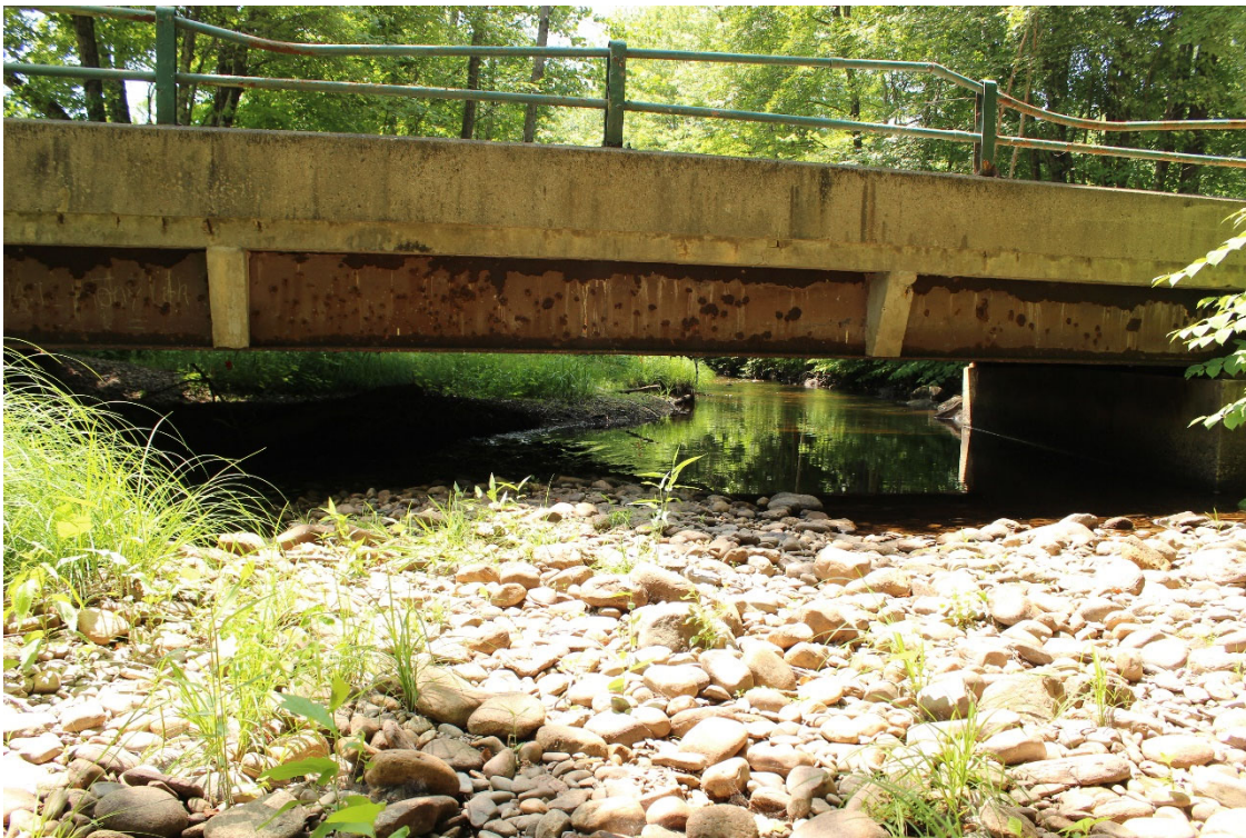
Photo 2: Downstream Face of South St. Bridge over Sawmill River
