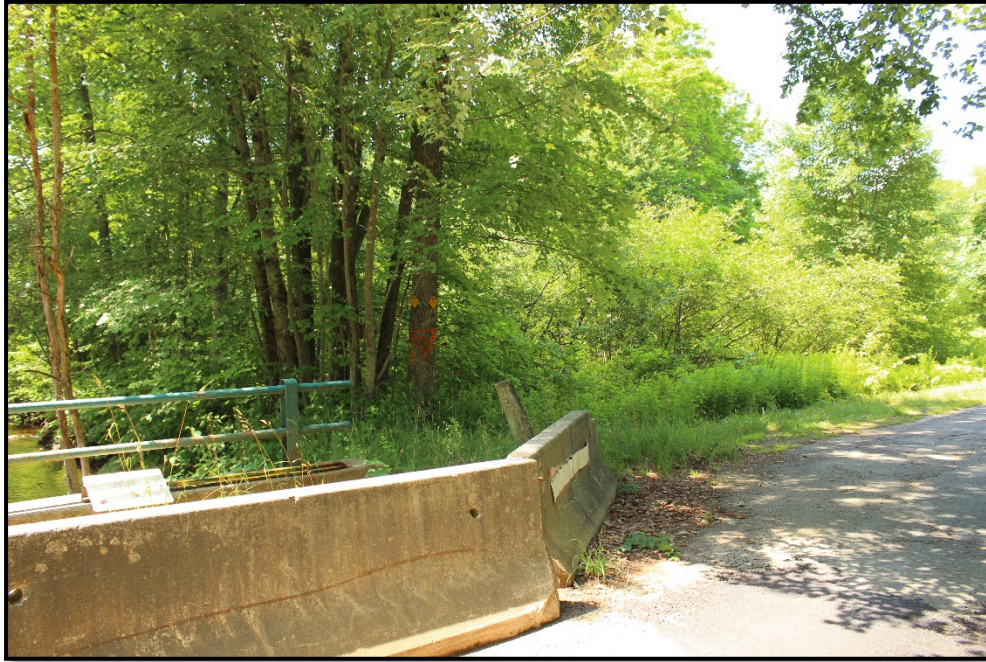
Photo 11: View of wildlife management area Southwest of the bridge, looking Southwest.
