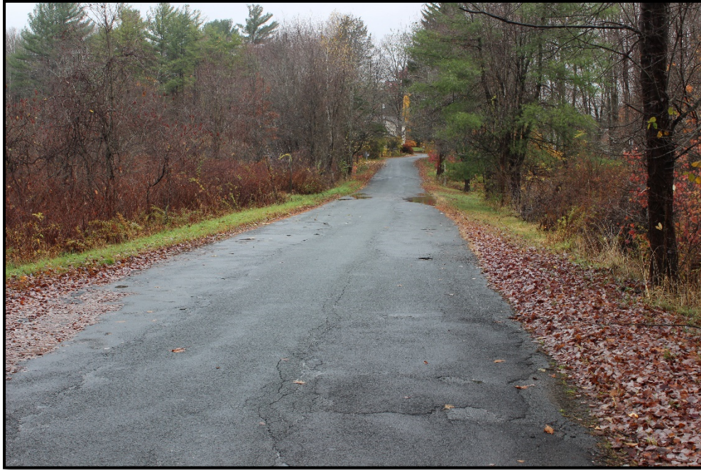
Photo 3: View of the West Approach, looking West.
