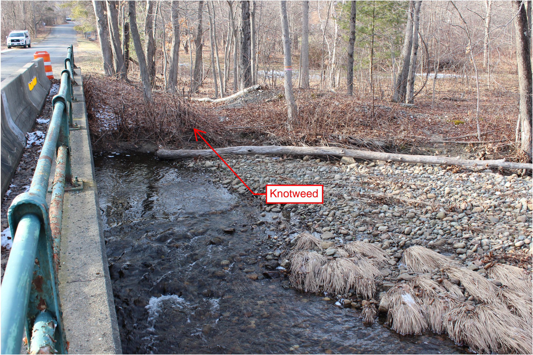
View of the northwest embankment downstream of the bridge, looking Northwest.
