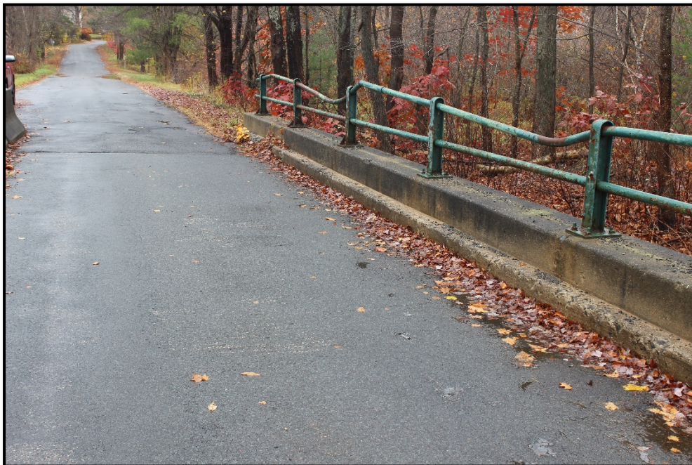
Photo 2: View of the top of bridge, looking West.
