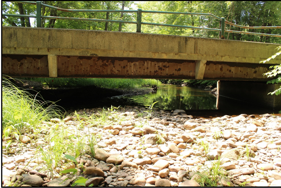
Photo 1: View of the North elevation of bridge, looking South.
