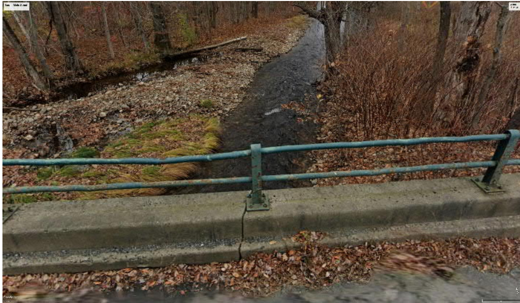
Figure 2-3: Sawmill River Downstream of the Bridge
