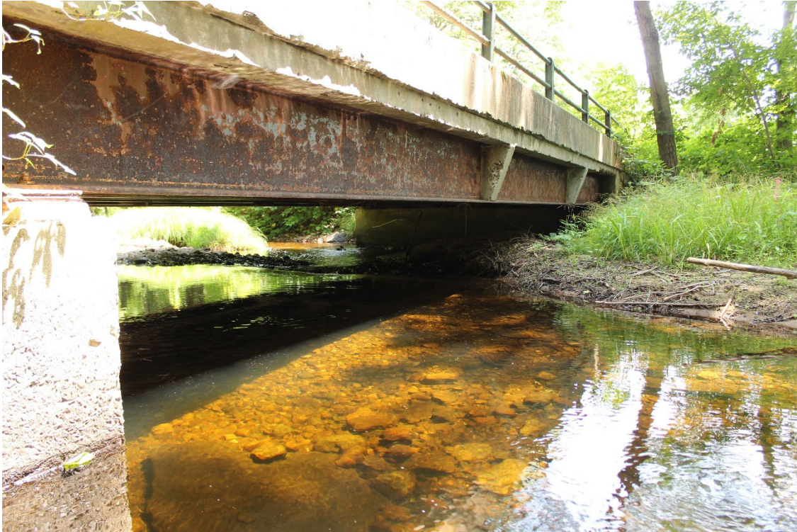
Photo 1: Upstream Face of South St. Bridge over Sawmill River
