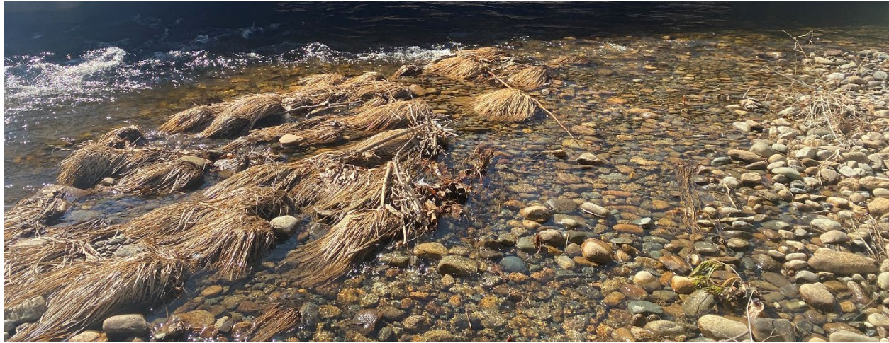
Figure A: Existing Streambed Material Near the Bridge
