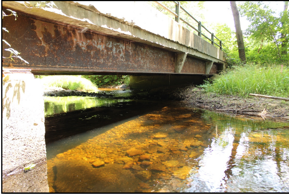
Photo 7: View of the South elevation of the bridge, looking Northeast.
