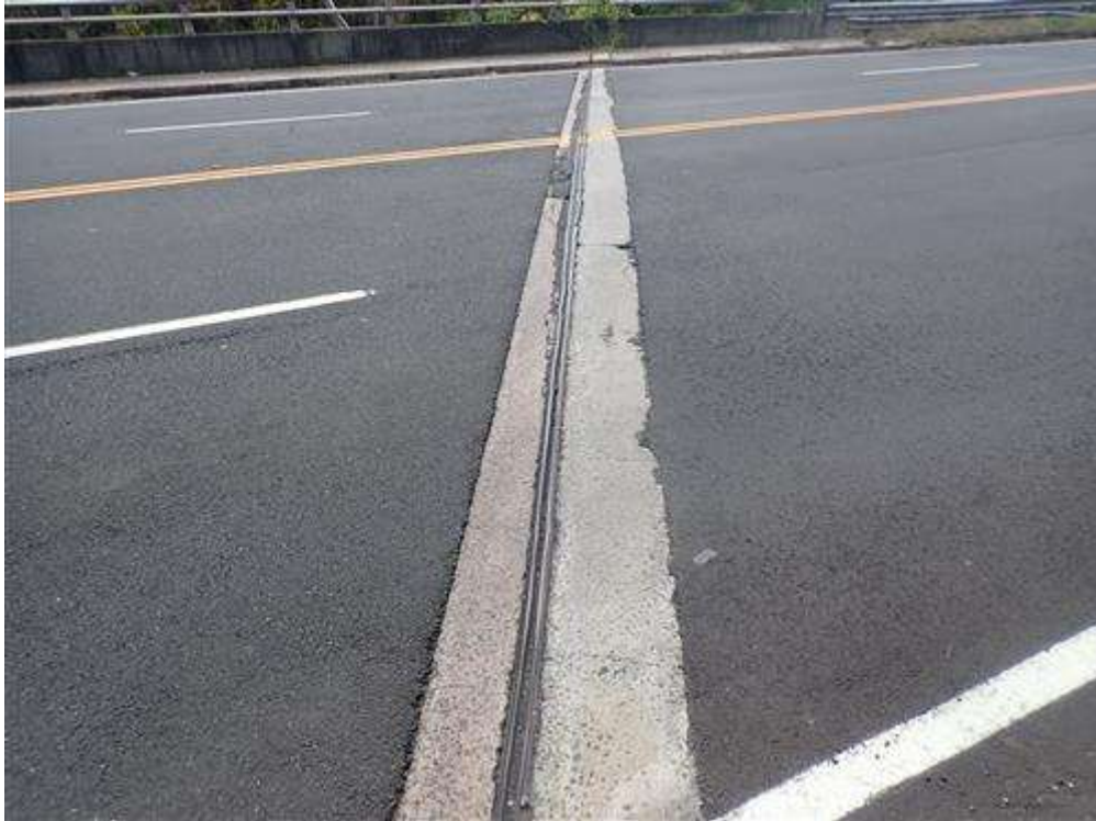
Joint over abutment 1
