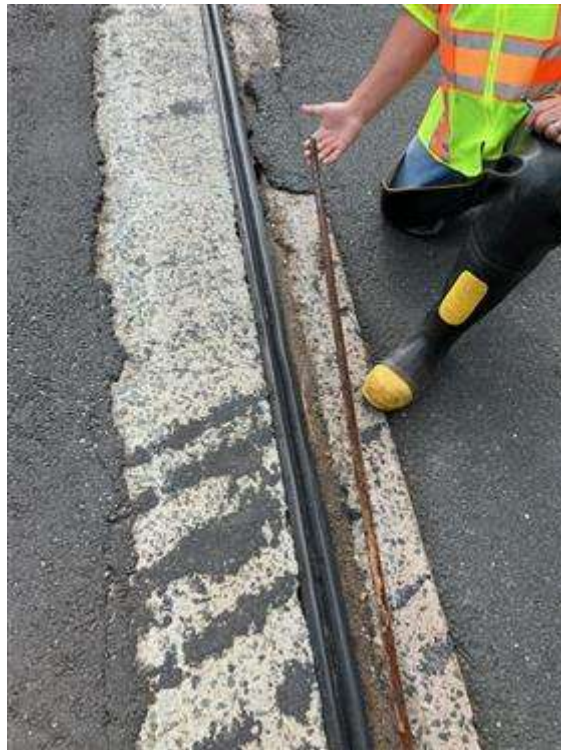
Compression seal joint header rebar is loose with free end in roadway.
