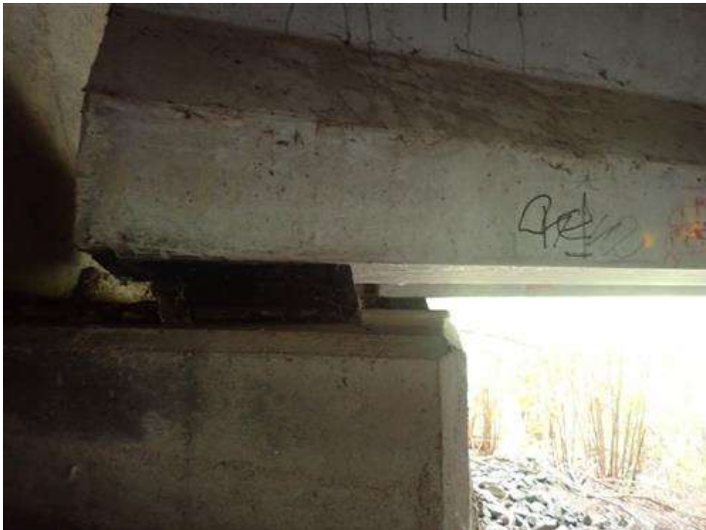
Typical bearing at abutment 2
