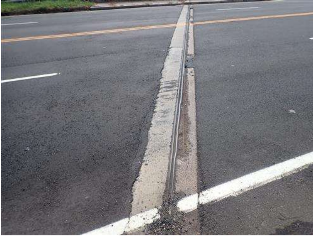
Joint over abutment 2
