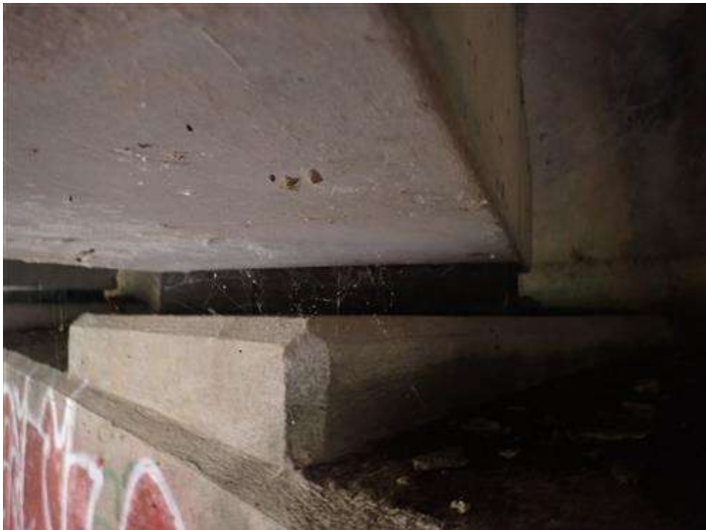
Typical bearing at abutment 1
