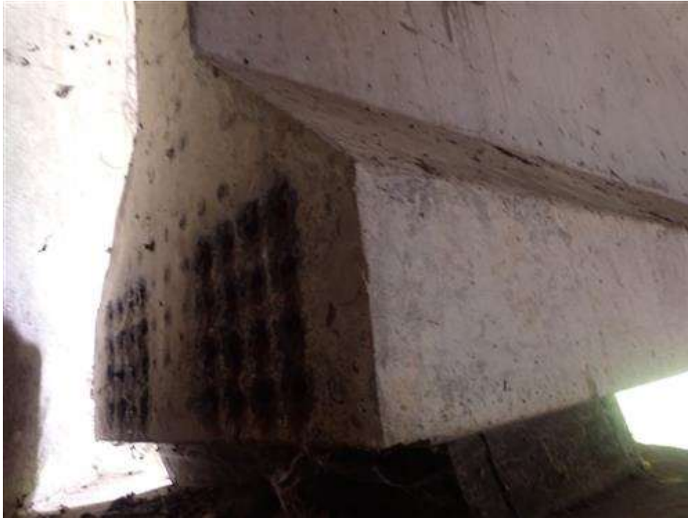
Typical strand on back side of beam 7 abutment 2 side
