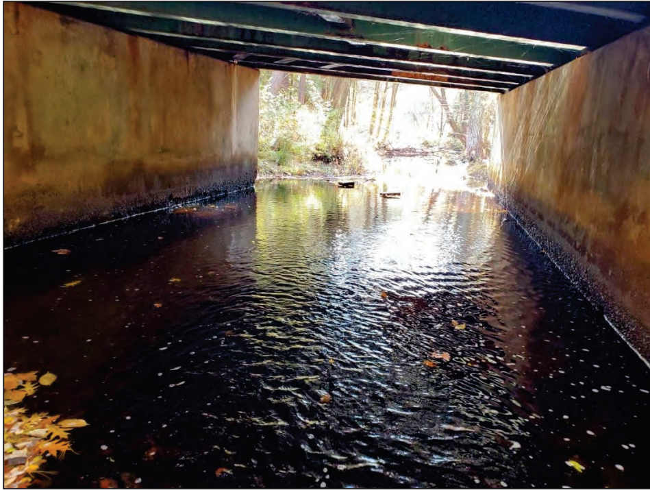
Photo No. 9 – Typical Underside looking east
