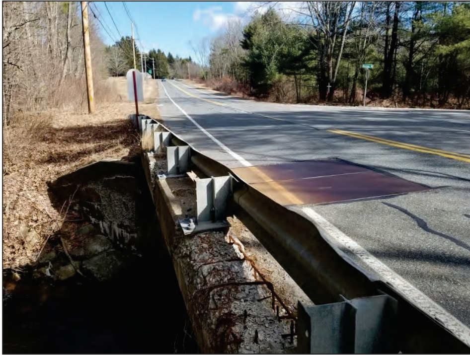
Photo No. 1 – ST 31 West fascia looking North
