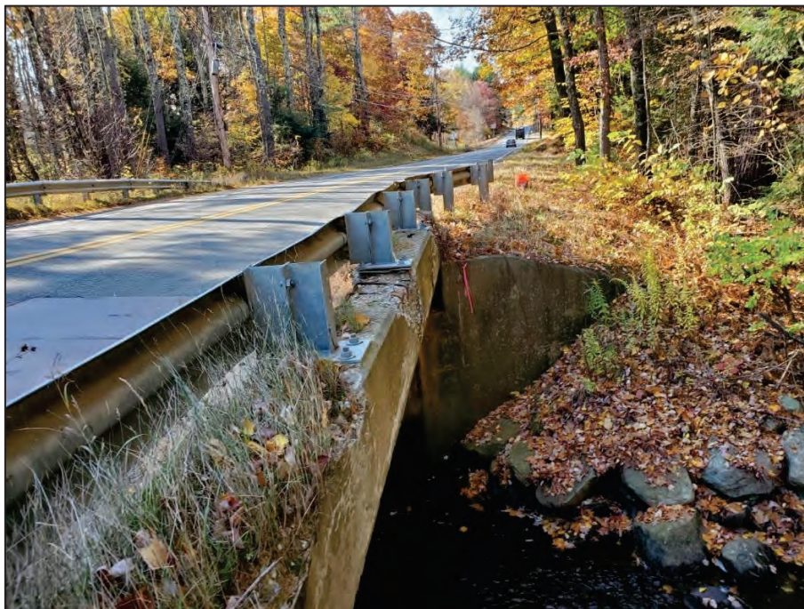
Photo No. 2 – ST 31 West fascia looking South
