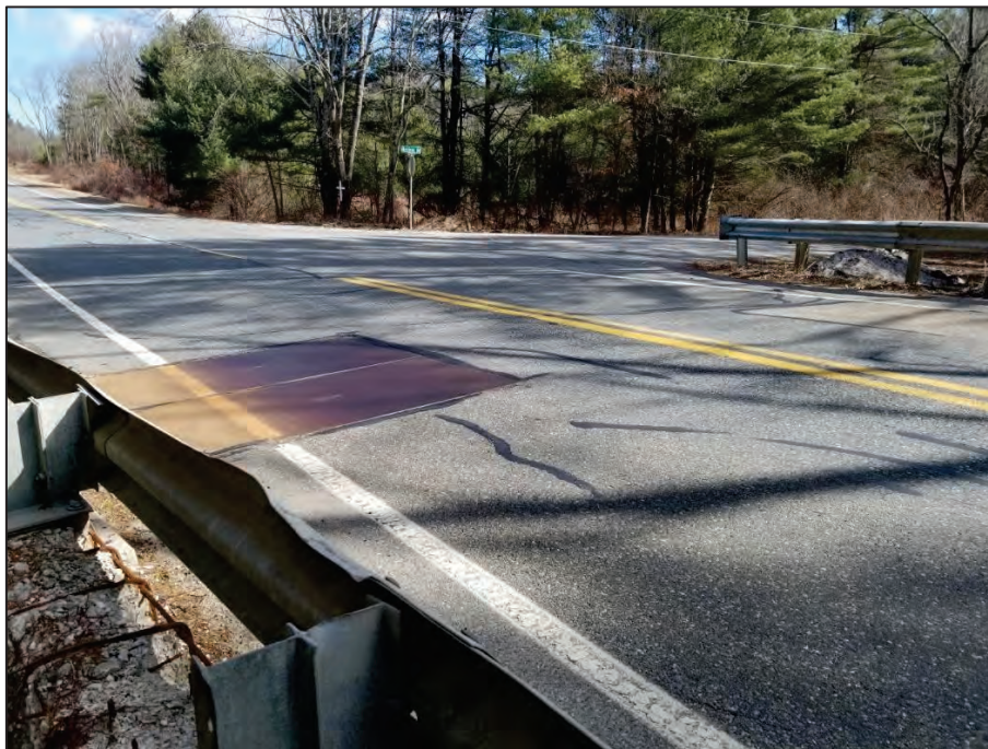
Photo No. 4 – ST 31 / Hastings Road intersection
