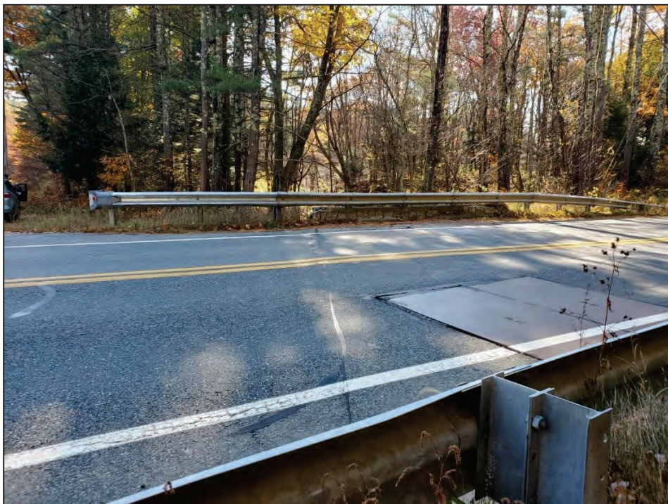
Photo No. 10 – Wearing Surface / road plates
