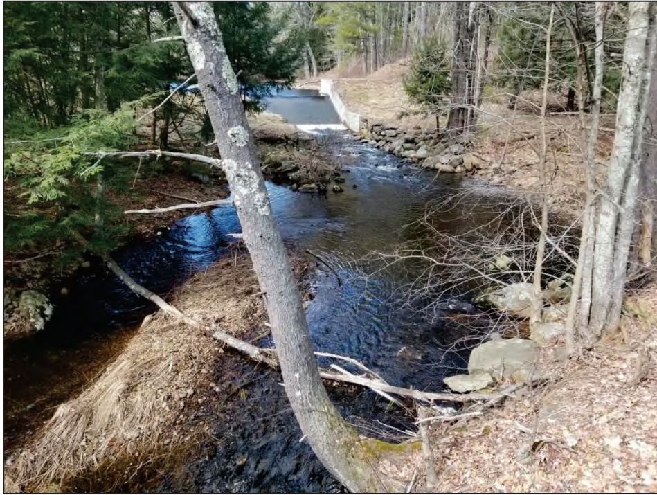
Photo No. 5 – Looking west at upstream channel
