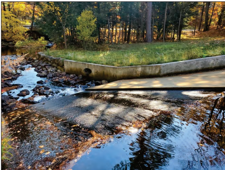
Photo No. 16 – Dam spillway
