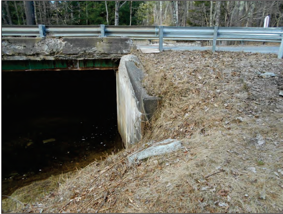
Photo No. 13 – Northeast quadrant
