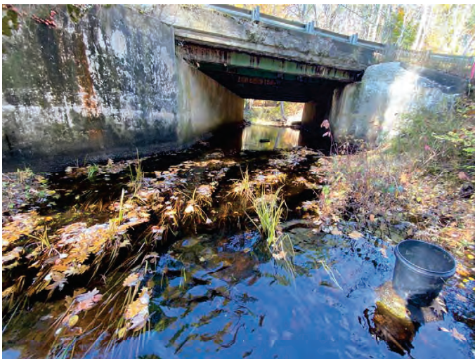
North Spencer Road bridge; this is where S. undulatus was detected.
