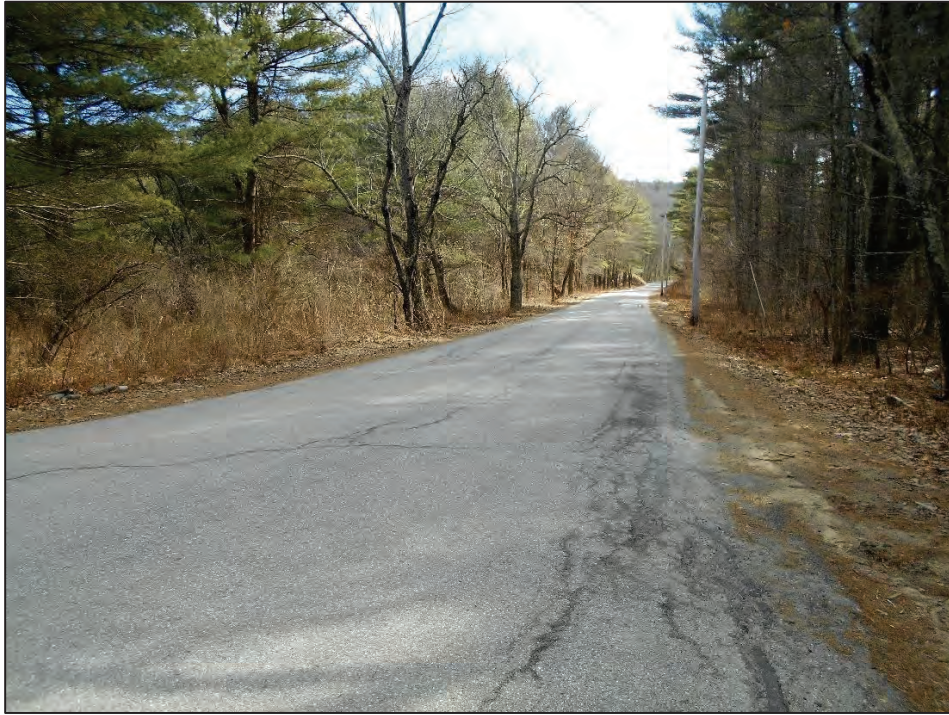
Photo No. 3 – Hastings Road looking East
