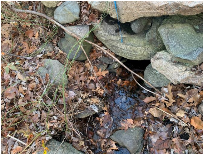
Photograph 1 – Stone headwall Culvert # 110 inlet
