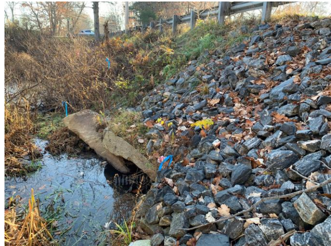
Photograph 4 – Stacked stone headwall Culvert #149 outlet
