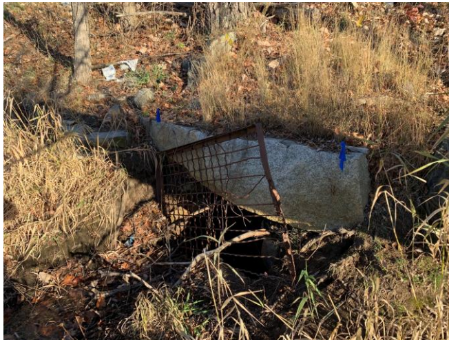
Photograph 3 – Stone headwall Culvert # 149 inlet
