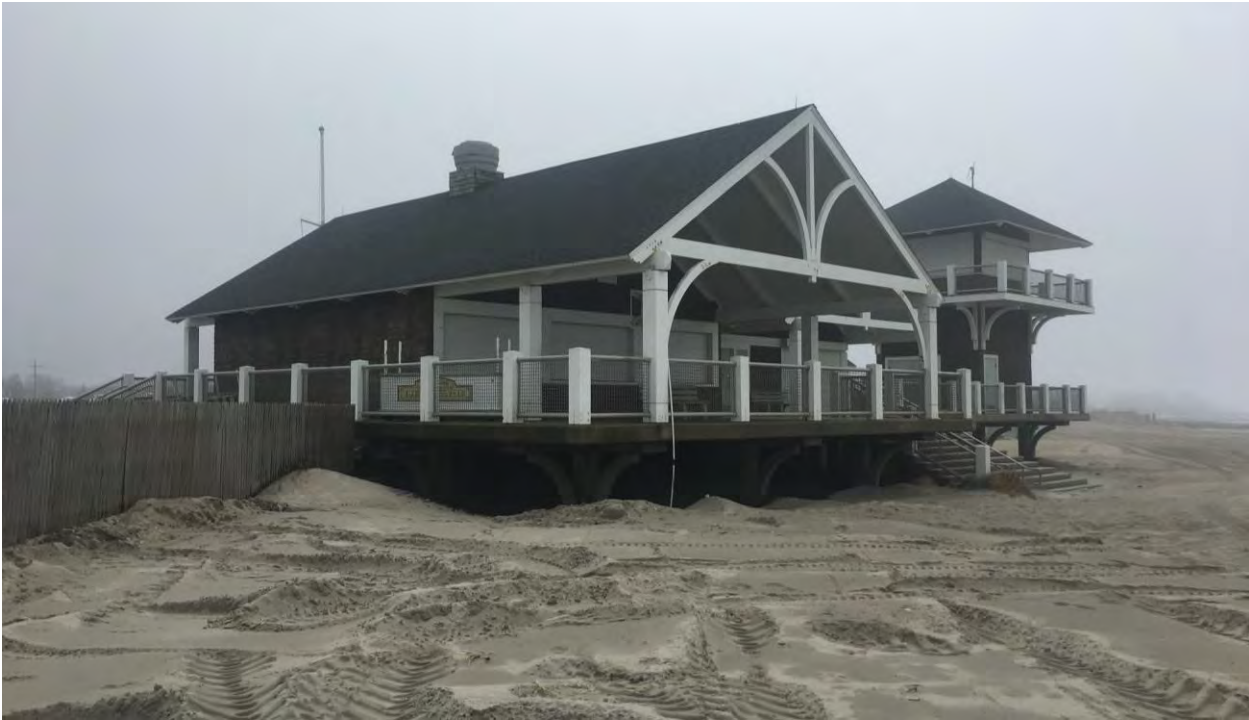
Photo No. 3: Existing concession building and environmental education area at center of beach along the existing bulkhead.
