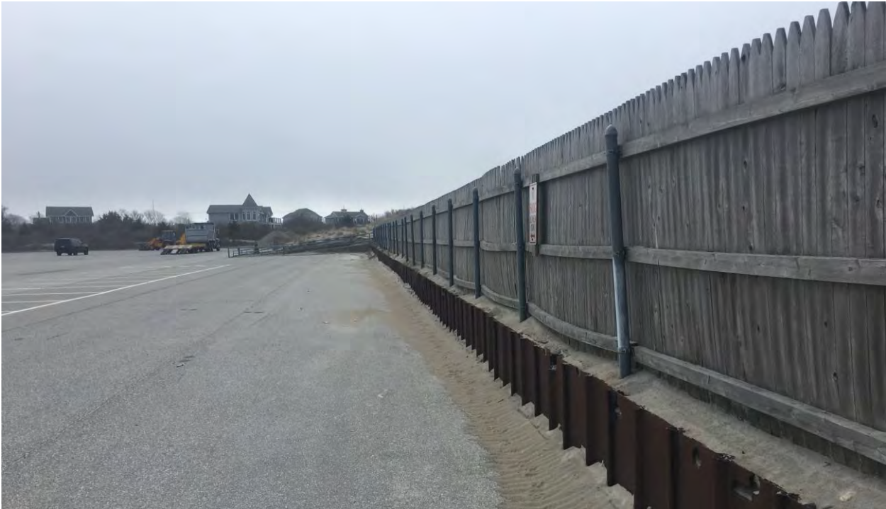
Photo No. 5: Easternmost extents of bulkhead, facing east
