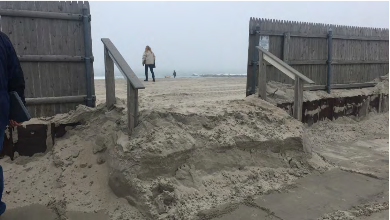
Photo No. 2: Example of sand drifts at stairs and along bulkhead impeding foot traffic
