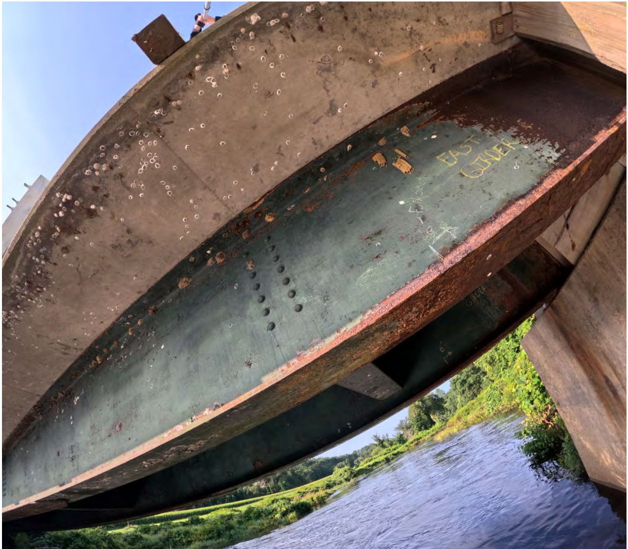
Photo 2: A southerly view of the steel beams and concrete abutments supporting bridge H-08-003=N-07-002.
