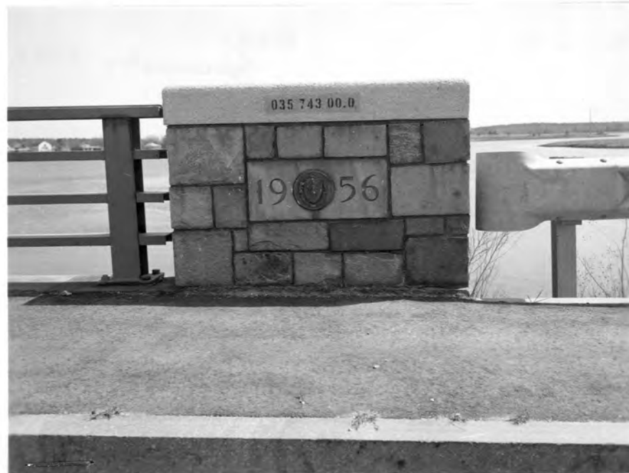
DATE & SEAL, SE CORNER (4/6/83)
