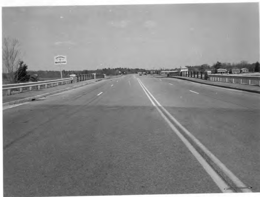
THRU VIEW LOOKING N (4/6/83)
