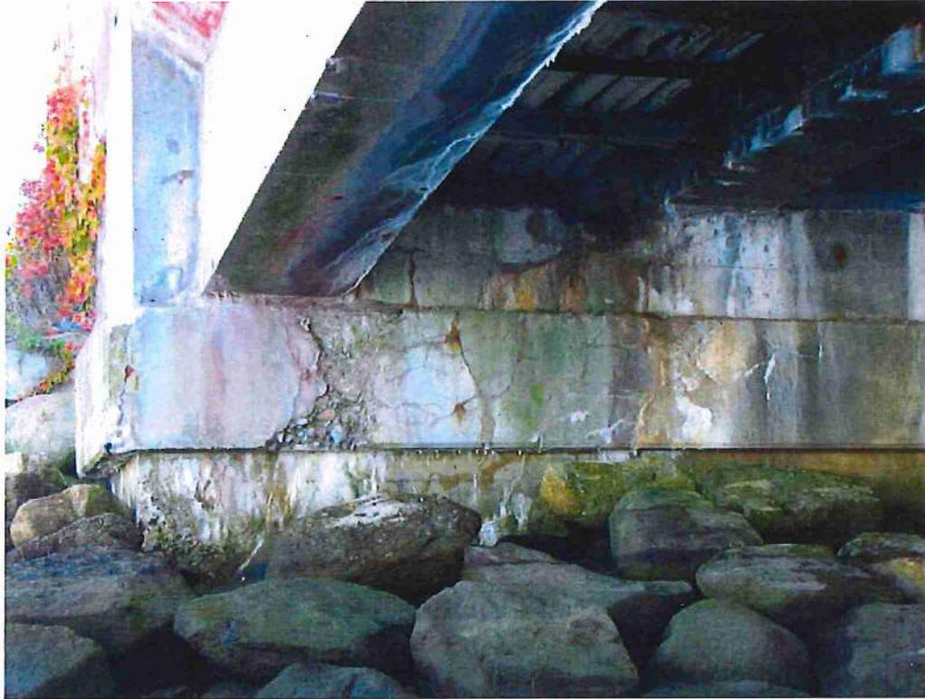
Photo 49: East abutment, at bay 1, north end
