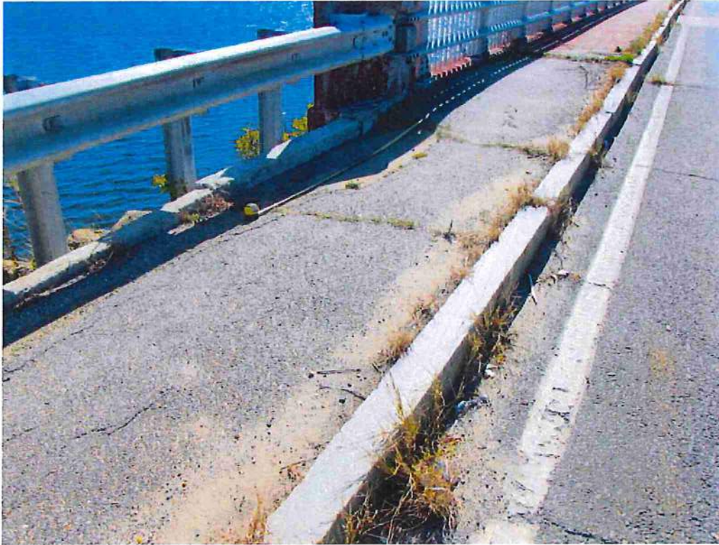
Photo 37: Overview of SE approach sidewalk
