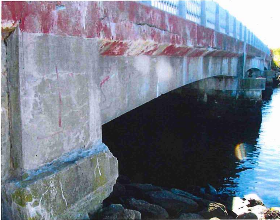
Photo 29: Overview of north face of sidewalk and deck
