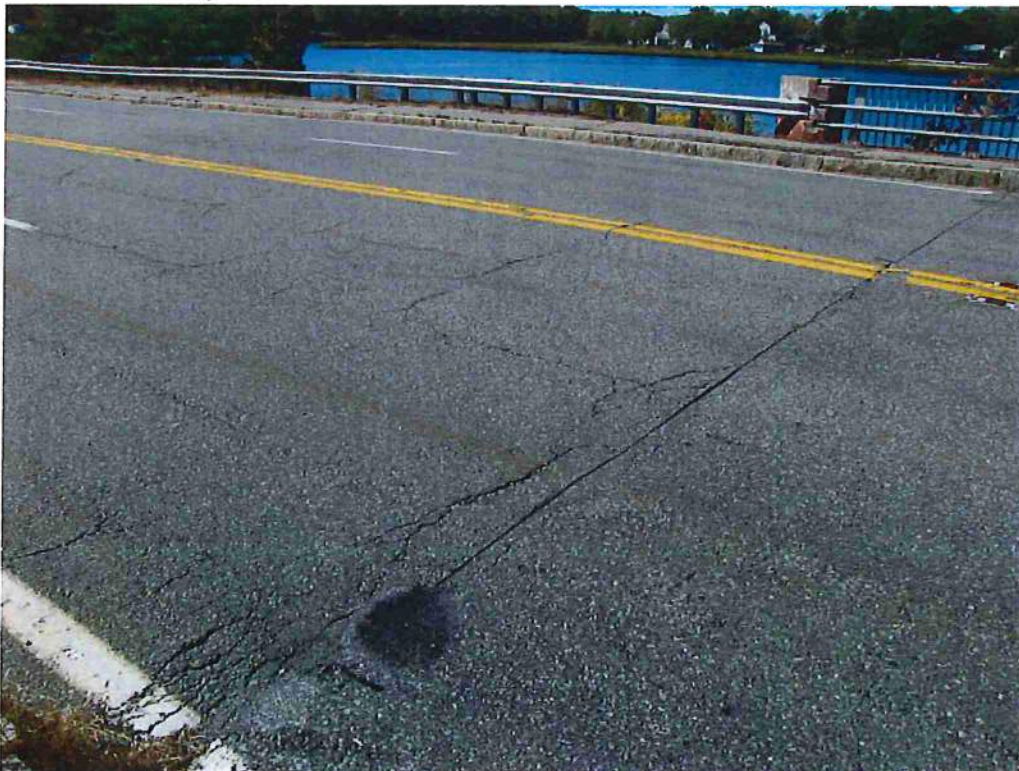
Photo 36: Overview of west approach pavement and sawcut joint. East approach pavement and sawcut joint is similar
