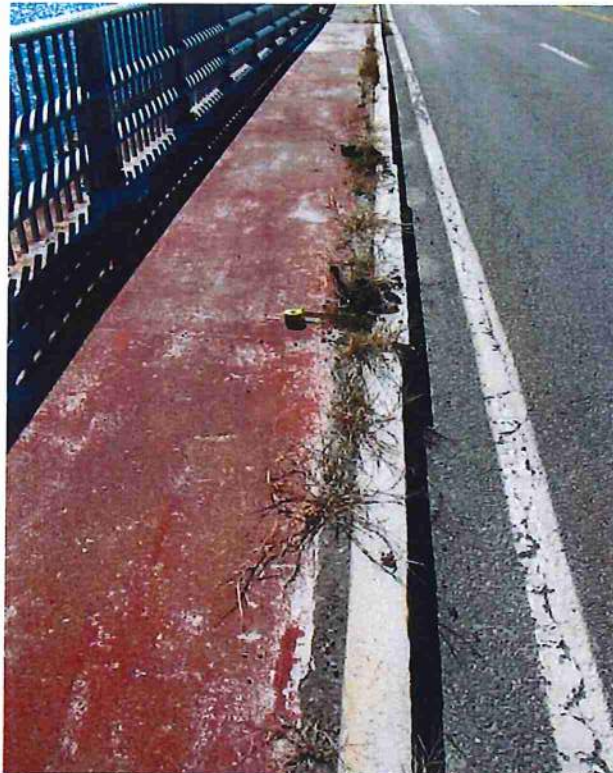
Photo 31: South sidewalk looking west
