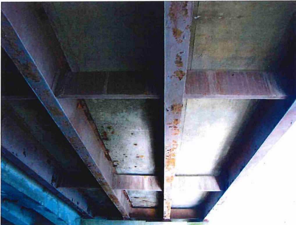
Photo 20: General underside of span 1 (south extension) looking east
