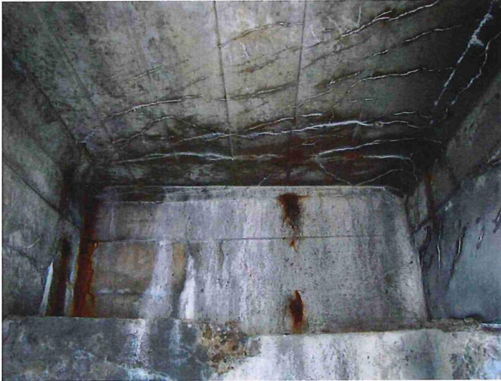
Photo 19: Span 1, bays 2 at west abutment
