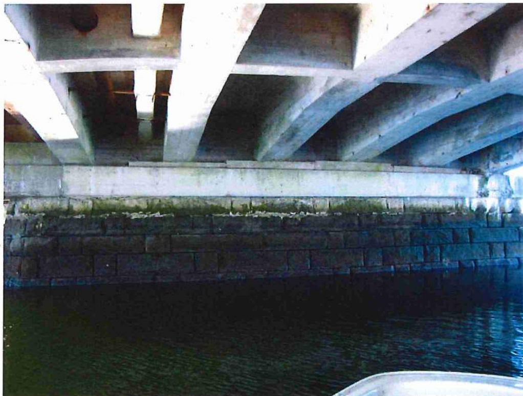
Photo 52: Overview of pier 1, east face
