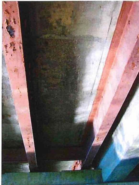
Photo 22: Close up of previous photo, bay 1 near pier 1
