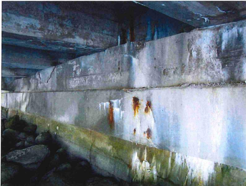
Photo 46: Overview of west abutment
