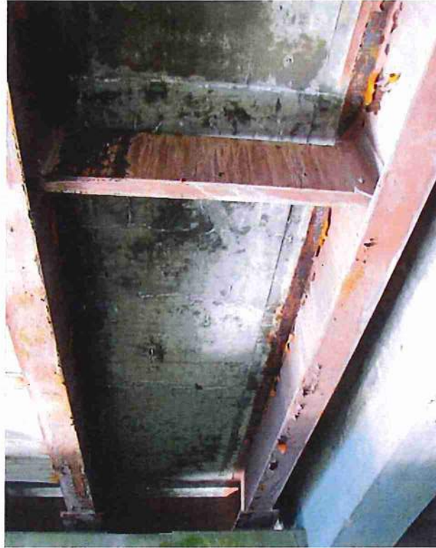
Photo 25: Close up of previous photo, bay 1 near pier 2
