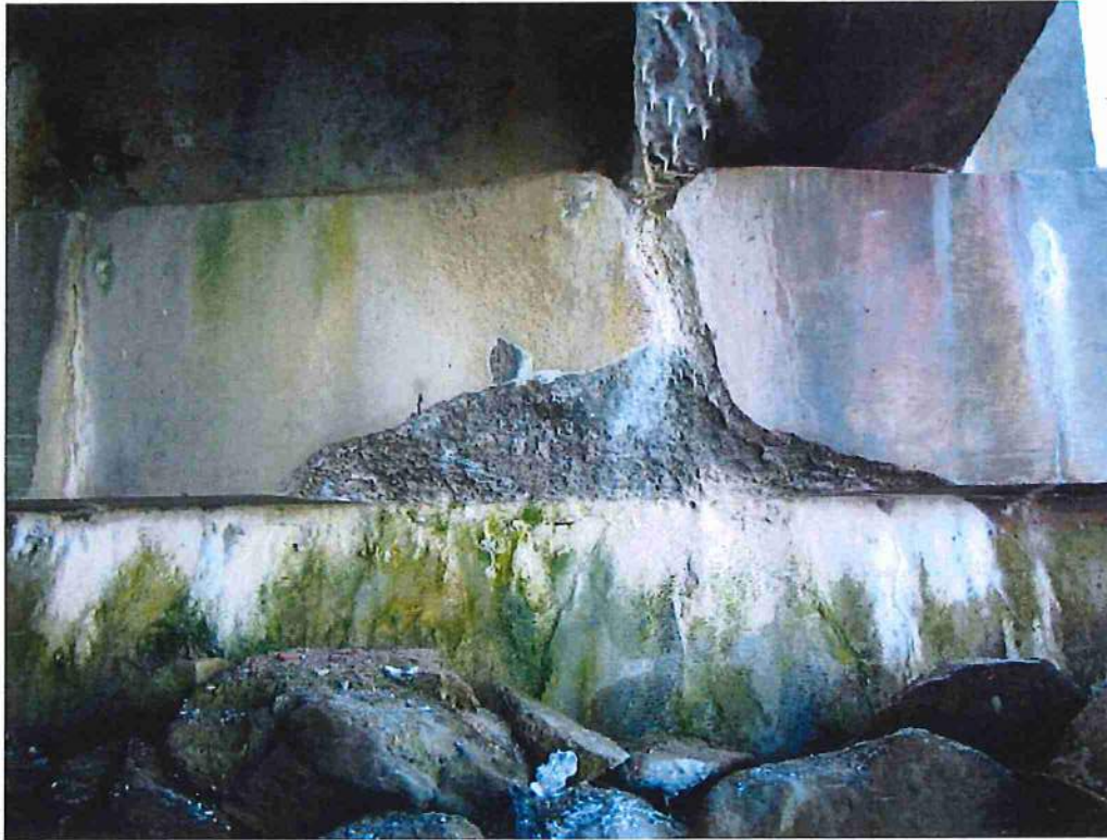
Photo 47: West abutment, at bay 1, north end
