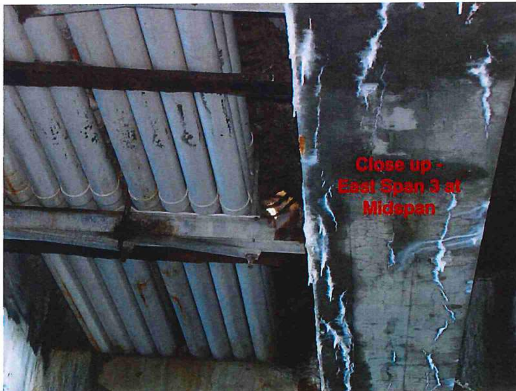
Photo 14: Close up of previous photo. Area below photo 12 looking east
