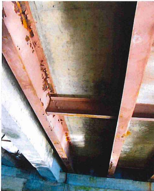
Photo 26: Span 3 bay 1 and 2 (L to R) near east abutment
