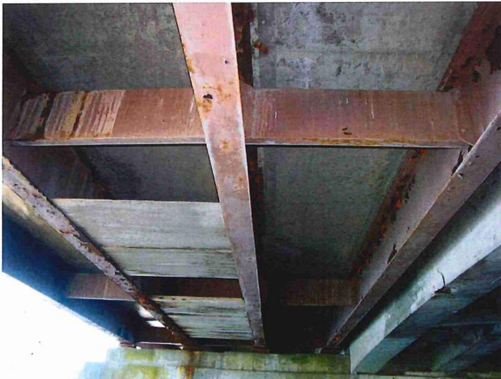
Photo 24: General underside of span 3 (south extension) looking west
