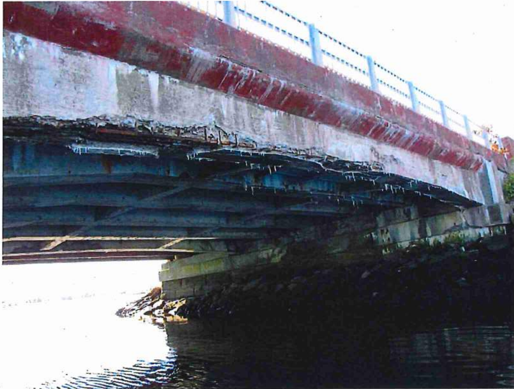
Photo 41: Overview BM 1, span 1, north face and bottom
