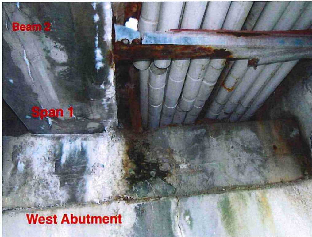
Photo 7: Underside of previous photo looking west. Span 1, bay 1 at west abutment
