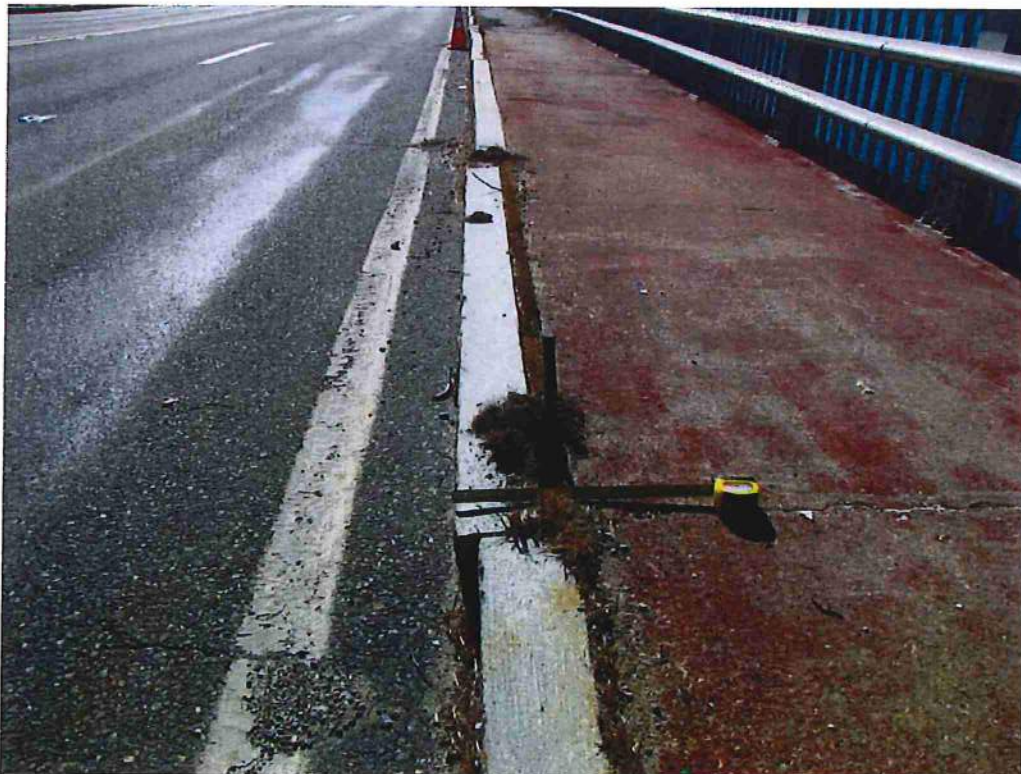
Photo 32: North sidewalk, span 2 looking west
