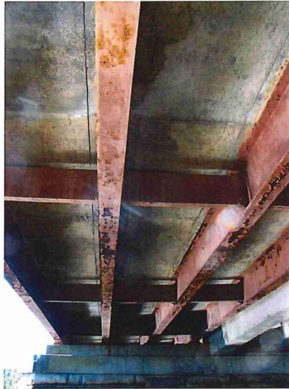
Photo 21: General underside of span 2 (south extension) looking west
