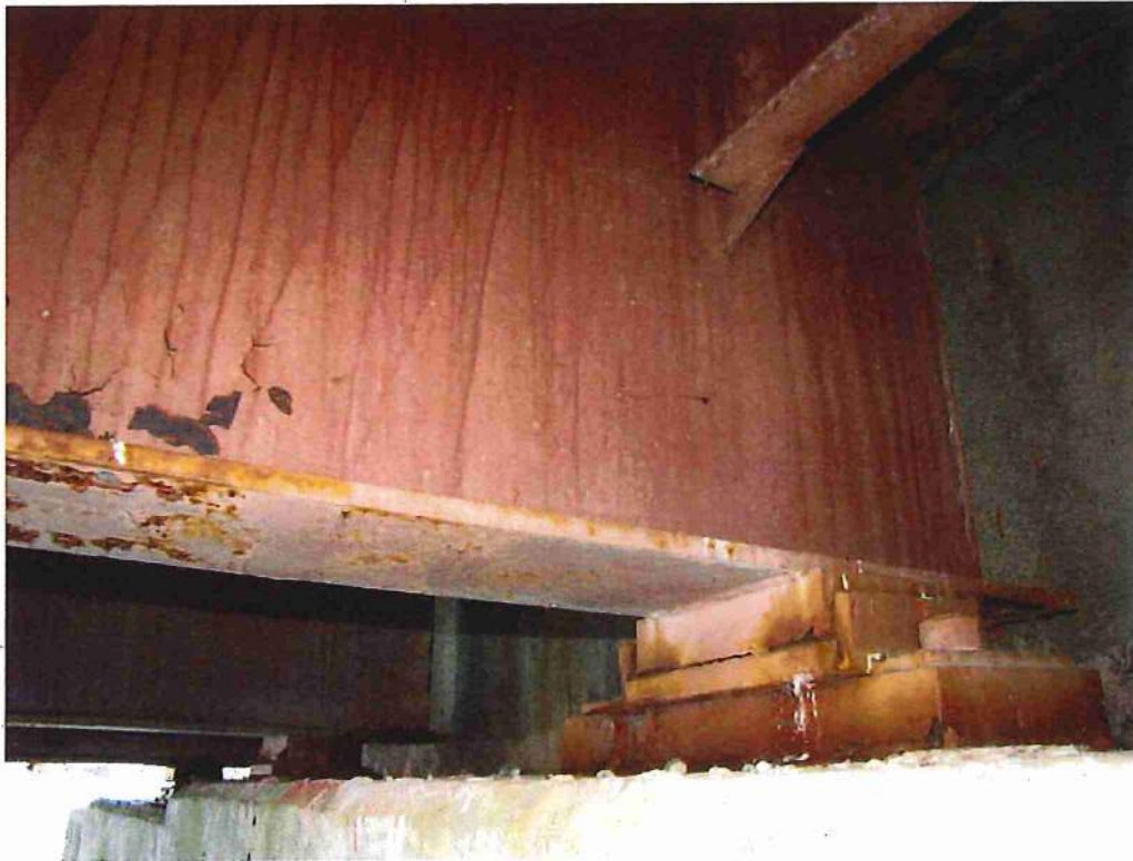
Photo 39: BM 2, north face at west abutment. Typical beam end at abutments
