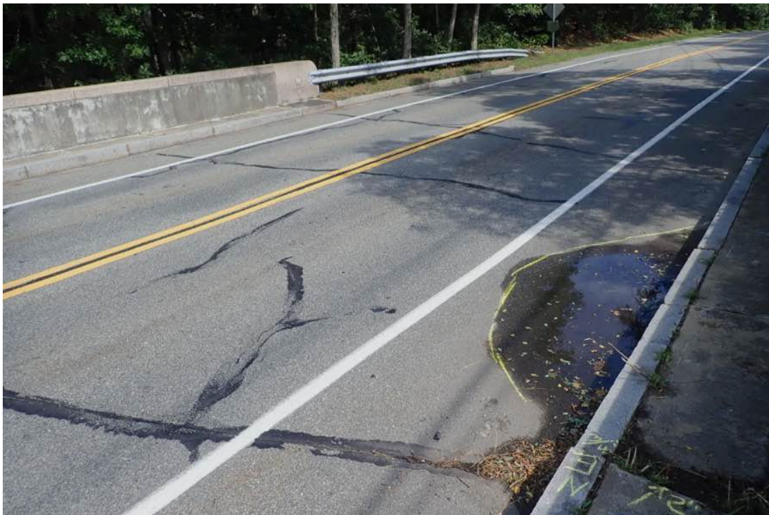
Photo 7: Looking NW over north approach pavement, severe rutting in the wheel paths, sealed/unsealed cracks and NE sidewalk/curb settlement (Ponding).
