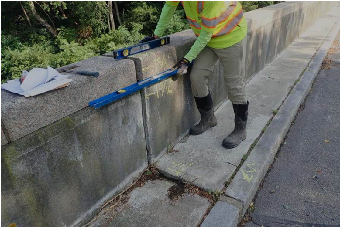
Photo 5: Looking NW at SW corner, parapet field measurements and sidewalk/curb settlement.
