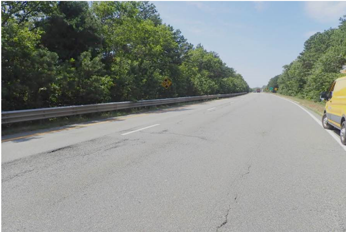
Photo 2: Looking west between Mile Markers 68.4 & 68.6 south of exit 68, height posting sign obscured with vegetation and a sign is missing.
