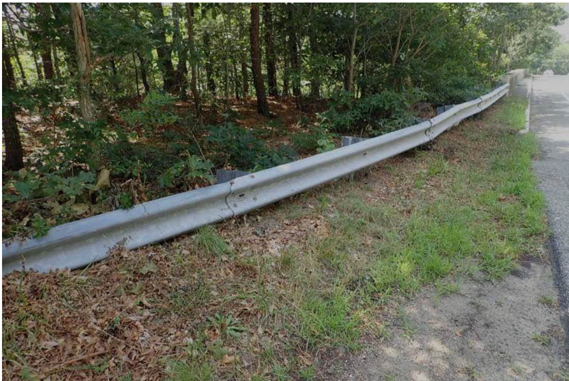
Photo 13: Looking south at NE approach guardrail, panels damaged FL.
