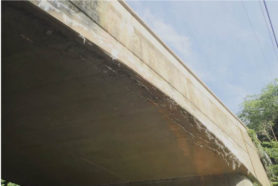
Photo 9: Close up of previous photo (East Soffit Edge), FL active efflorescence with HL densely spaced longitudinal cracks.
