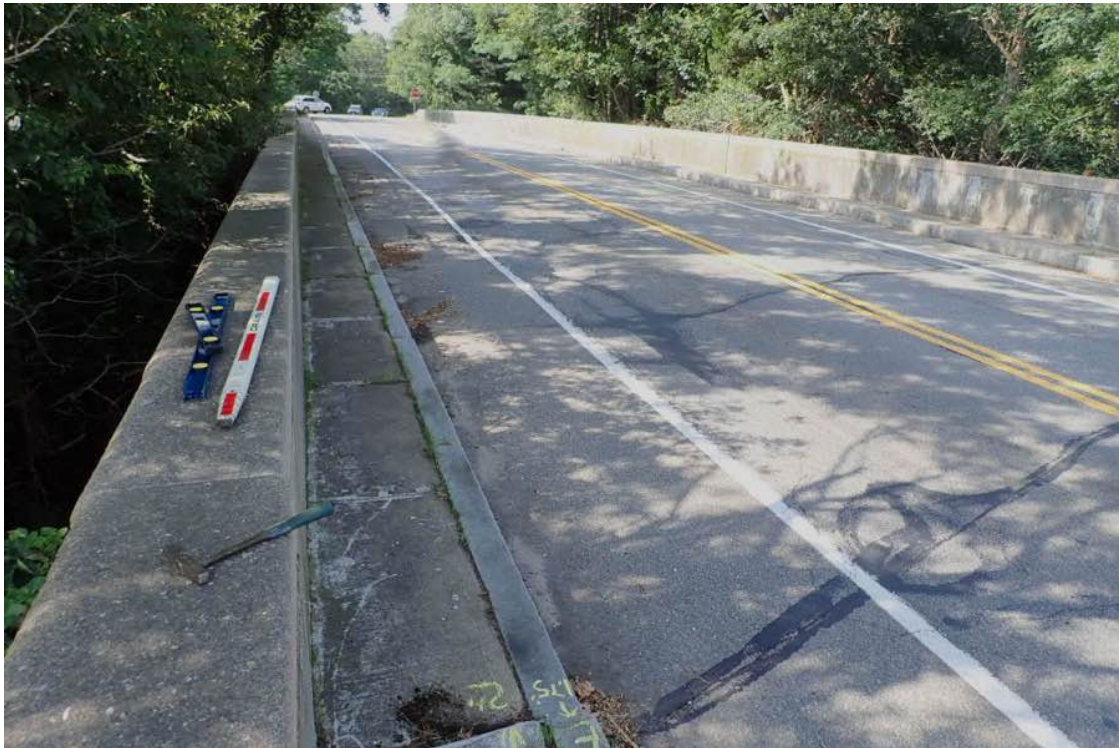
Photo 6: Looking south over north approach pavement, severe rutting in the wheel paths, sealed/unsealed cracks and SE sidewalk/curb settlement.
