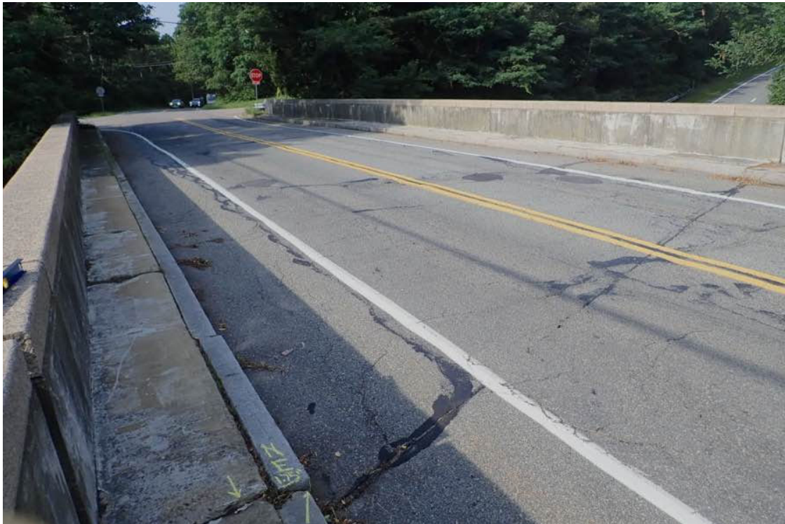
Photo 3: Looking SW from the NE over wearing surface, severe rutting in the wheel paths, sealed/unsealed cracks and isolated/random asphalt filled potholes.
