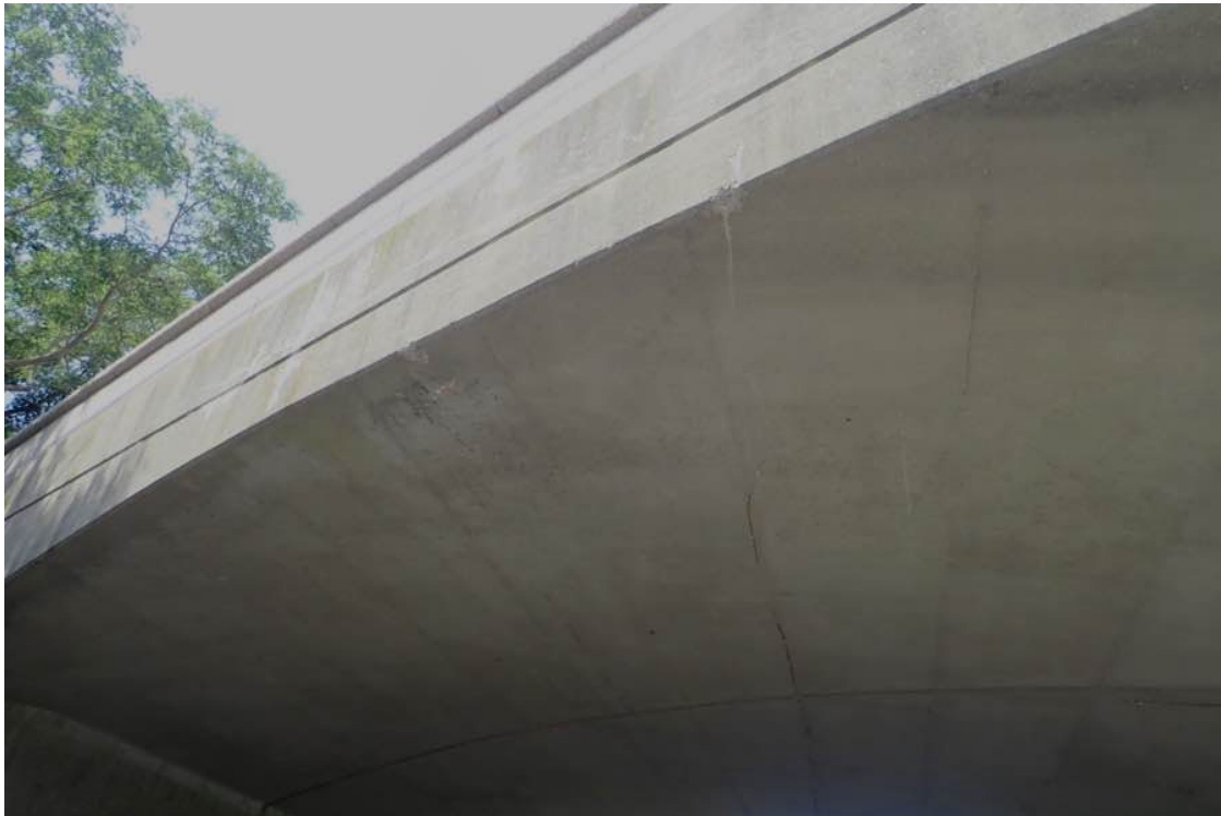
Photo 12: Looking west at east edge of rigid frame soffit, two entry spalls and FL scrapes over both lanes.
