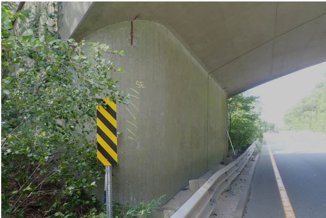
Photo 11: Looking west at SE corner of rigid frame leg, spall at the top and delamination below. Vegetation encroaching.
