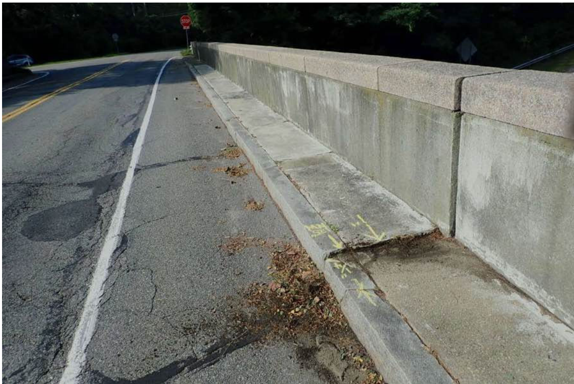
Photo 4: Looking south at NW corner, sidewalk settlement, severe rutting in the wheel paths, sealed/unsealed cracks and isolated/random asphalt filled potholes.
