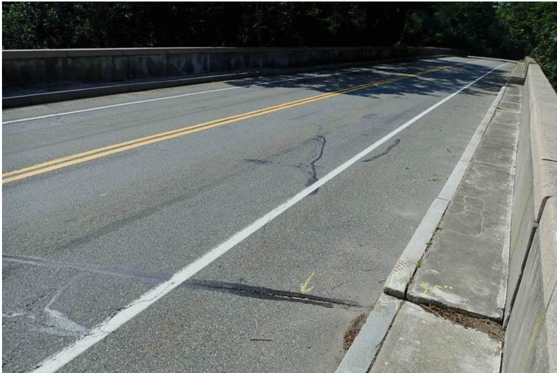
Photo 4: Looking SE from the NW over wearing surface, severe rutting in the wheel paths, sealed/unsealed cracks and NW approach sidewalk settlement.
