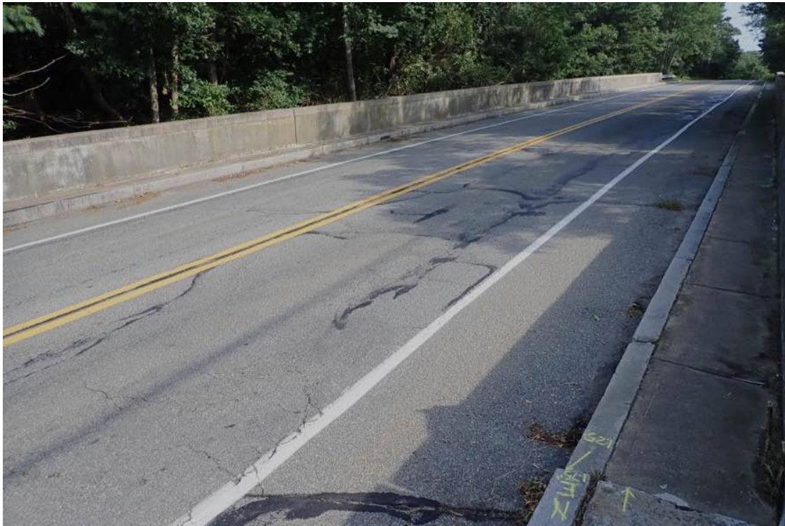
Photo 7: Looking NW over north approach pavement, continued wearing surface deficiencies and NE corner sidewalk/curb settlement.
