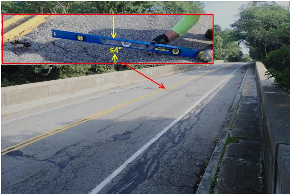
Photo 2: Looking NW from the SE over wearing surface, severe rutting in the wheel paths, sealed/unsealed cracks and isolated/random asphalt filled potholes.
