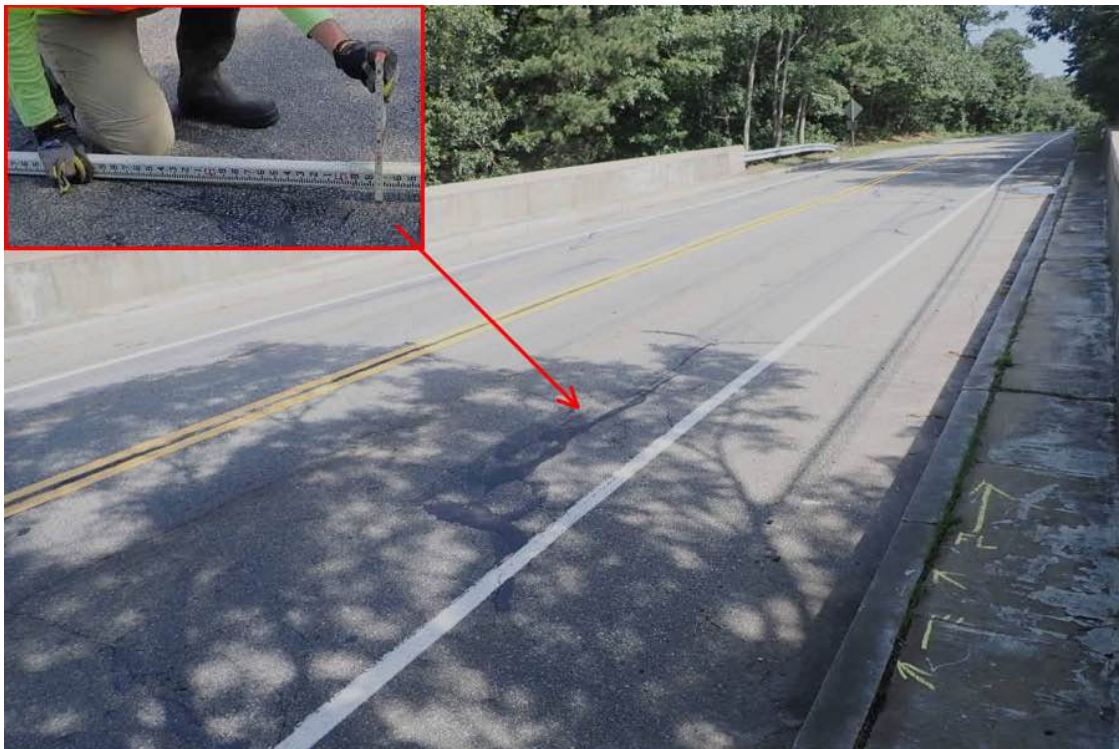
Photo 3: Looking NW from the SE over wearing surface, severe rutting in the wheel paths, sealed/unsealed cracks and isolated/random asphalt filled potholes.
