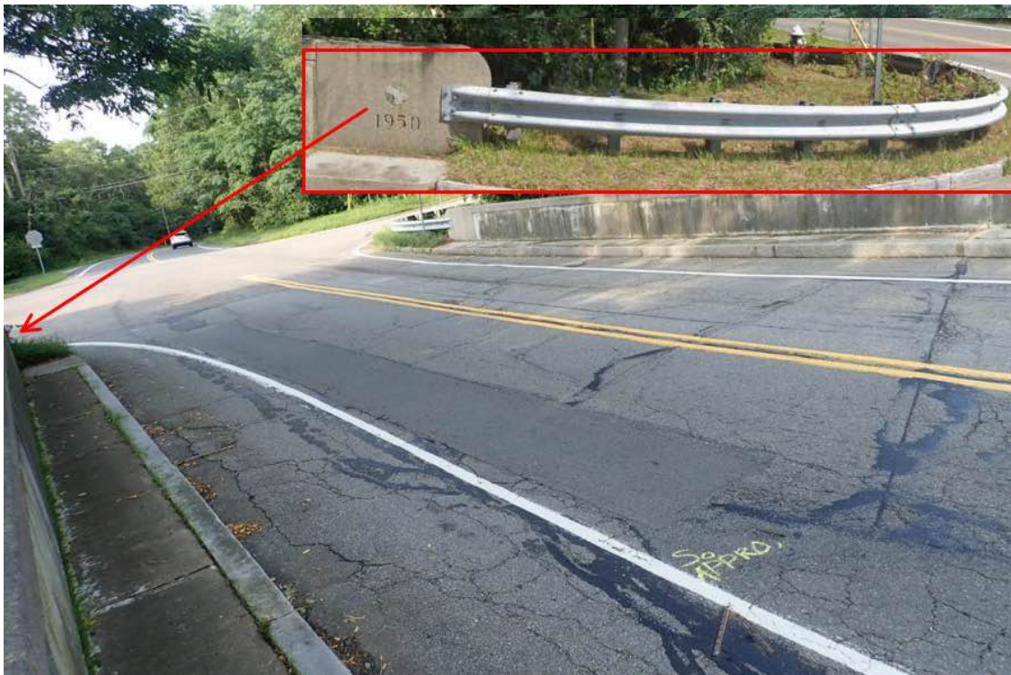
Photo 6: Looking SW over south approach pavement, continued wearing surface deficiencies with FL asphalt patch in NB lane.
