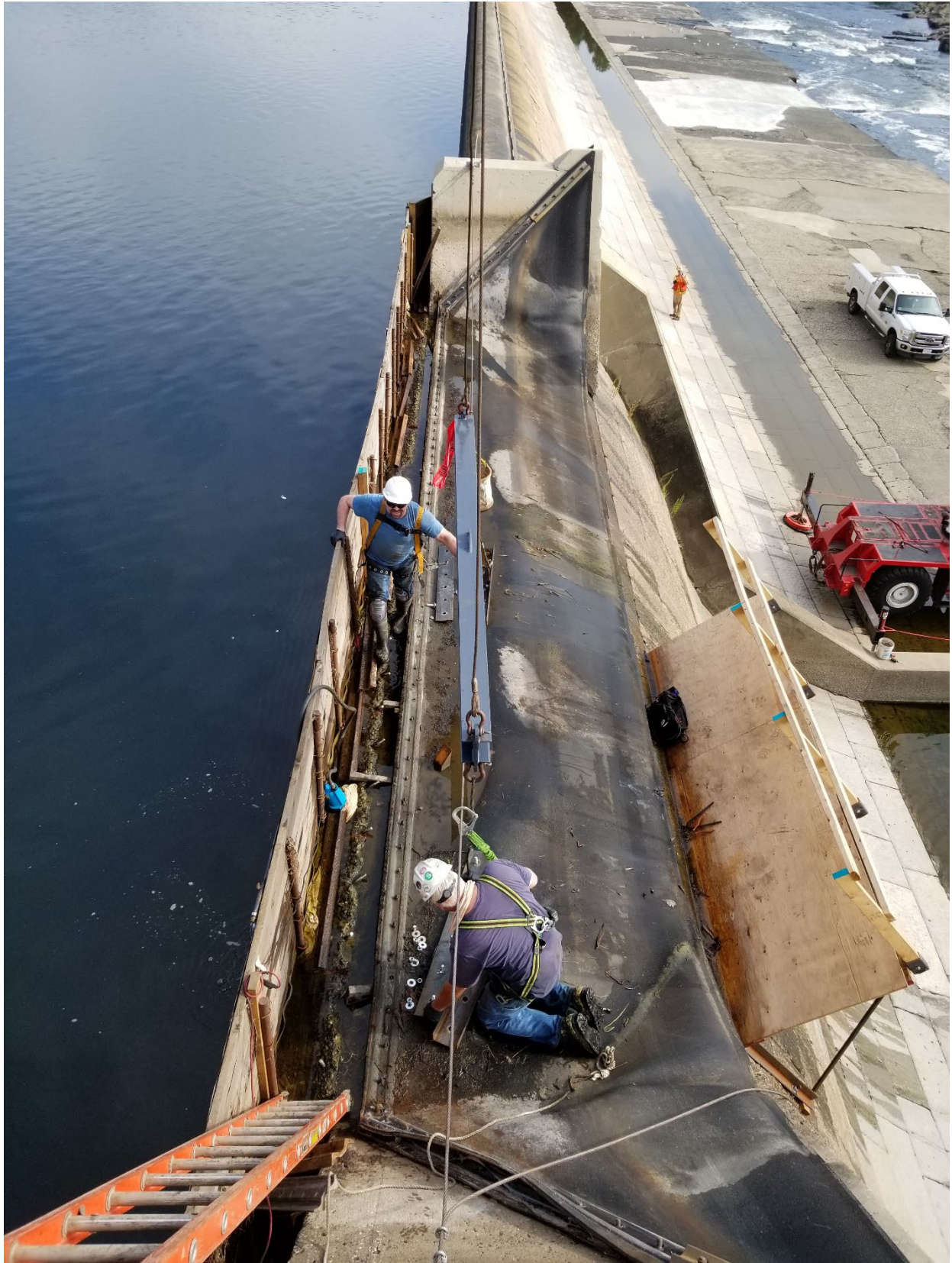
2019 Rubber Dam # 5 Repair
