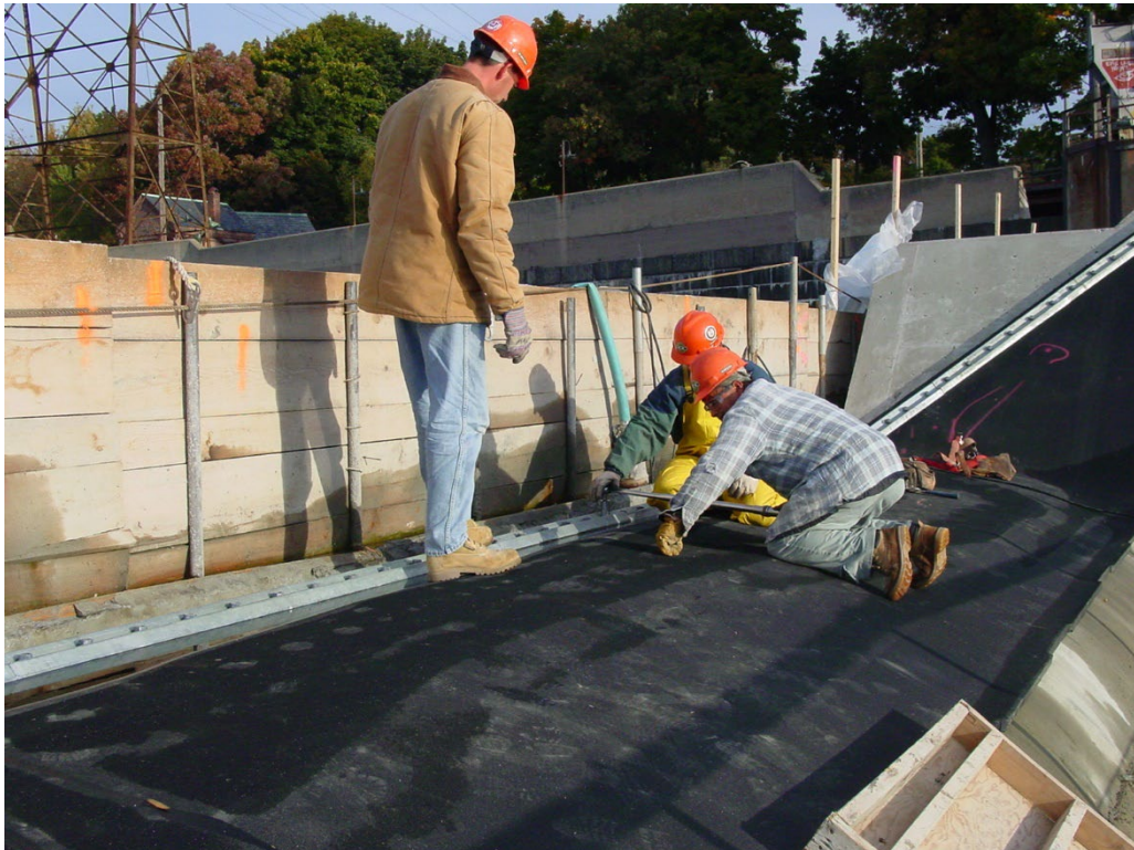
Torquing clamp bar Bladder #2
