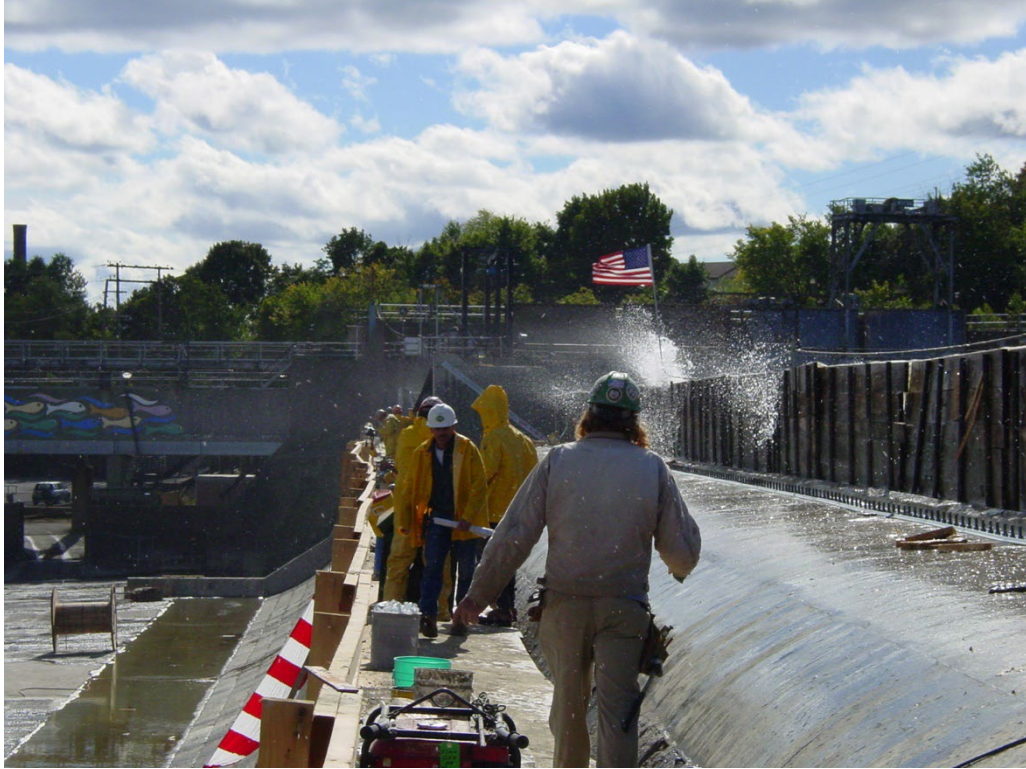
Windblown water over flashboards
