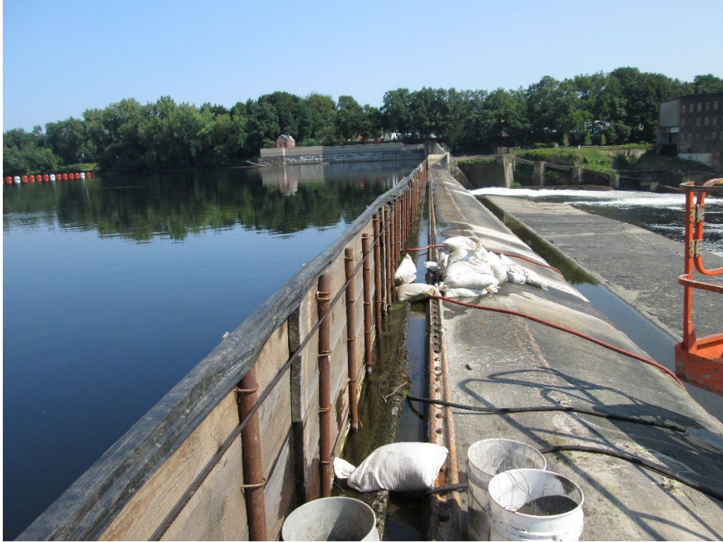
2013 Rubber Dam #3 Repair
