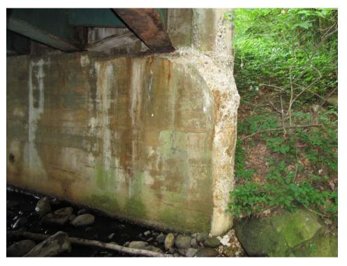
**Photo 8:** View of spall to the bridge seat and breastwall end under around Beam #1 at the east breastwall.
