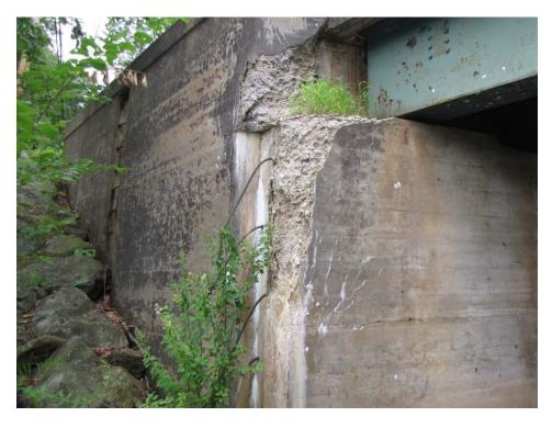
**Photo 6:** View of spall to the north end of the east breastwall and backwall.
