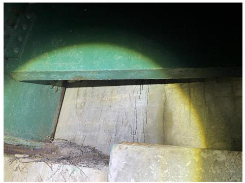
Figure 4. Gap above abutment on Bridge H-24-003 over Burnshirt River
