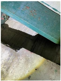
Figure 7. Space between abutment and bridge deck on Bridge H-24-003 over Burnshirt River
