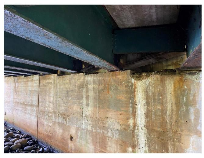
Figure 3. Example photograph of top of bridge abutment and connection with steel I-beams on Bridge H-24-003 (Williamsville Road over Burnshirt River).
