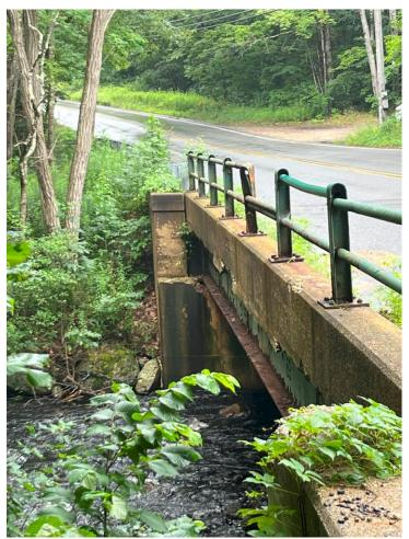
Figure 2. Guardrails and abutment of bridge H-24-003 over Burnshirt River.
