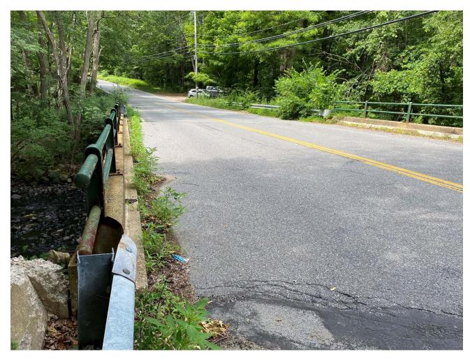
Figure 4. Solid metal guardrails and bridge approach guardrail structure (in foreground) on Bridge H-24-003 (Williamsville Road over Burnshirt River).
