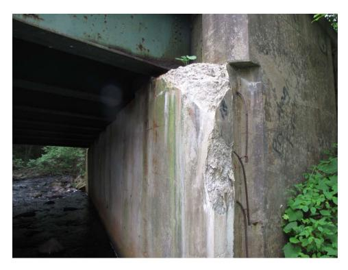
**Photo 7:** View of spalls to the north end of the west breastwall.
