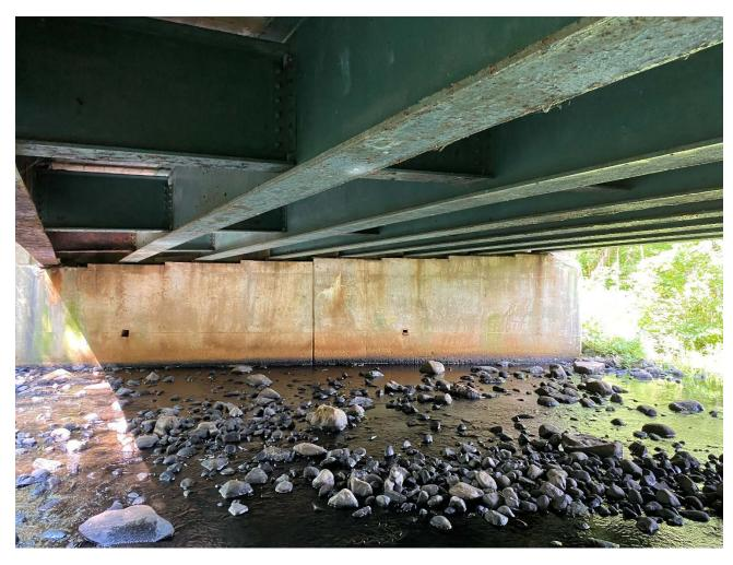
Figure 2. Steel I-beams, concrete abutment, and weep holes along underside of Bridge H-24-003 (Williamsville Road over Burnshirt River).
