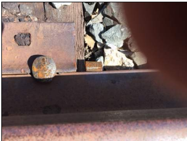
Tie Plate with Anchors Applied Correctly
