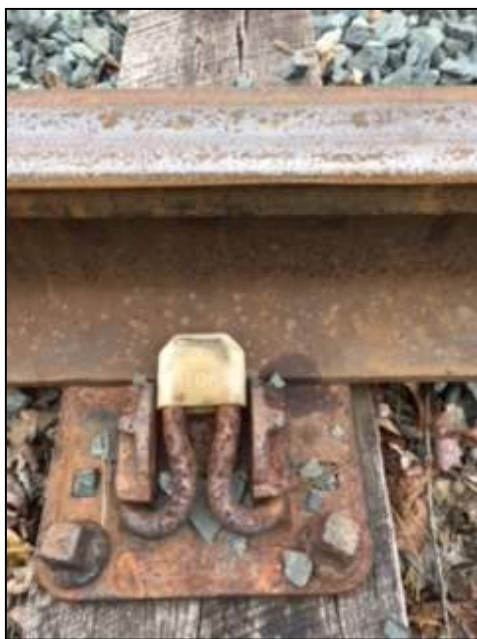
Elastic Fastener: Pandrol Fast Clip
