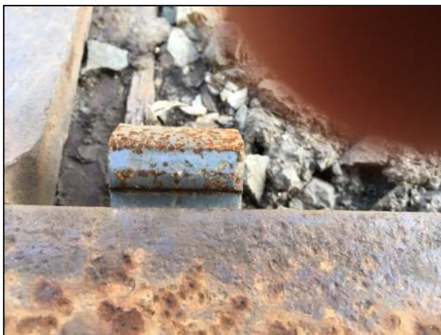
Tie Plate with Anchors Overdriven
