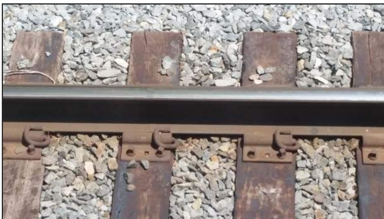
Elastic Fastener: Pandrol E-Clip
