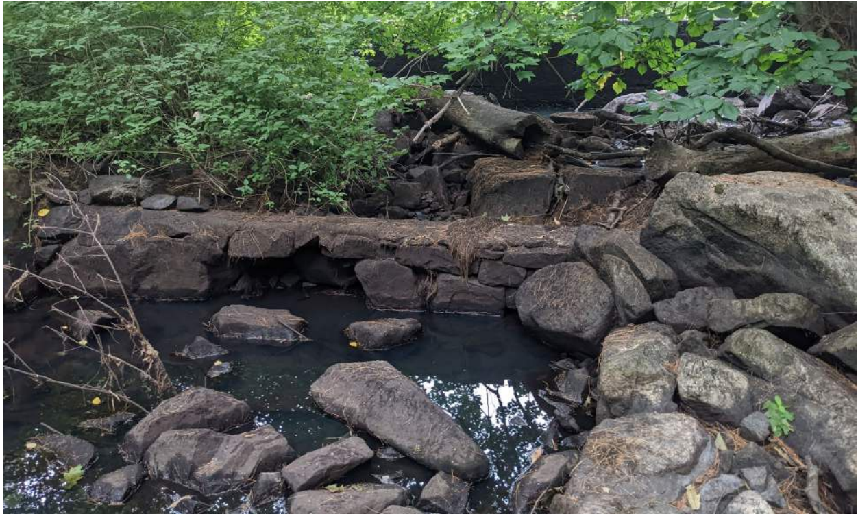
South masonry fish weir with spillway in background
