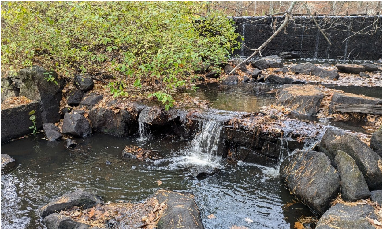
South masonry fish weir with spillway in background and fishway entrance at left
