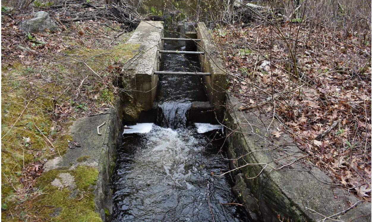
Upstream fishway exit into impoundment (looking southwest)
