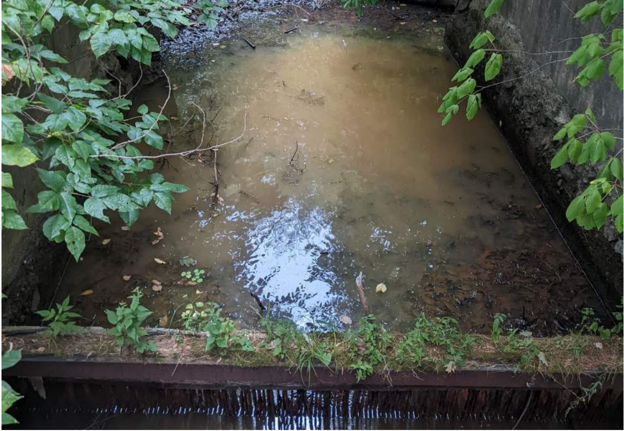
Trashrack and channel bottom during drought conditions
