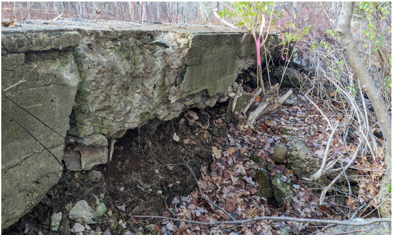
Right (south) abutment deterioration, looking northwest toward spillway
