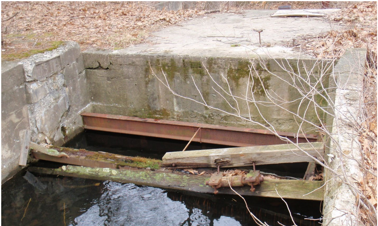
Former headgate/trashrack structures and headwall
