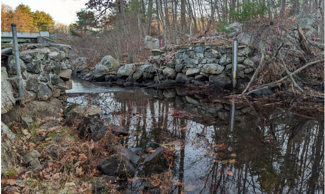
Weir abutments, looking downstream (note stream gaging equipment at left and right)
