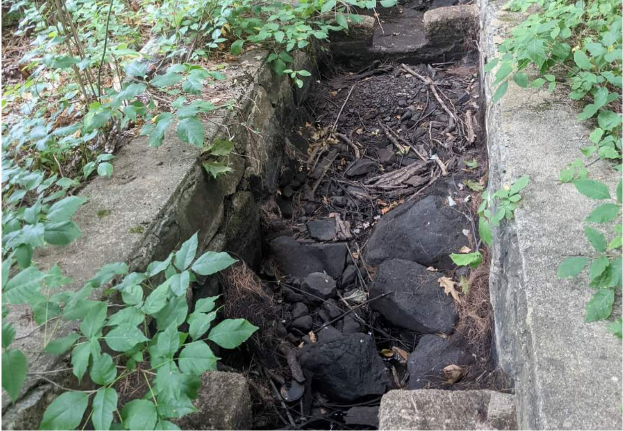
Dewatered fishway showing bottom substrate
