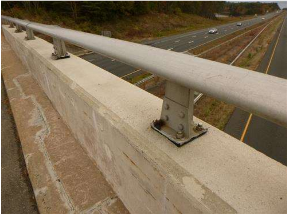
East parapet railing post 13 with loose anchor bolt nuts.
