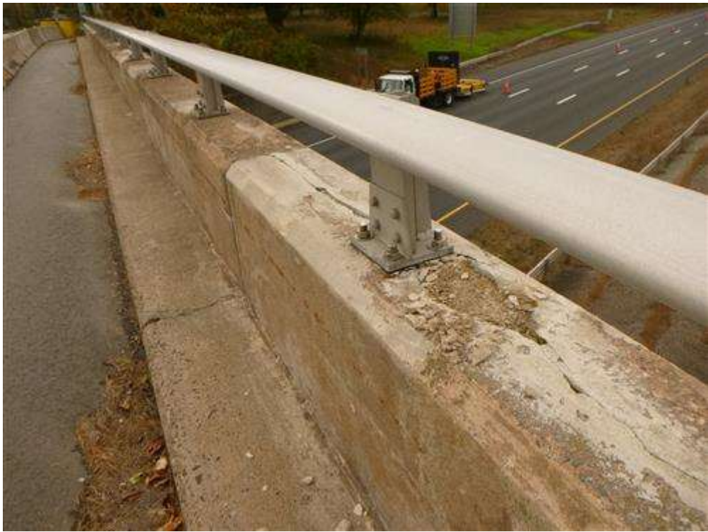
West parapet over the pier. Note the spall around the post.
