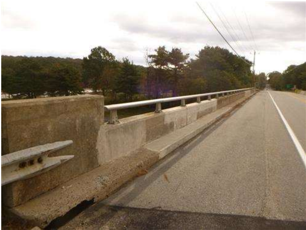
East parapet, bridge railing, and safety walk.
