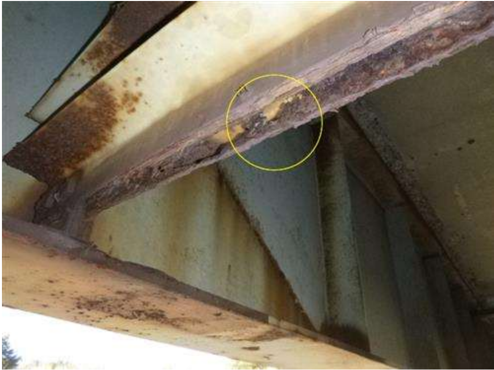
Photo Number: 28 Span 2, bay 1, second diaphragm with a rusted through hole in the lower angle. Photo Taken: 10/17/2023
