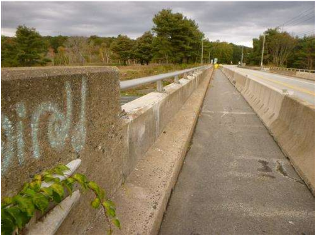
West parapet, bridge railing, safety walk, and jersey barrier.
