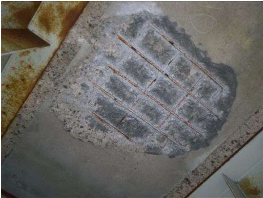
Span 2, bay 3, panel 2. Note spall with debonded rebar.
