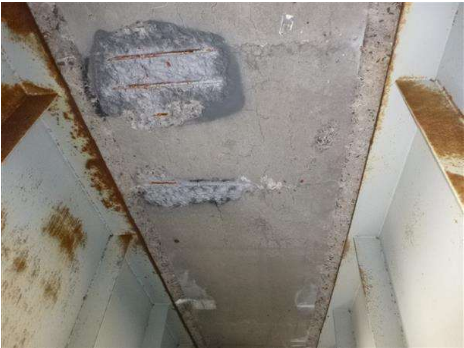
Span 2, bay 3, panel 3. Note spalls with exposed rebar and adjacent hollow areas.
