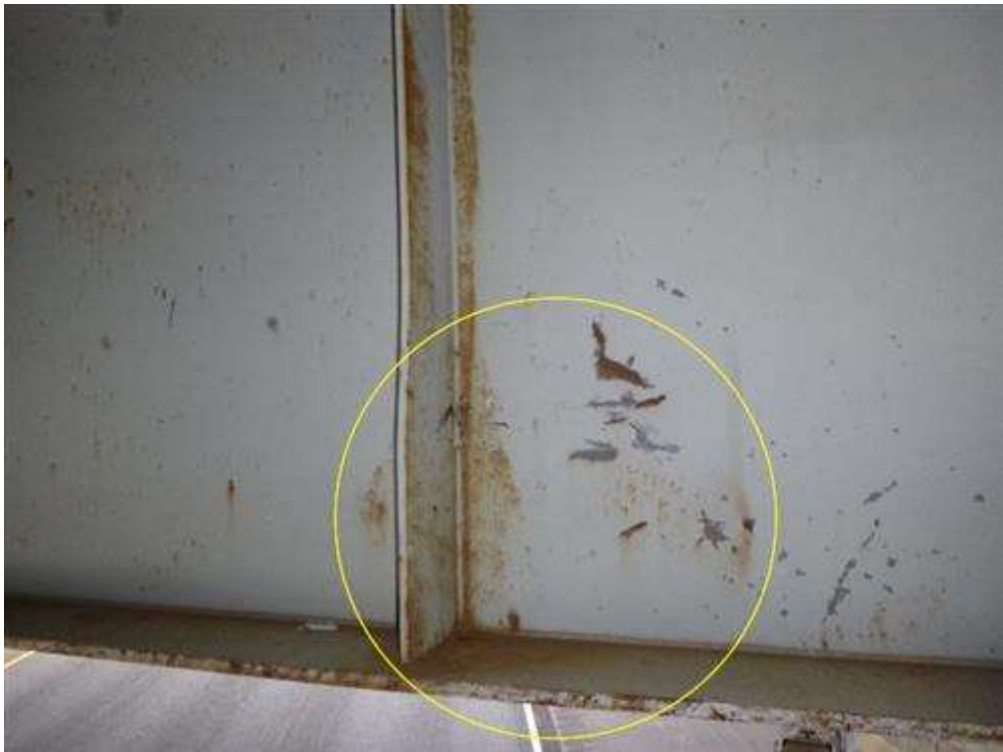
Span 1, girder 1 underside of bottom flange at the collision damage.
