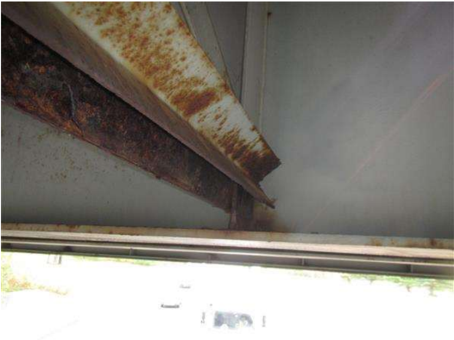
Span 1, bay 5, third intermediate diaphragm: Deformed/bent lower members and broken overhead welds due to impacted rust (rust removed).
