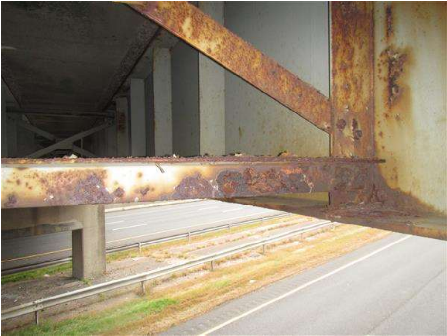
Span 2, bay 1, 4th diaphragm with a rusted through hole in the lower angle.
