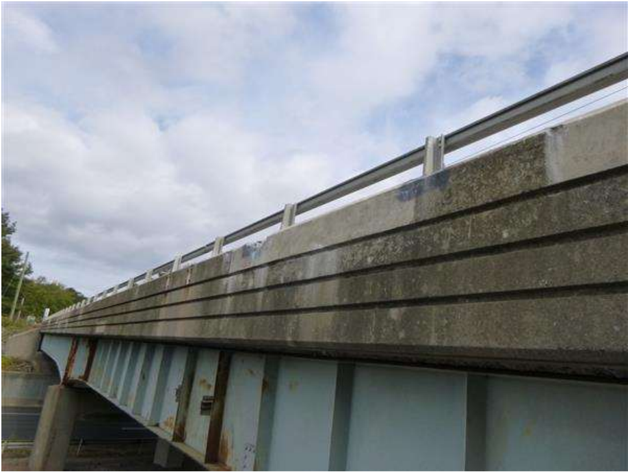
Span 1, west parapet near abutment 1 with hollow area.
