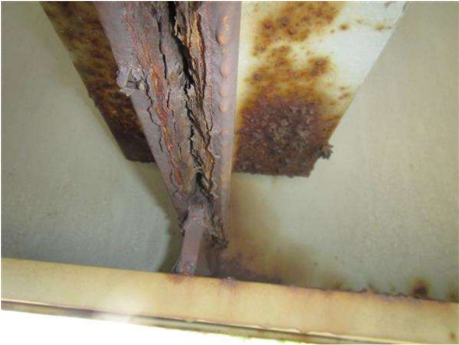
Typical impacted rust between lower intermediate diaphragm members. Also, note and broken overhead weld (typical condition).
