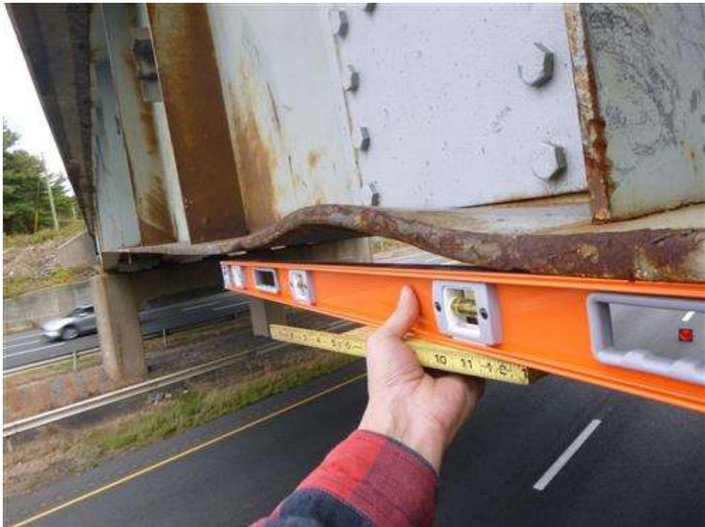
Span 1, girder 1 west elevation web with repair plate at the collision damage.
