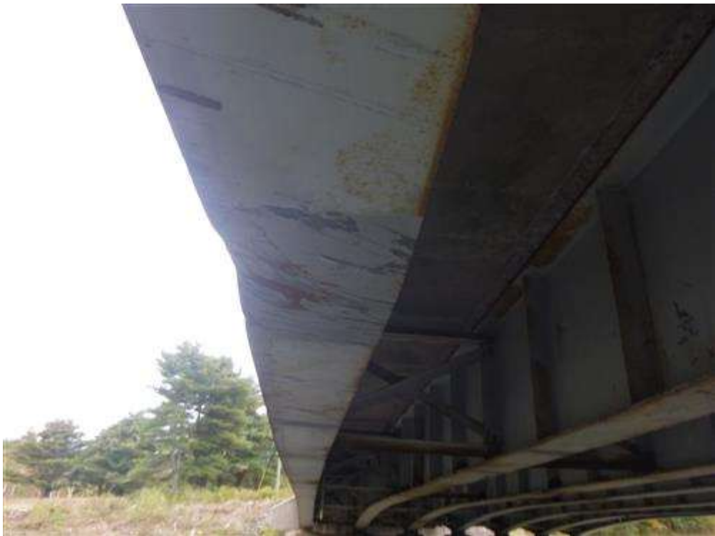
Span 1, girder 1 underside of bottom flange at the collision damage.
