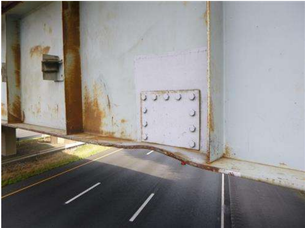
Span 1, girder 1 west elevation web with repair plate at the collision damage.
