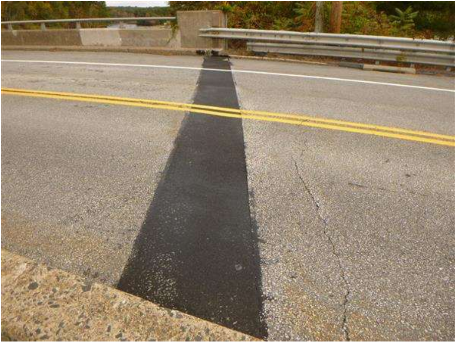
Asphaltic plug joint at abutment 1, looking east. Note the adhesion crack.
