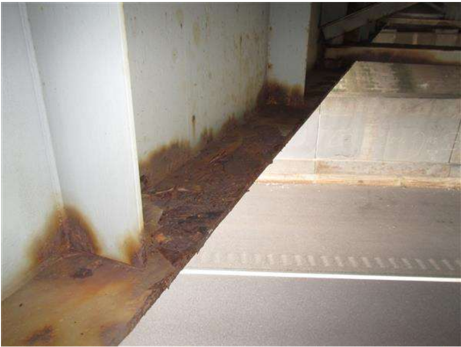
Span 2, girder 2, east elevation at panel 4: Laminated rust and section loss at bottom flange.
