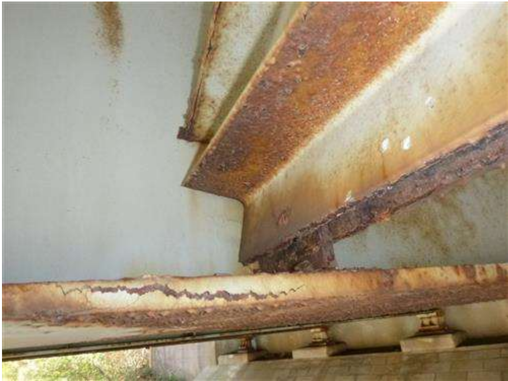
Photo Number: 27 Span 1, bay 2, first intermediate diaphragm. Note deformed/bent lower members and broken overhead welds due to pack rust. Photo Taken: 10/17/2023
