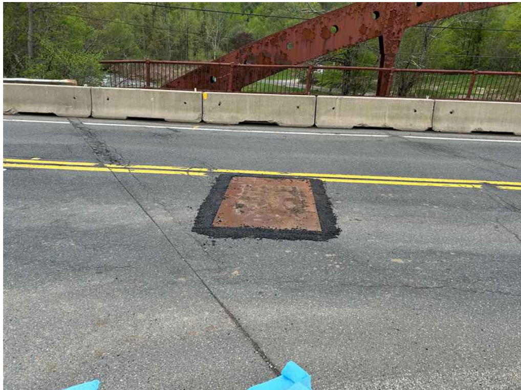
Photo 2: Steel plate installed at the east end, in the westbound lane, looking south.
