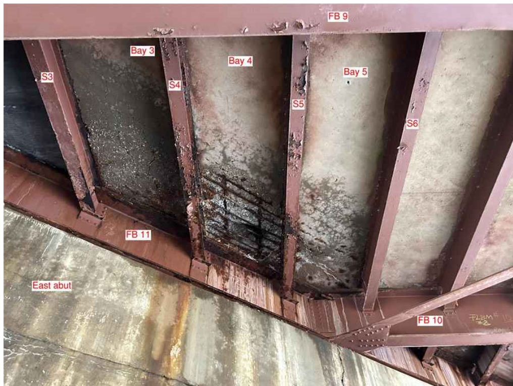
Photo 4: Deck underside at the east end of panel 9. Note the full width through spall in bay 4, and the cracking, efflorescence, and leakage in adjacent bays 3 & 5.
