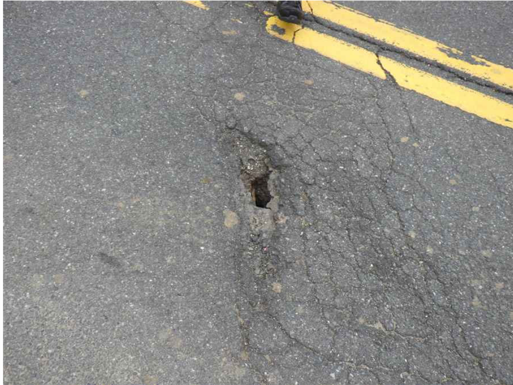
Photo 1: Full depth hole at the east end of the wearing surface and concrete deck, prior to steel plate installation.
