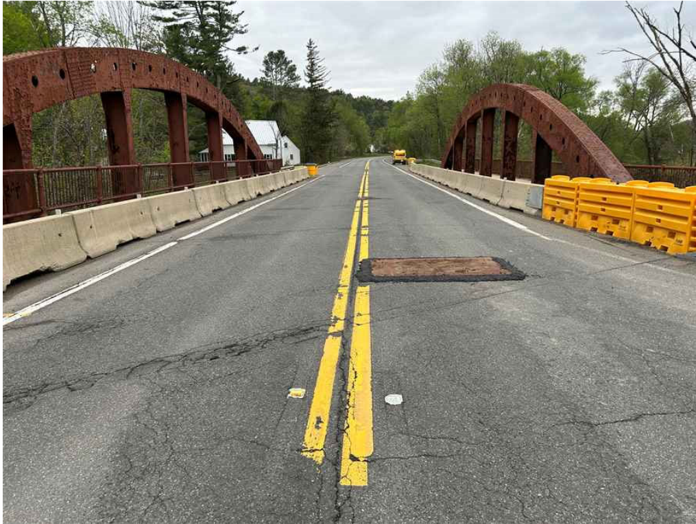
Photo 3: Steel plate installed at the east end, in the westbound lane, looking west.
