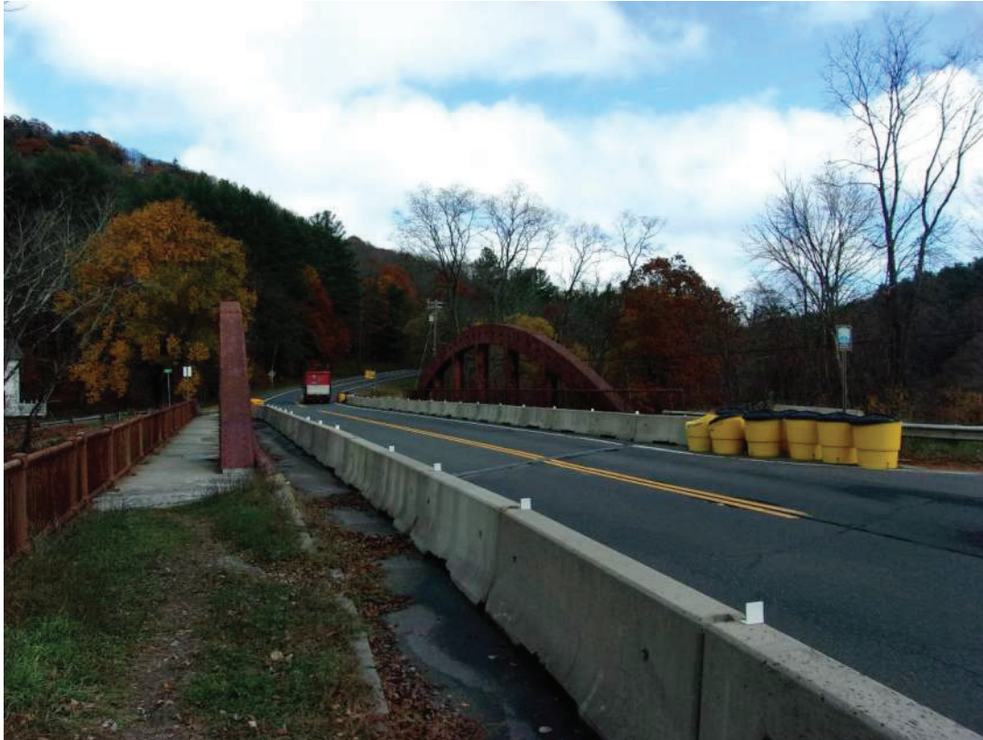
5. West Approach Looking East (Note North Sidewalk Lacking Connection Point)
