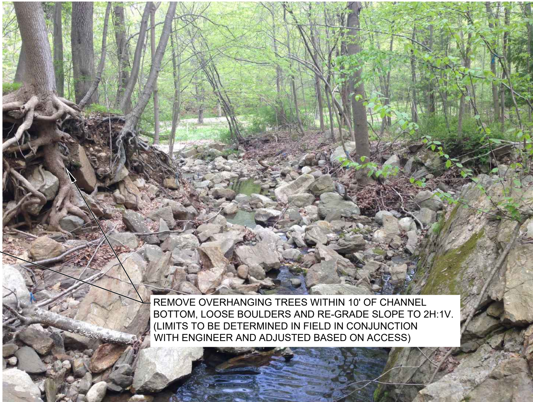
1B AUXILIARY SPILLWAY CHANNEL IMPROVEMENTS - LOOKING DOWNSTREAM
