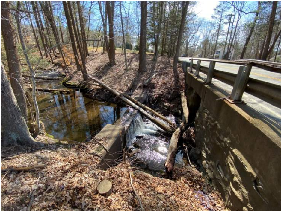
Photo 4 – East (upstream) side of bridge and abutments. Note small dam present upstream.
