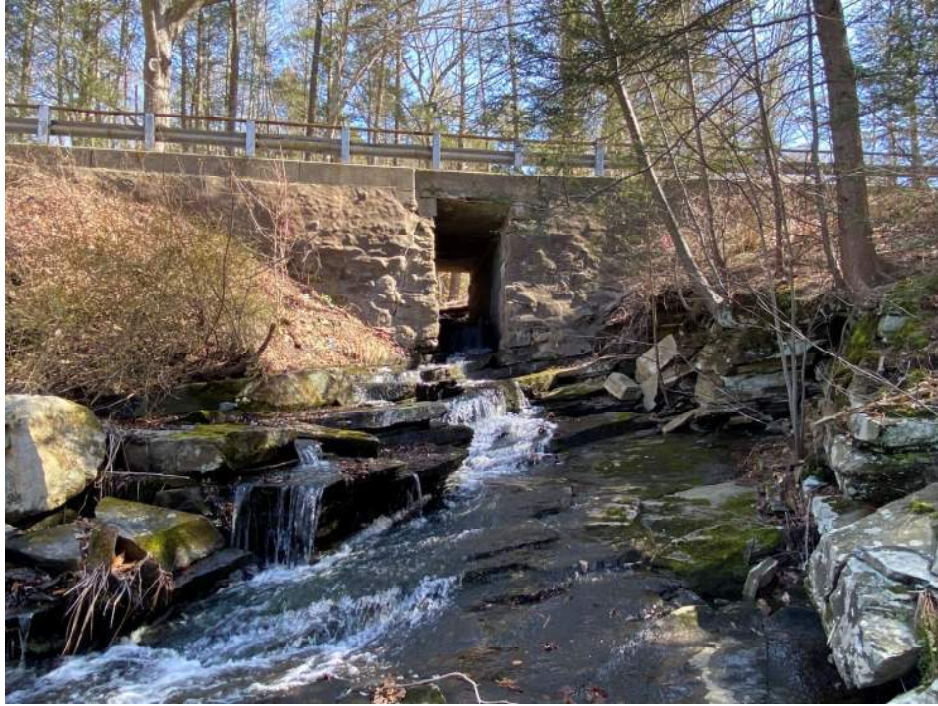
Photo 3 – View of west side wing walls and abutments from downstream. Note bedrock controlled streambed.
