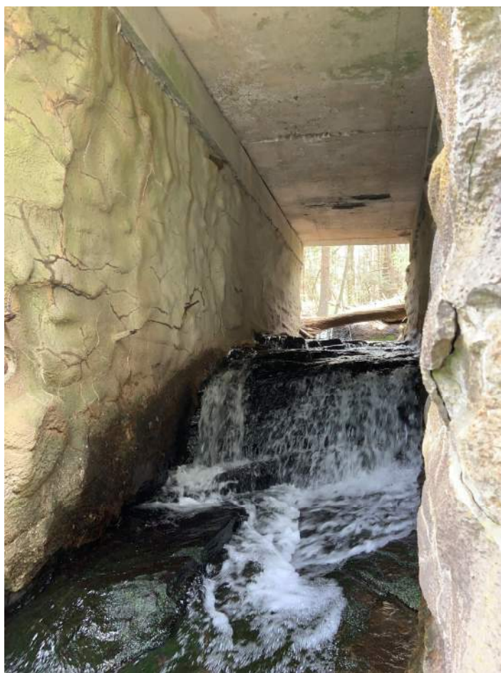
Photo 5 – Steep gradient bedrock streambed beneath the bridge.
