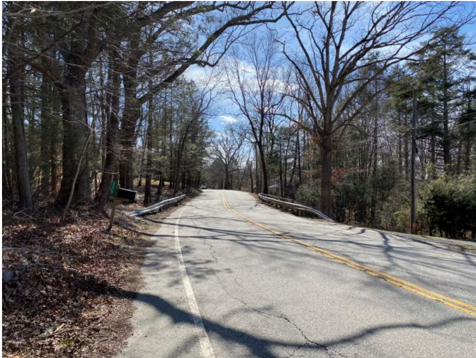
Photo 1 – Route 149 looking south over Bridge No. 02698.
