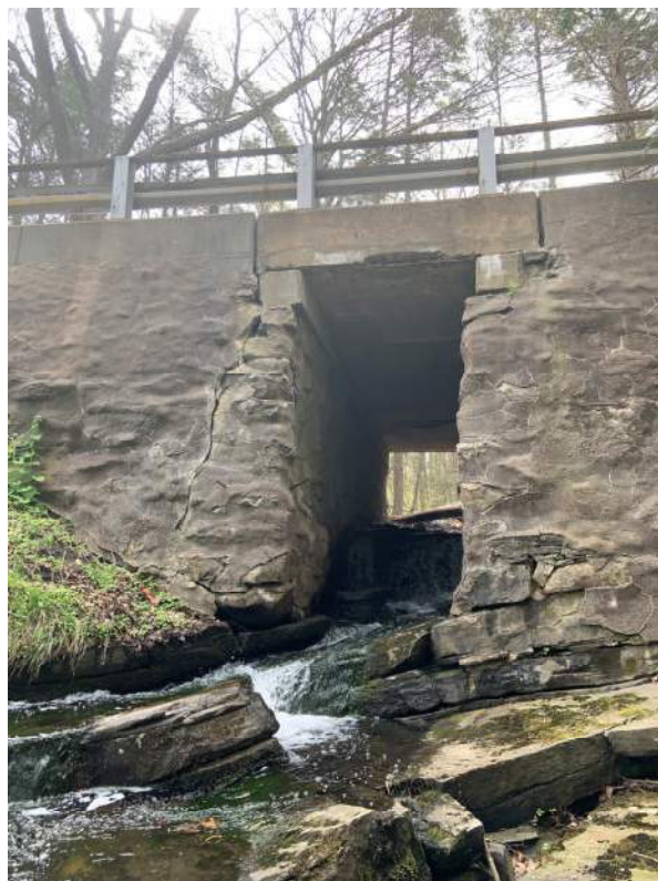
Photo 2 – Close up view of west side wing walls and abutments.
