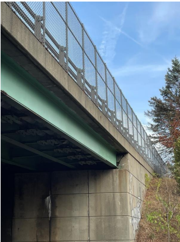
Figure 2. Metal guardrails and chain-link fencing on Bridge M-06-010 over I-495
