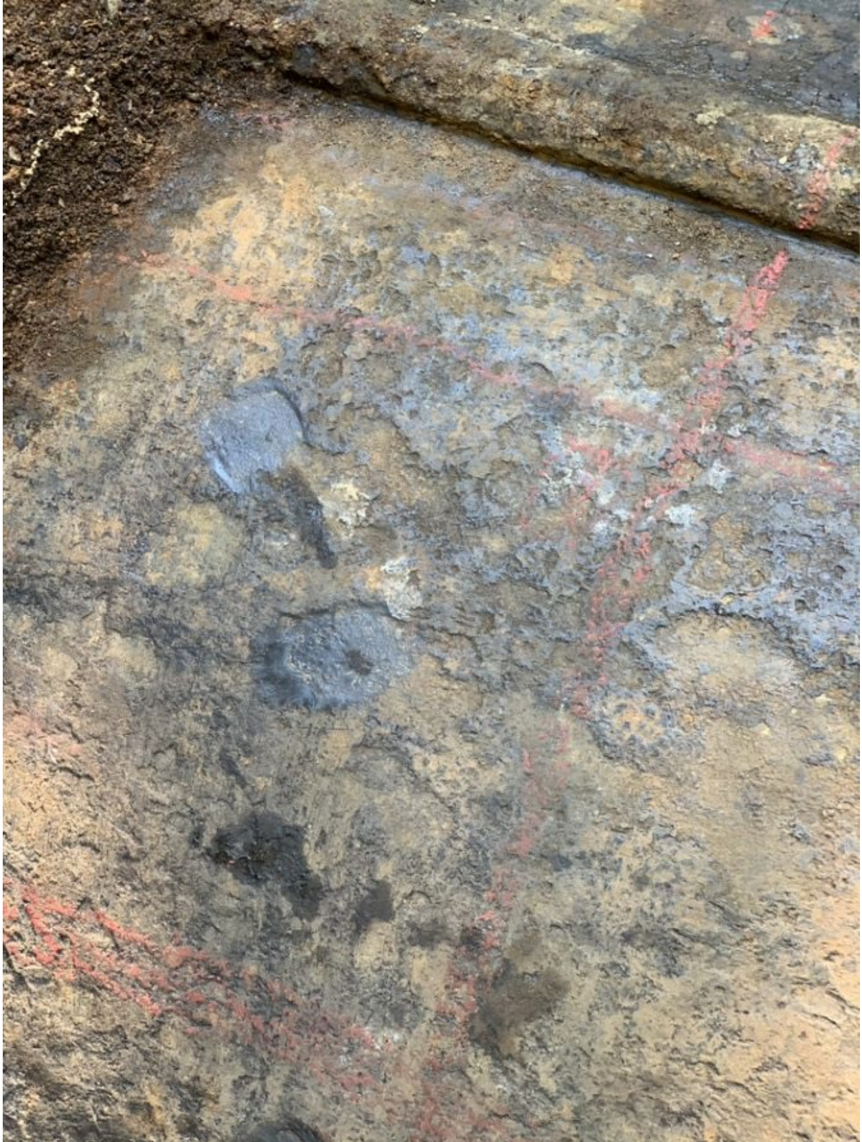
Site #3: Waverly Oaks Road: Coating De-lamination
