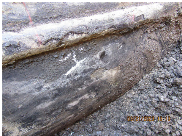
6 – Site 1 Spring line and lock bar
