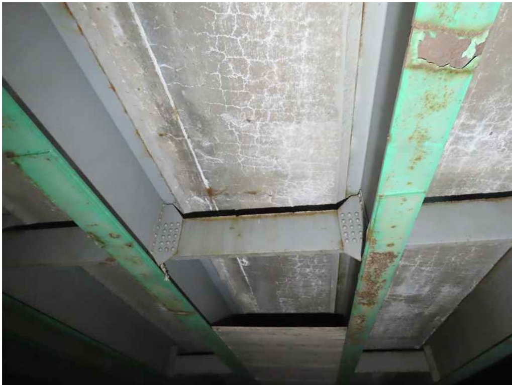
Photo 2: Span 2 bay 6 cold joint.
