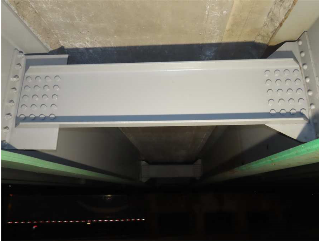
Photo 9: Span 3 bay 6 2nd diaphragm from pier 3 repair.
