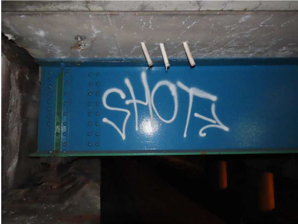
Photo 7: Typical deck weep condition. Northwest corner shown.
