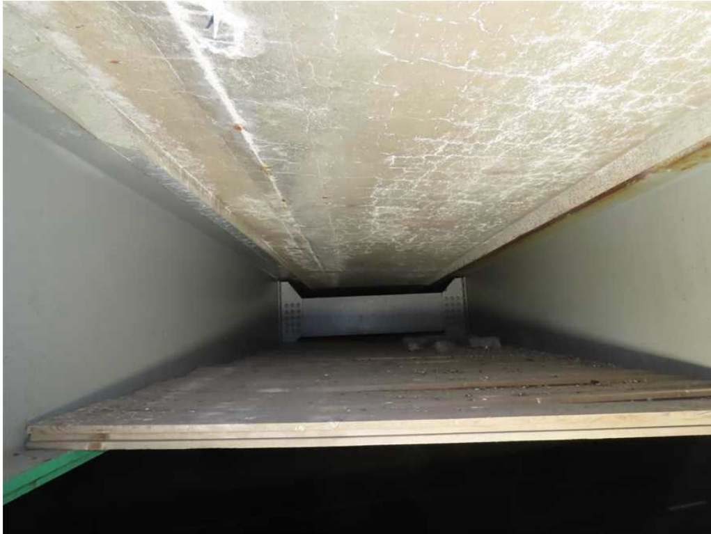
Photo 3: Span 2 bay 6, spalled haunch of timber shielding.
