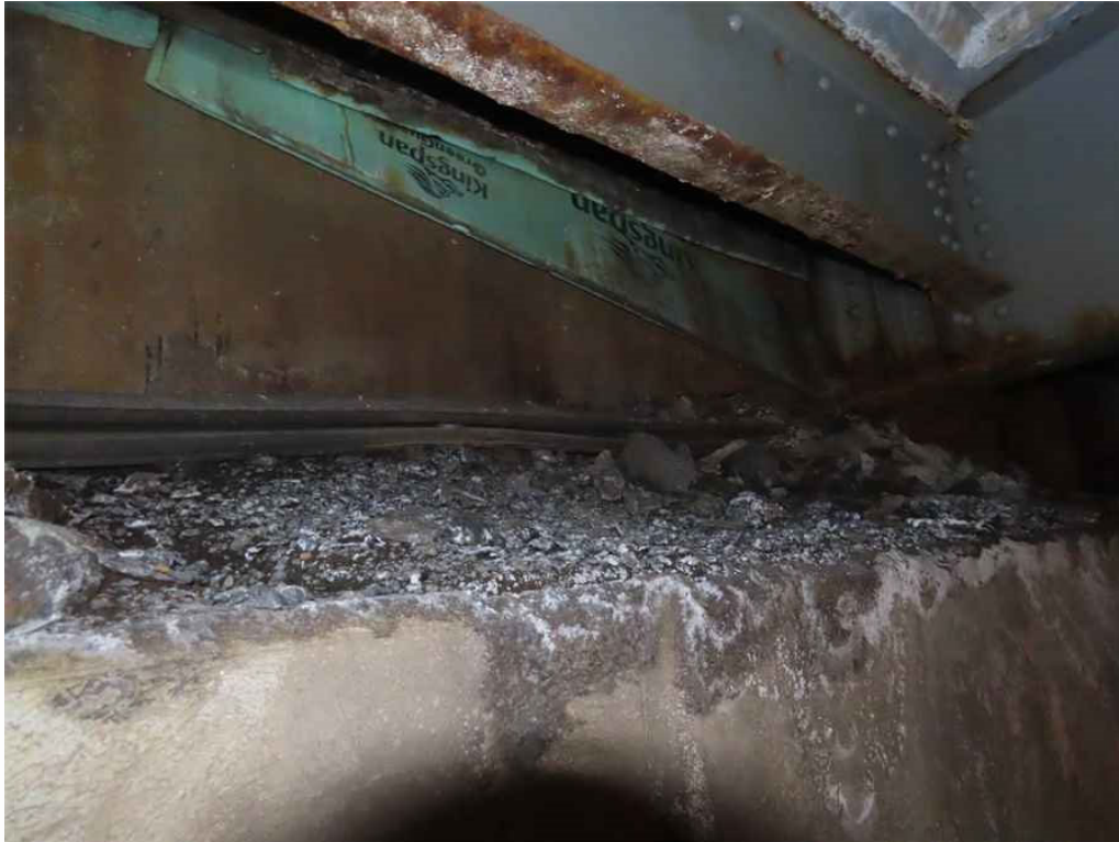
Photo 15: North abutment, bay 6 debris accumulation
