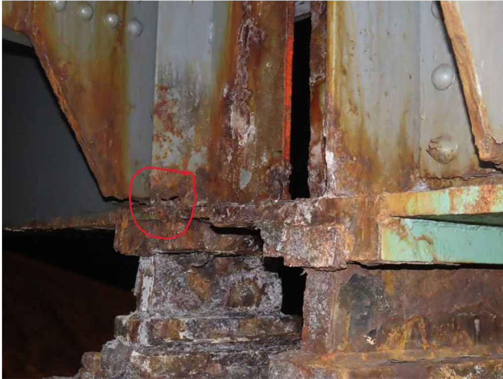
Photo 13: Beam 24 at pier 3, 100% section loss to stiffener.
