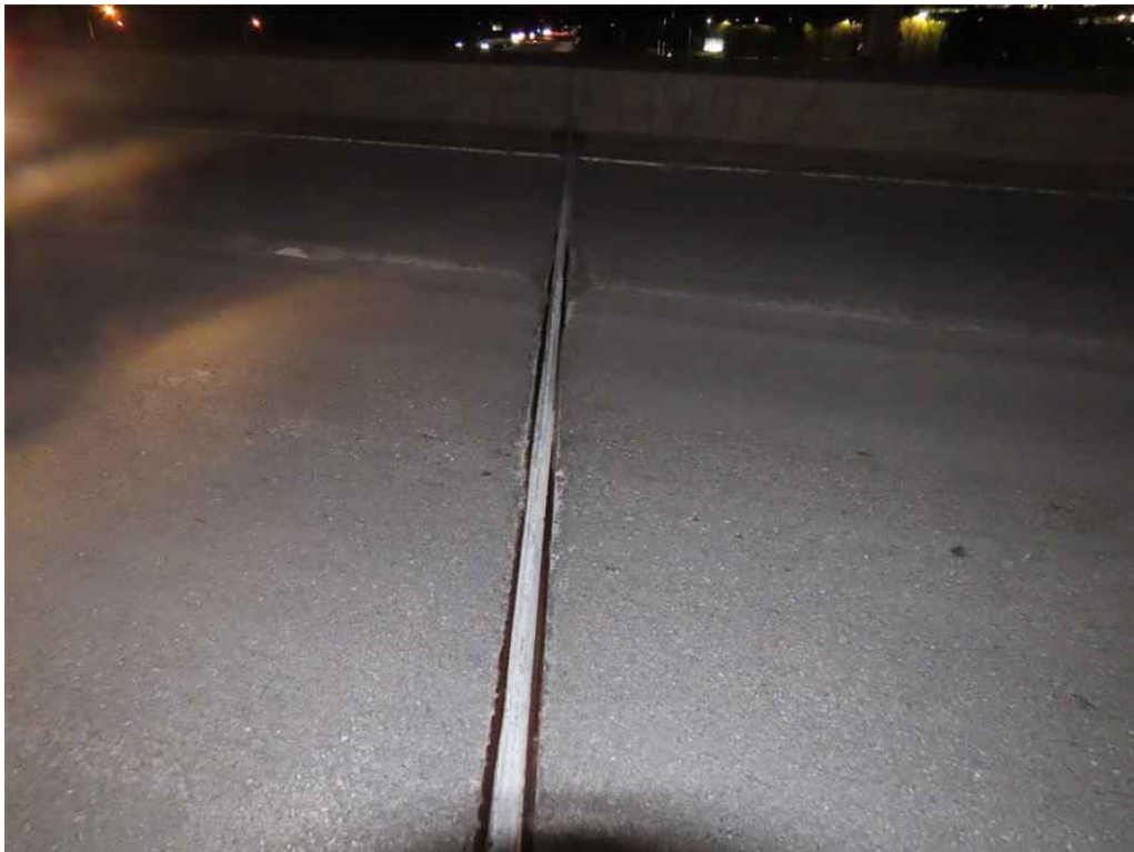
Photo 6: South deck joint.
