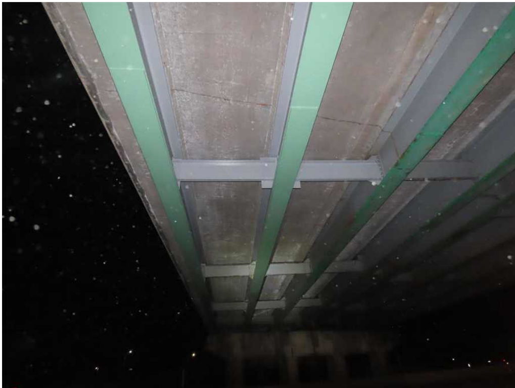
Photo 8: Span 3 beams 23-24 and diaphragm repairs.
