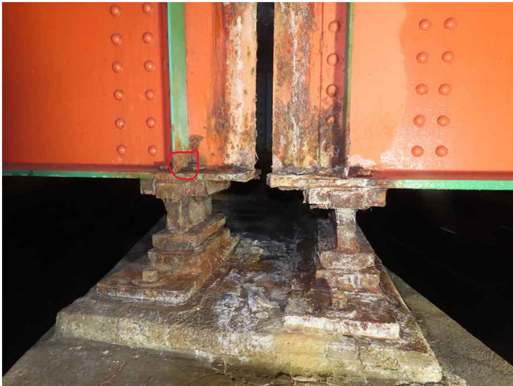
Photo 14: Beam 16 and 24 at pier 2. Note 100% section loss area to beam 16.
