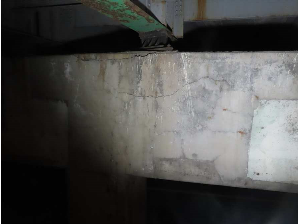
Photo 27: Typical delamination cracking in repaired areas. Pier 2 south face under beam 10.
