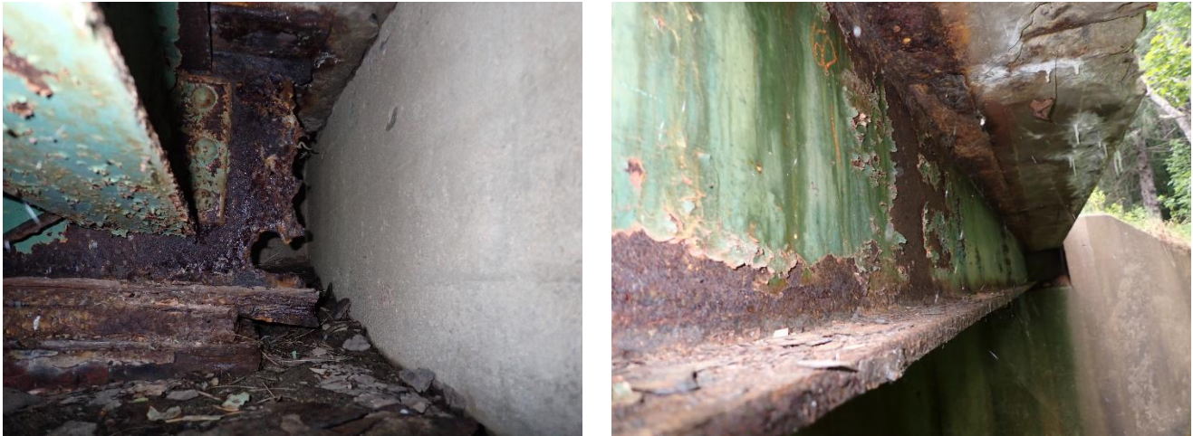
Figure 1: Severe Corrosion of Beam Ends
