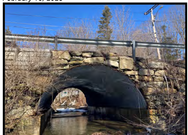
Photo 18: View facing upstream from the culvert outlet showing the decaying headwall. Photo taken February 15, 2023
