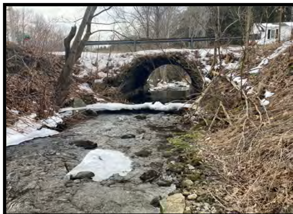
Photo 4: View facing downstream showing the culvert inlet. Note the stream downcutting and steep, eroding banks. Photo taken February 15, 2023
