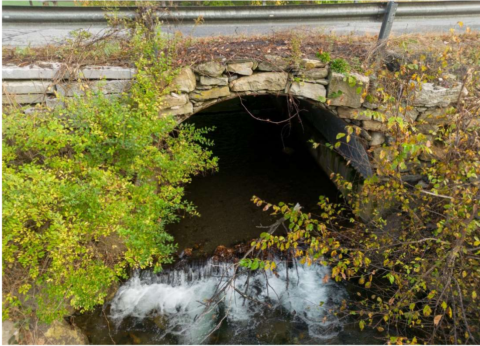
Photo 1: Existing Culvert Outlet
