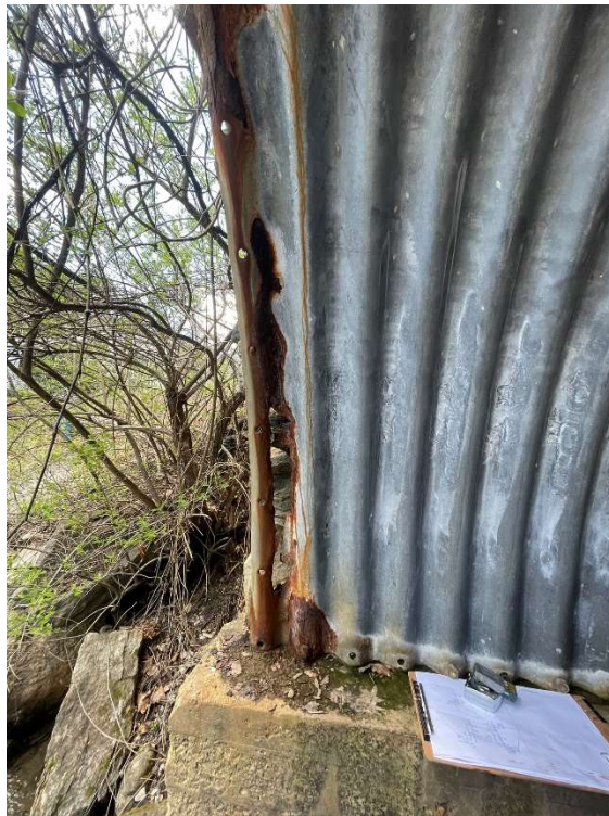
Photo 6: Deterioration on South End of Existing Culvert
