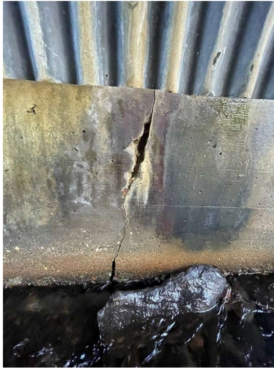
Photo 5: Spall in West Footing
