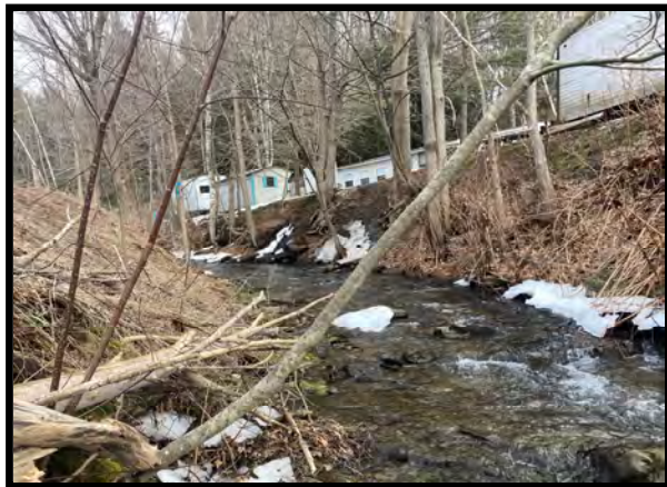
Photo 8: View facing upstream from the culvert inlet. Note the stream downcutting and eroding stream banks. Photo taken February 15, 2023
