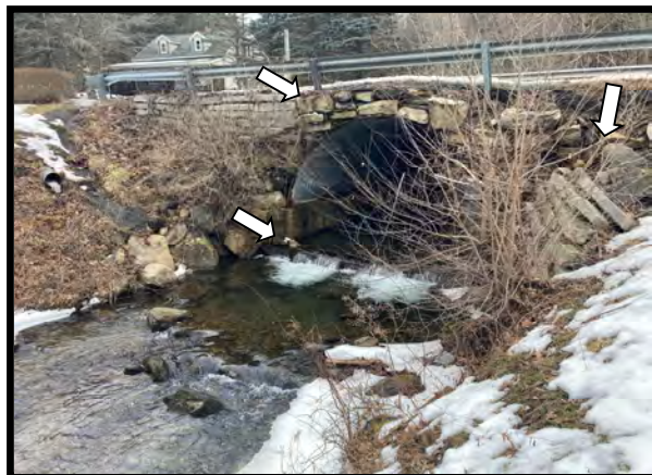
Photo 5: View facing upstream showing the culvert outfall. Note the berm at the outfall (arrow) and concrete debris on the left descending stream bank. Also, note the condition of the field stone headwall (arrow). Photo taken February 15, 2023
