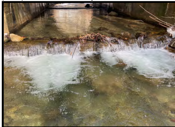
Photo 6: View facing upstream showing the elevational drop at the outfall, which has led to a 50-inch-deep scour pool. Photo taken February 15, 2023
