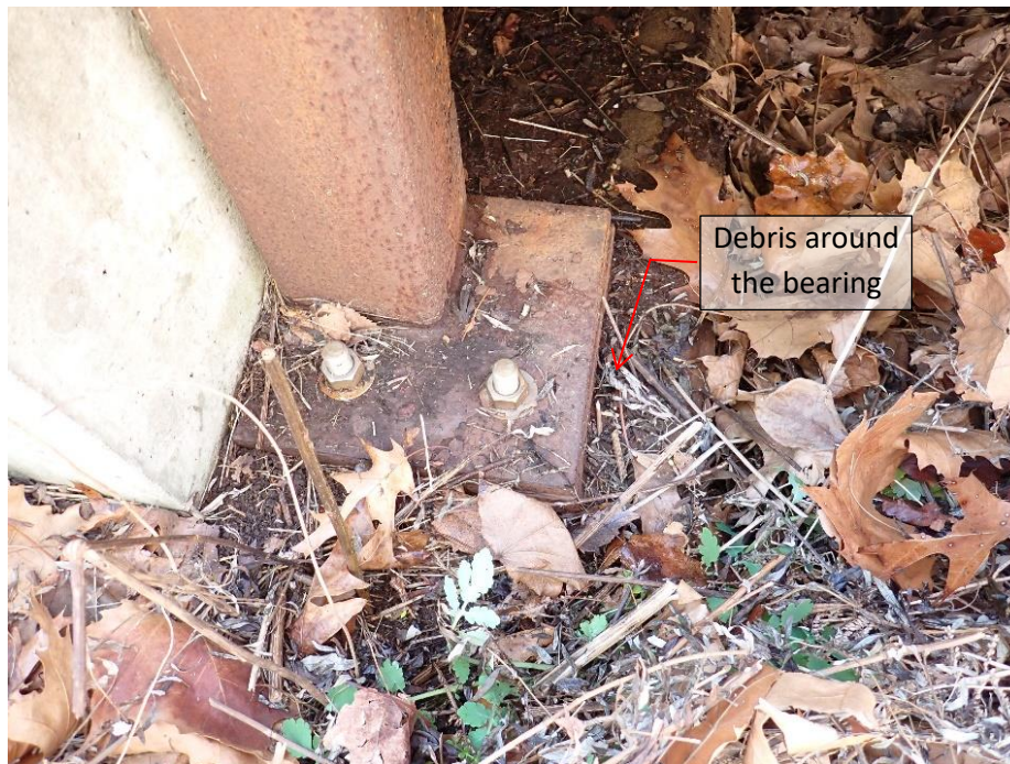
Bearing on North Abutment
