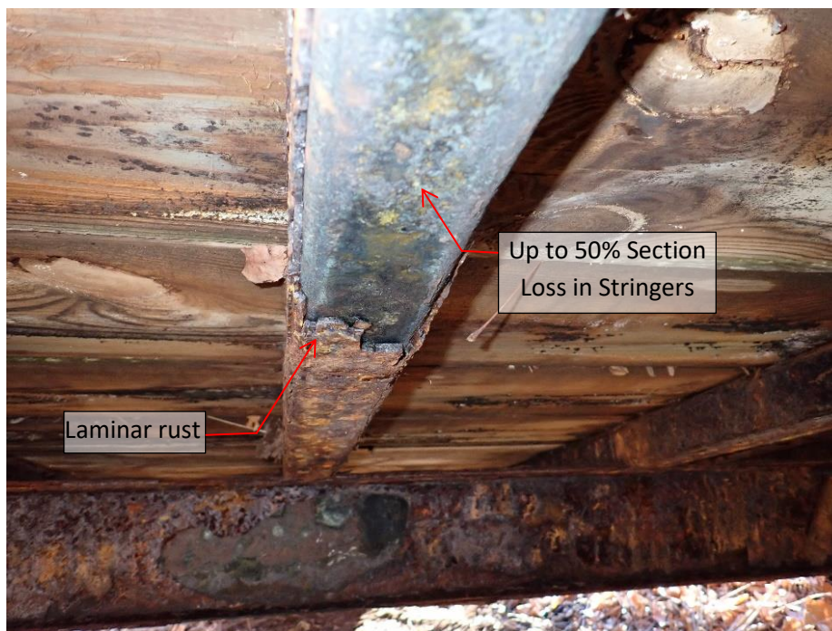
Section loss on steel sections
