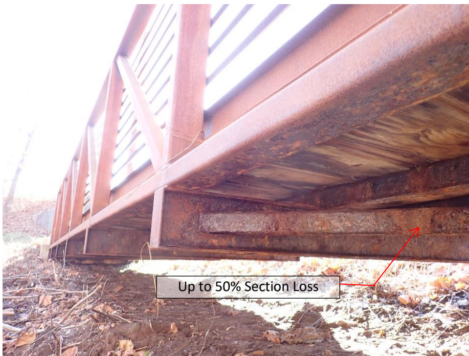
Section loss on steel sections
