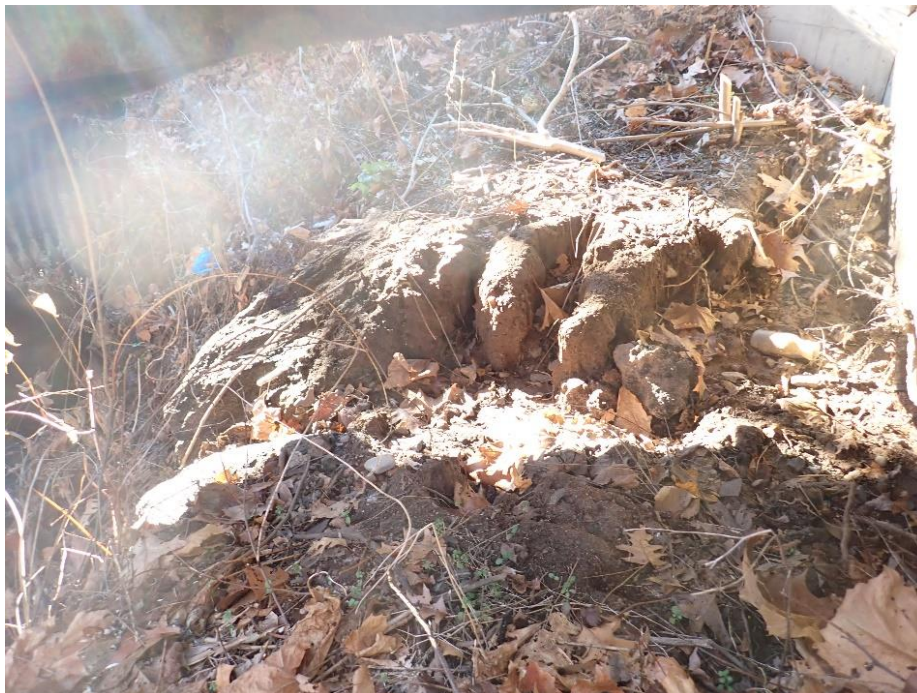
Evidence of erosion on Southern abutment
