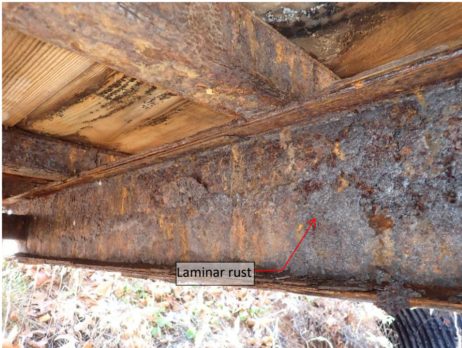
Section loss on steel sections
