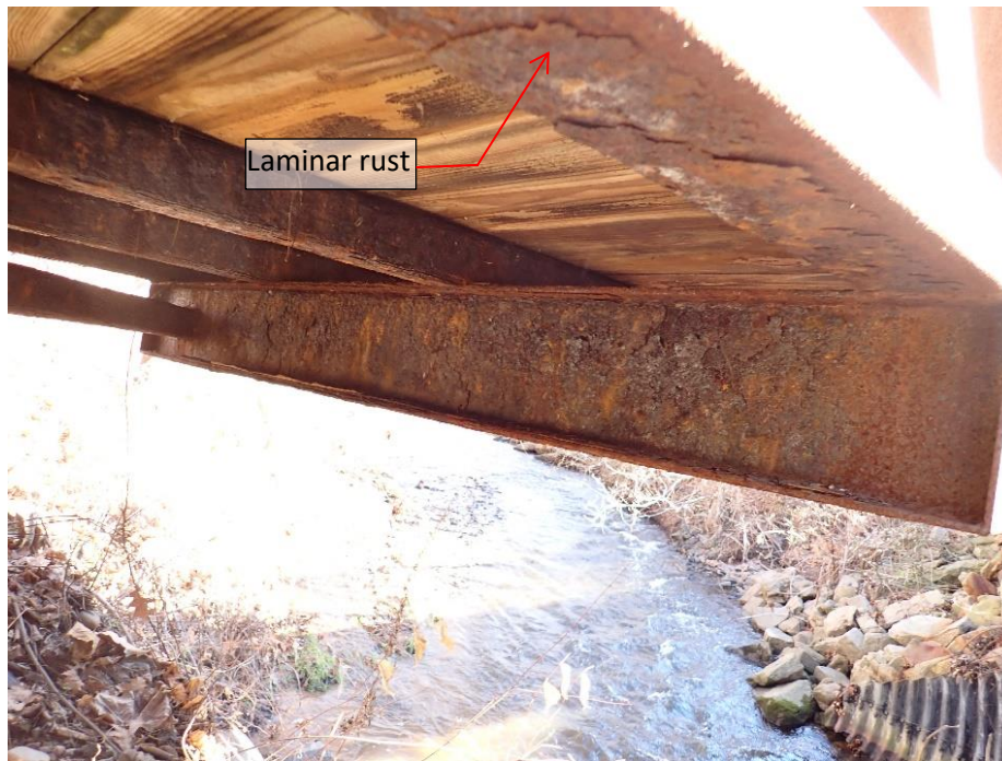
Section loss on steel sections
