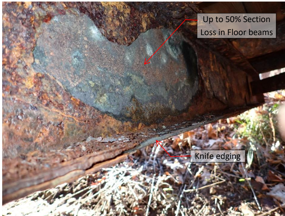
Section loss on steel sections
