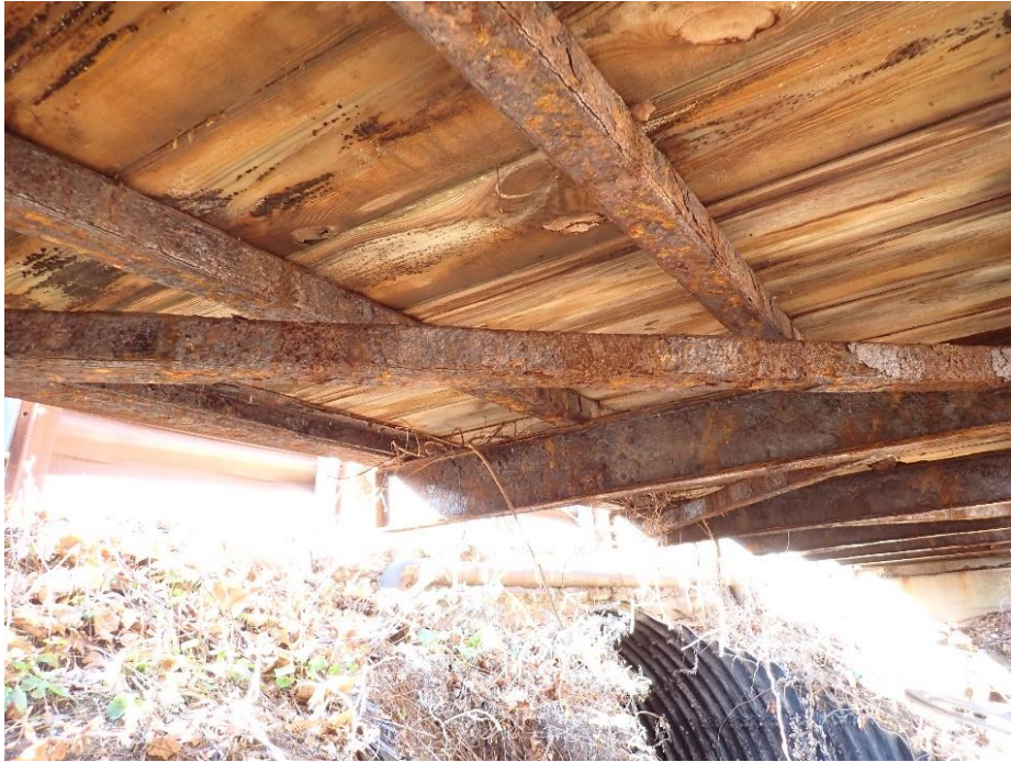
Section loss on steel sections
