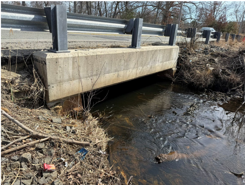
Figure B: Overview of the riverbed from the downstream side of the bridge (Maple Meadow Brook)
