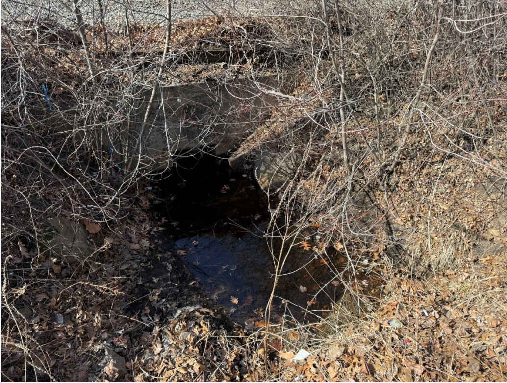
Figure C: Overview of the streambed at the Special Drainage Structure No. 1
