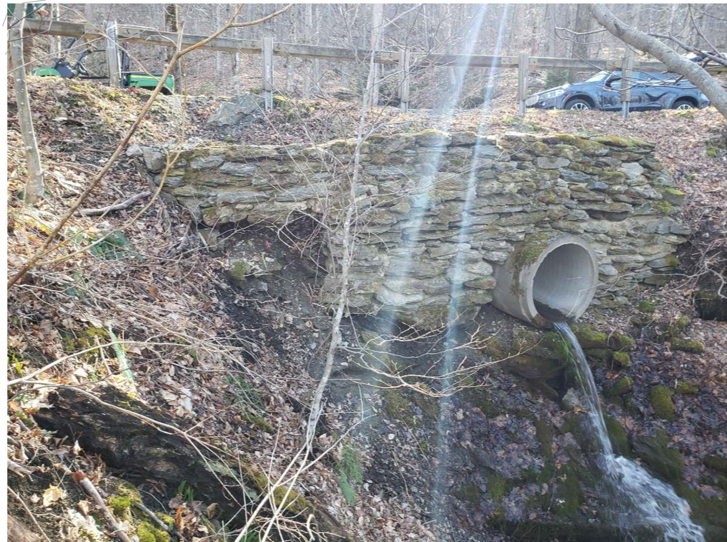
PHOTO 2 EXISTING CID 33 DOWNSTREAM HEADWALL
