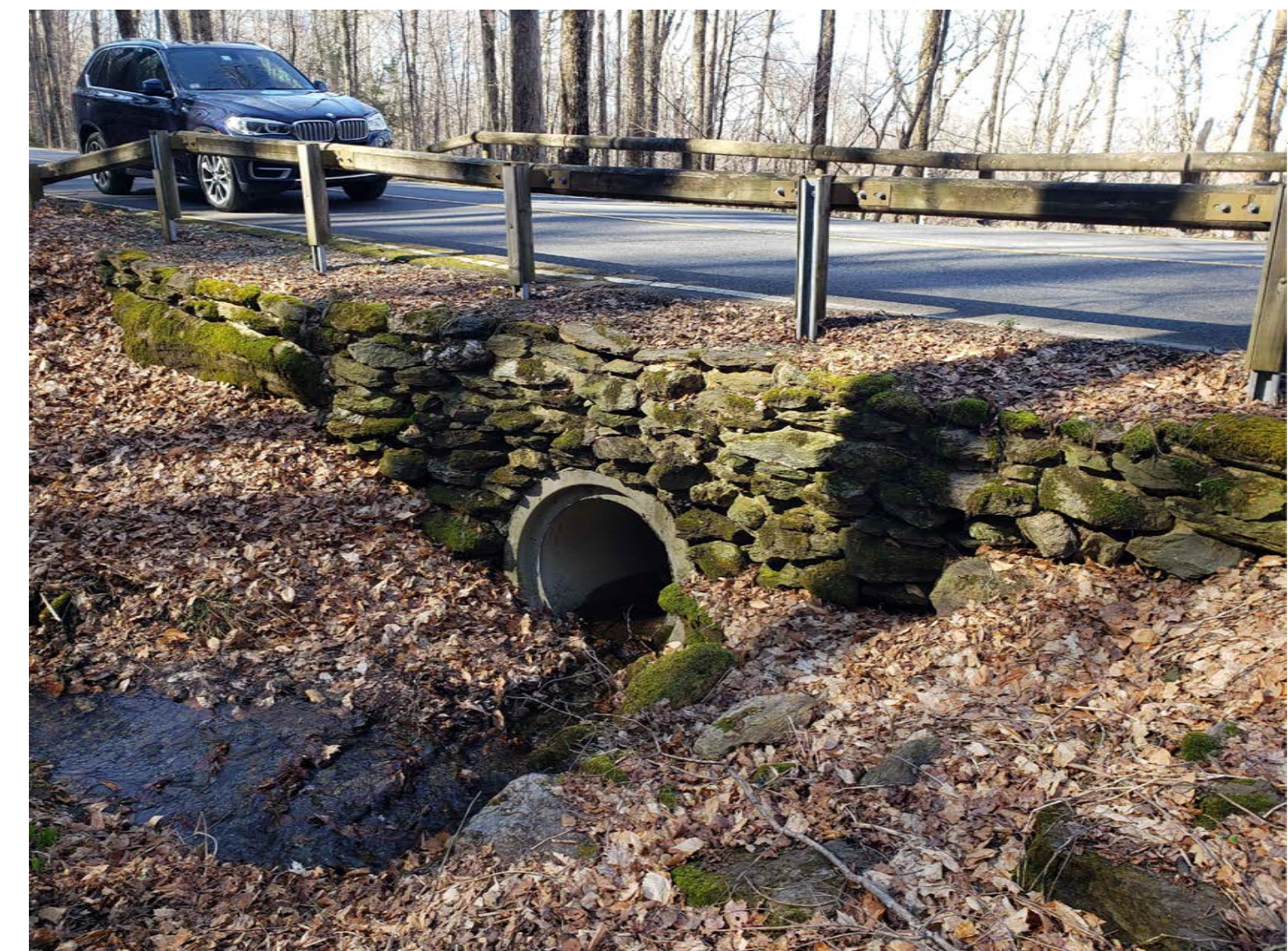
PHOTO 1 EXISTING CID 33 UPSTREAM HEADWALL
