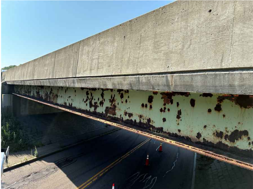
Photo 5: Beam 1 north fascia. Typical fascia condition.
