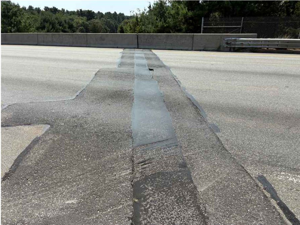
Photo 3: West asphaltic plug joint, looking south.
