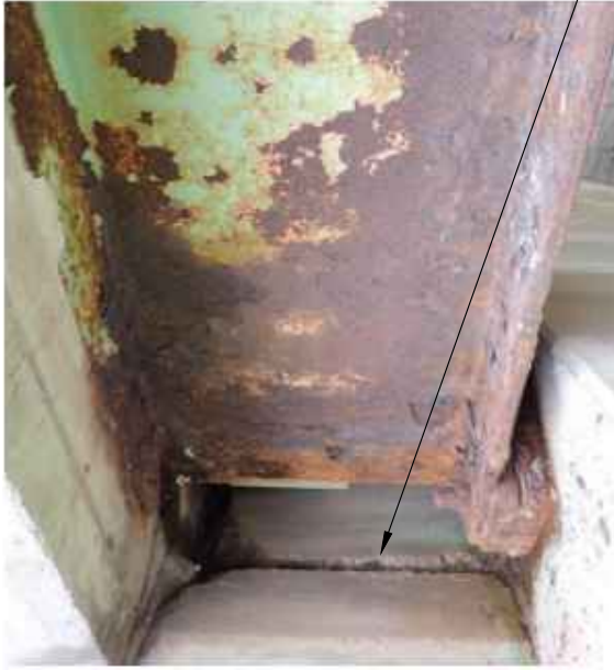
BEAM 1, EAST ABUTMENT, NB
