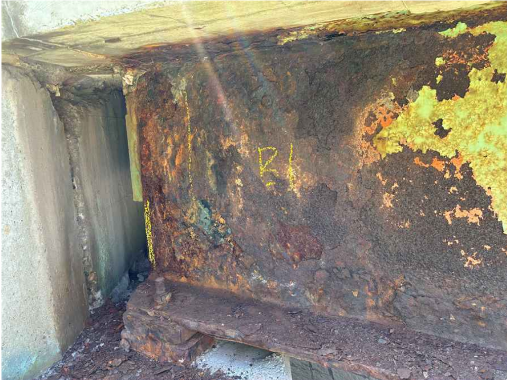
Photo 7: Beam 1 east end north face.
