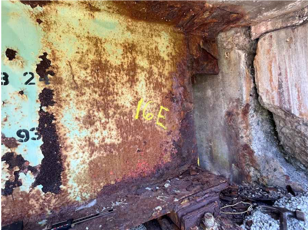
Photo 11: Beam #16, east end.
