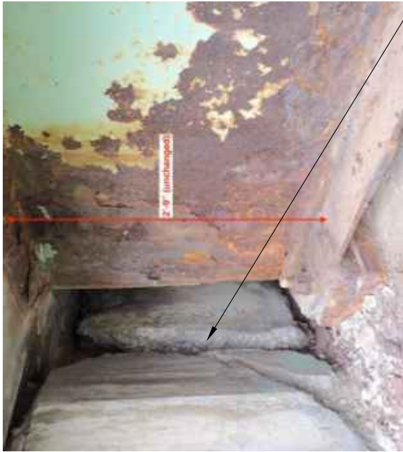
BEAM 1, WEST ABUTMENT, SB
