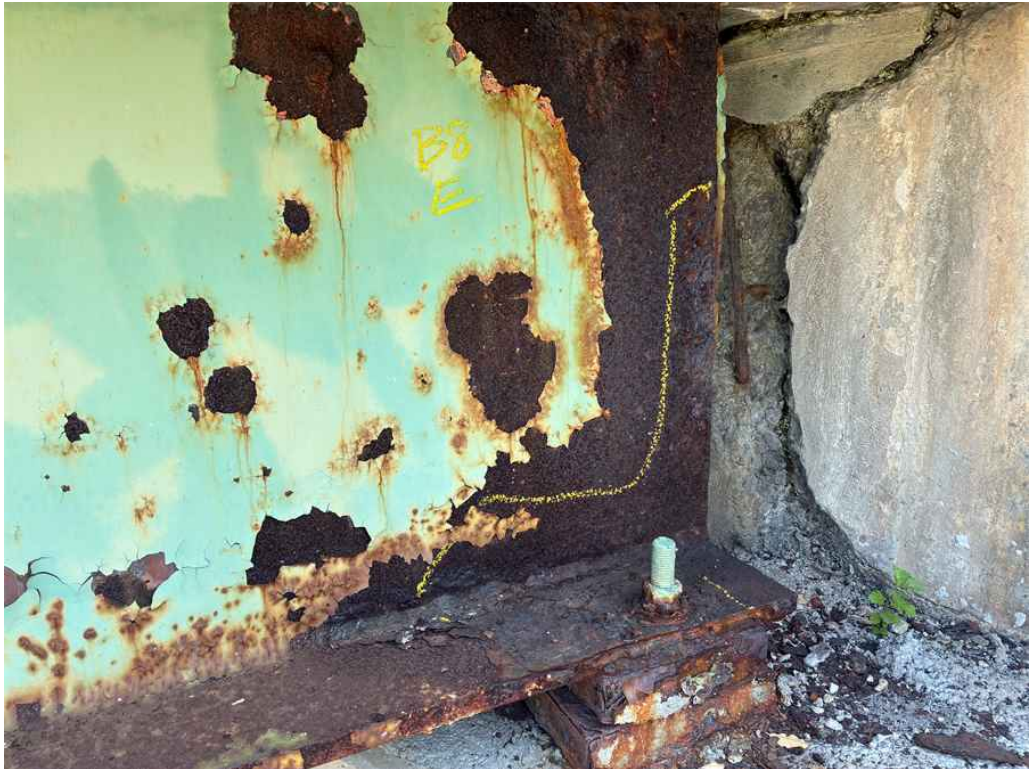
Photo 6: Beam 8 east end south face.
