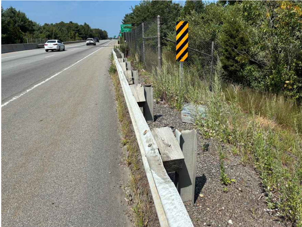
Photo 13: Northeast approach guardrail.
