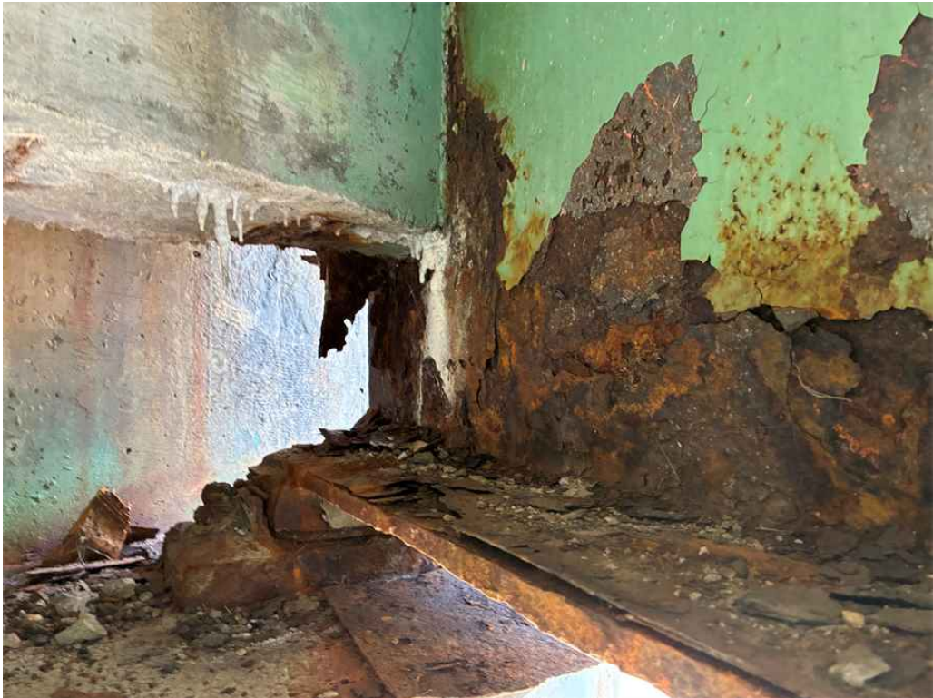
Photo 10: Beam 1 west end south face.
