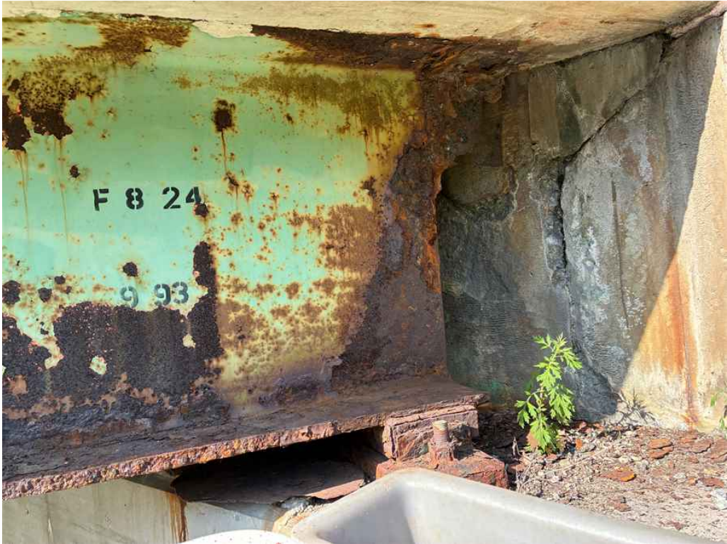
Photo 9: Beam 1 west end north face.
