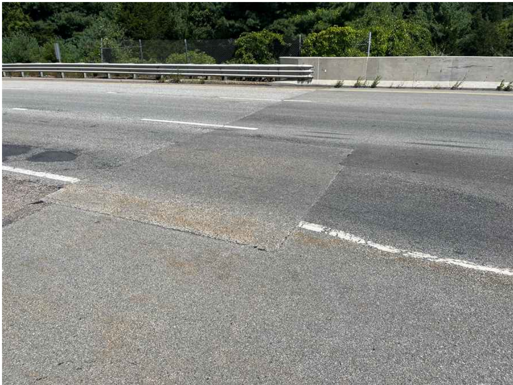
Photo 4: West approach pavement.
