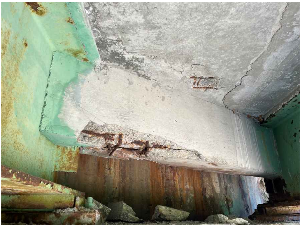
Photo 2: Bay #15, east deck end and diaphragm.
