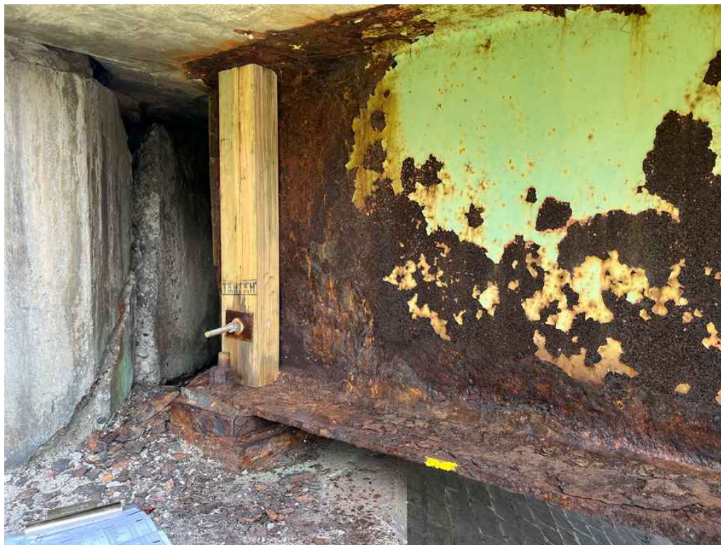
Photo 10: Beam #16, west end, south face.
