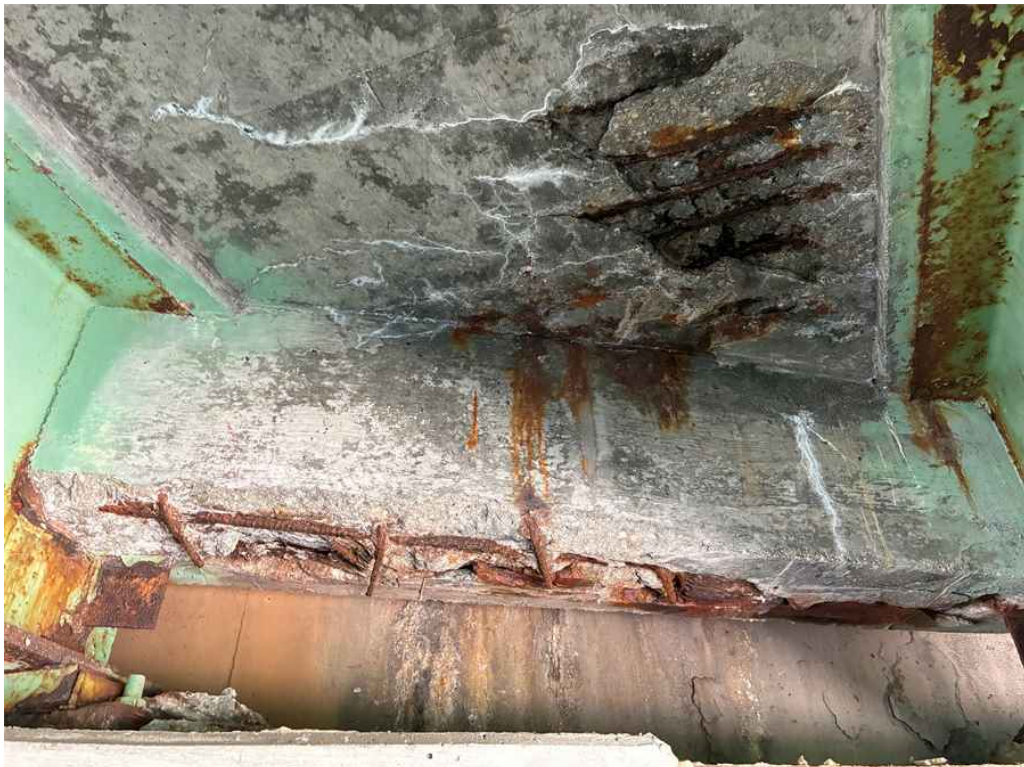
Photo 2: Bay 4 west end.
