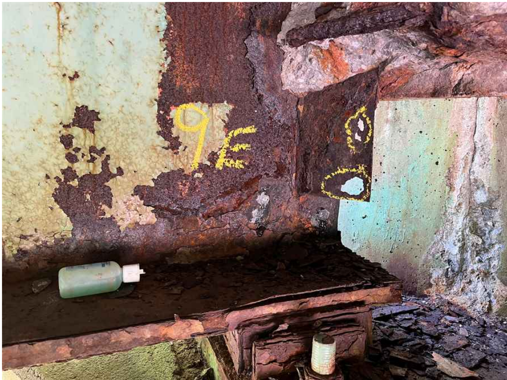
Photo 8: Beam #9, east end.
