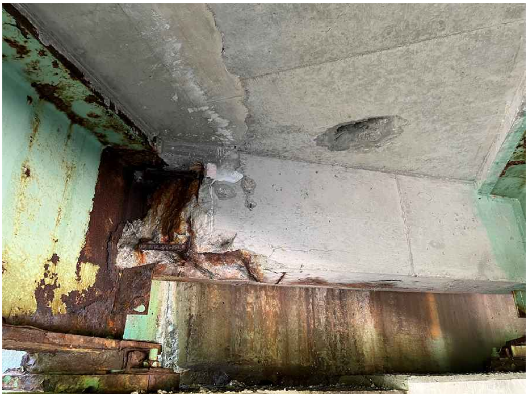
Photo 1: Bay #9, east deck end and diaphragm.
