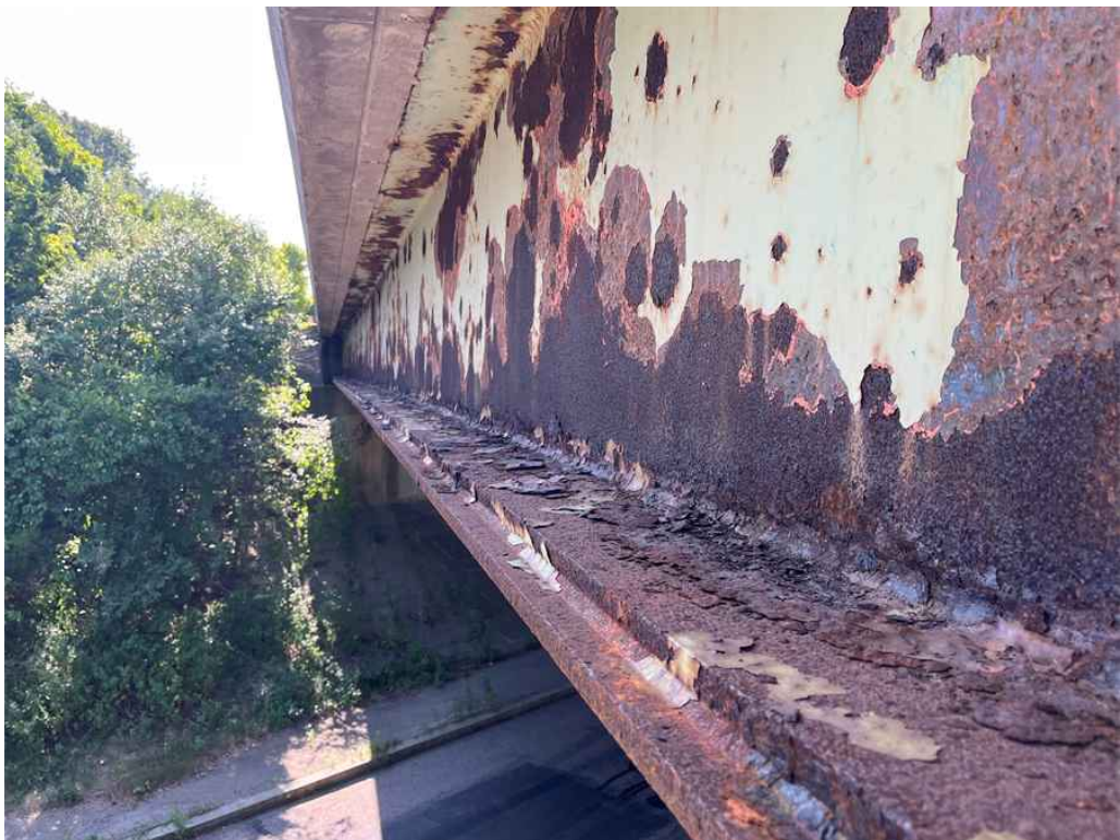
Photo 5: Typical fascia beam condition. Beam #9 looking east.
