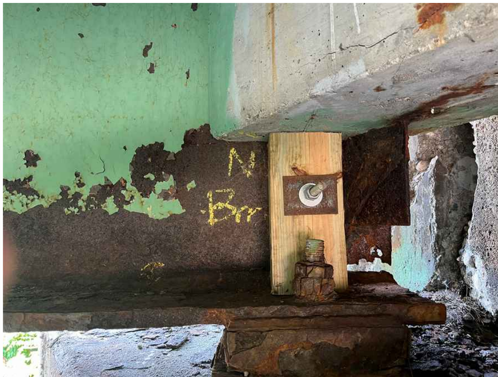
Photo 9: Beam #16, west end, north face.
