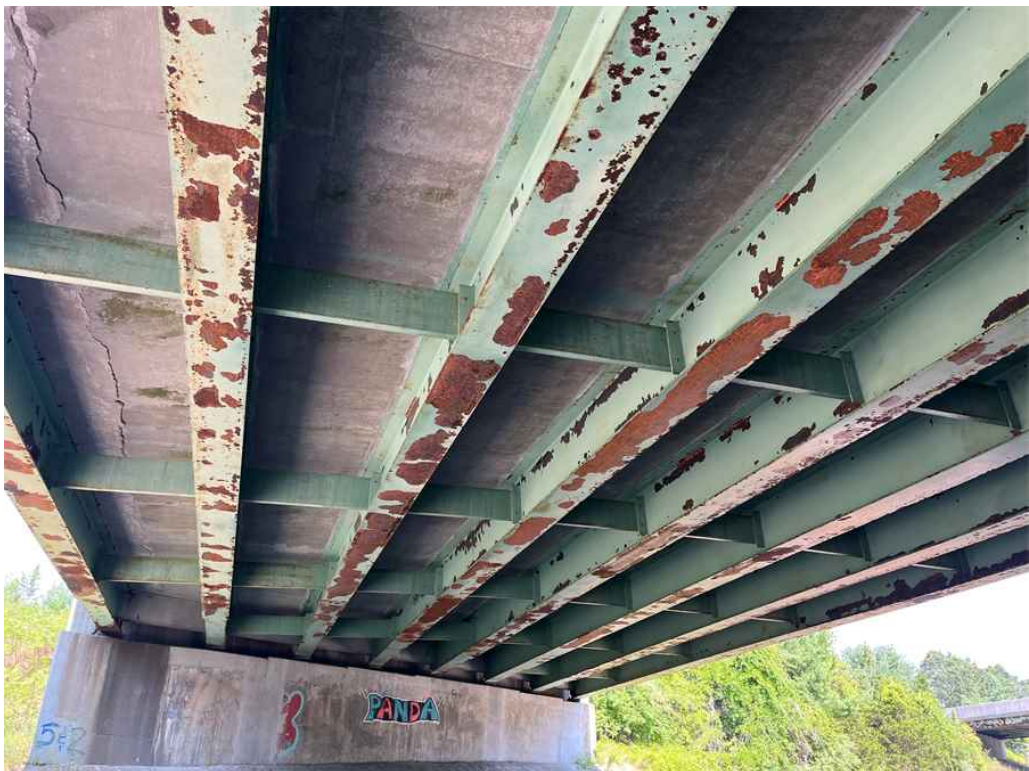
Photo 6: Typical interior beam condition. Looking west.
