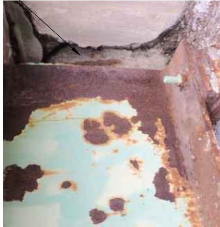
BEAM 8, EAST ABUTMENT, NB
