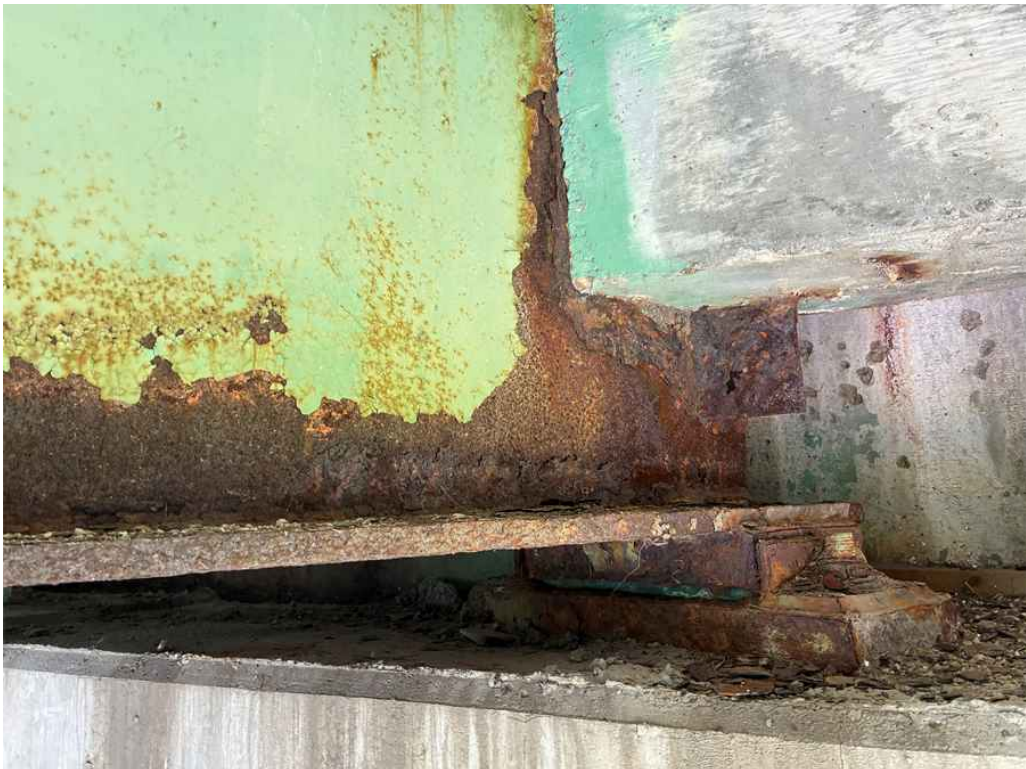
Photo 8: Beam 2 west end north face.
