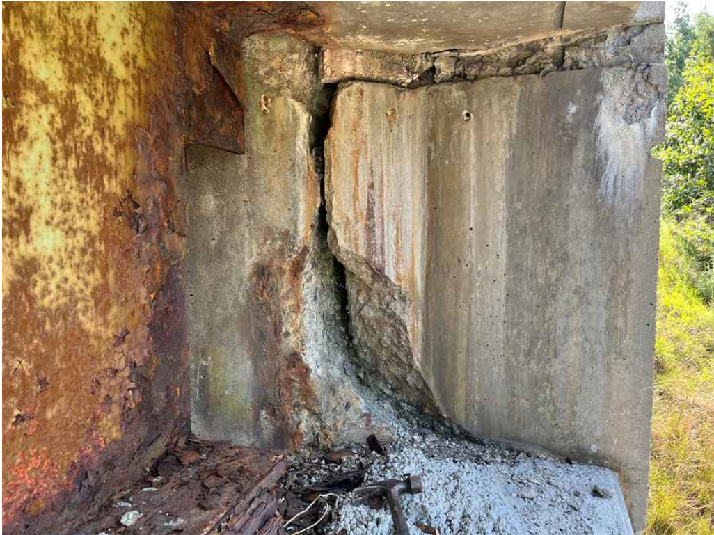
Photo 13: East backwall, south end.
