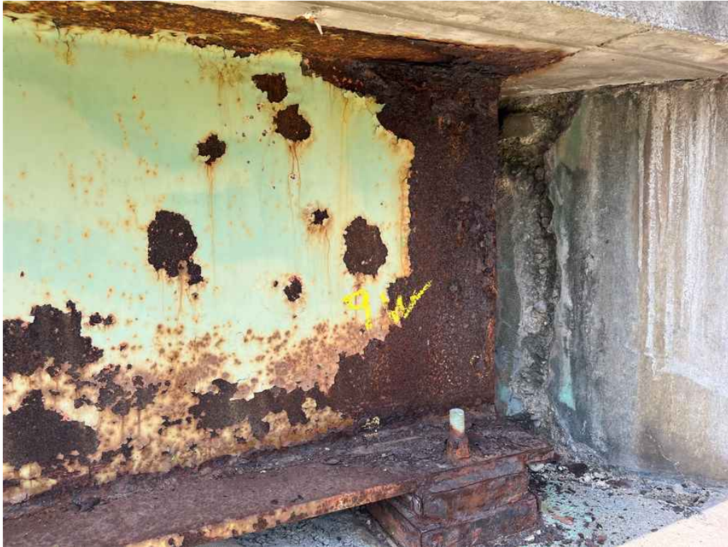
Photo 7: Beam #9, west end.
