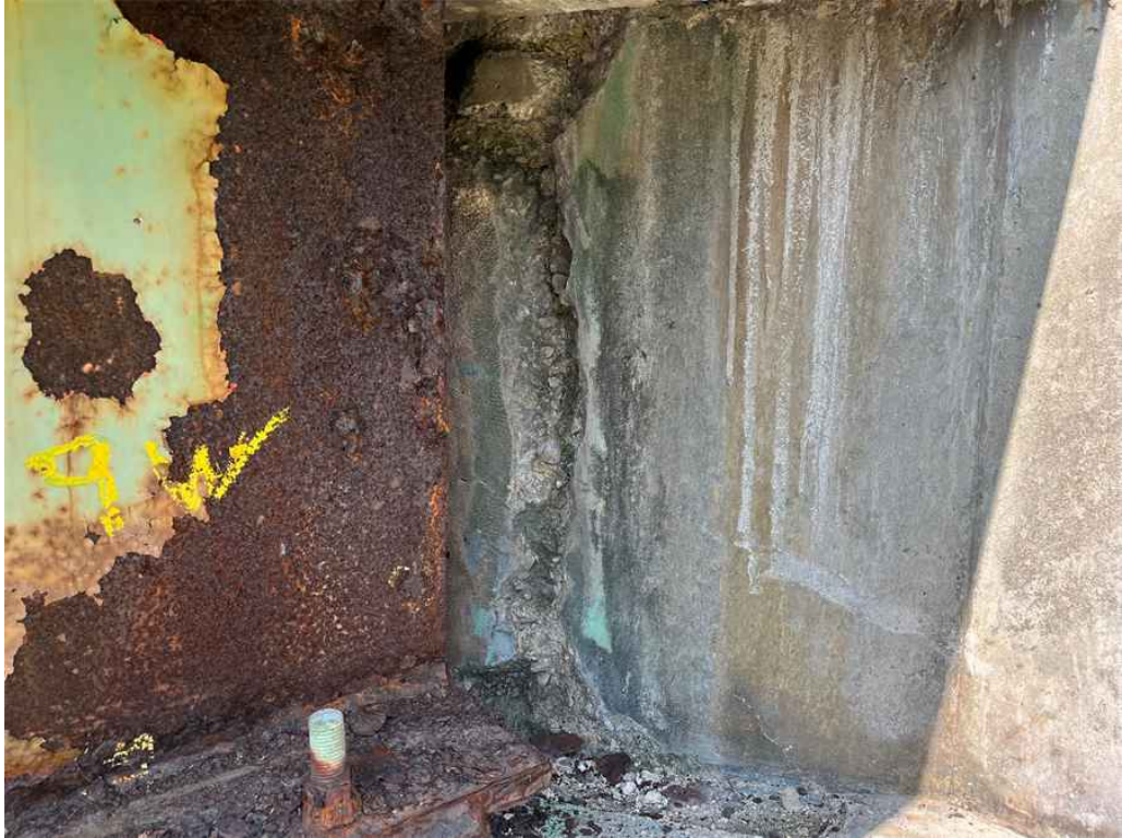
Photo 12: West backwall, north end.
