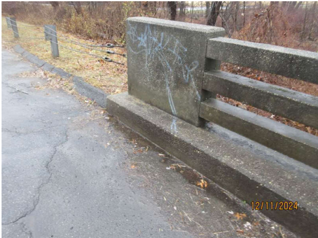
Photo 6: Northeast Concrete Endpost has been repaired.
