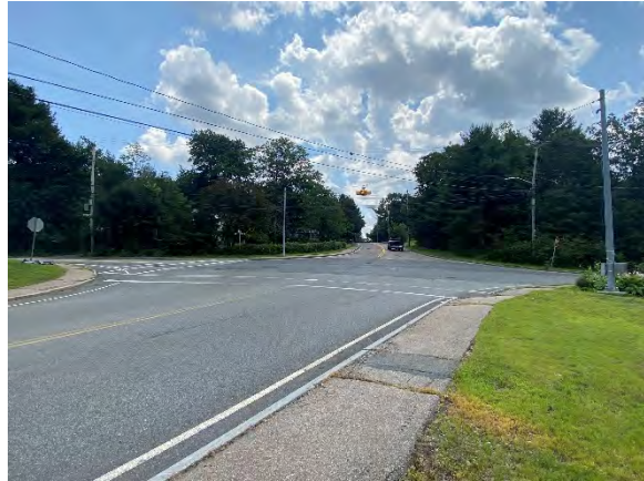
Photo 2: Hancock Street (Facing South)
