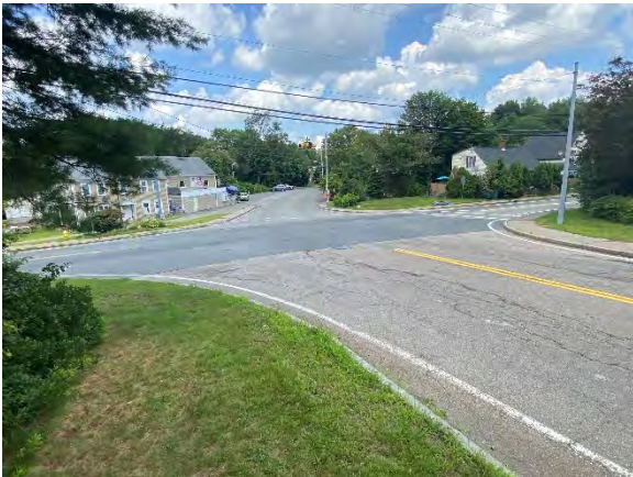
Photo 3: Hancock Street (Facing North)
