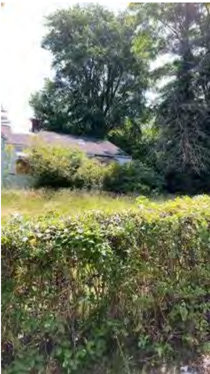
Figure C-7. Project 609440, Segment 1: Fire damaged house behind hedge row
