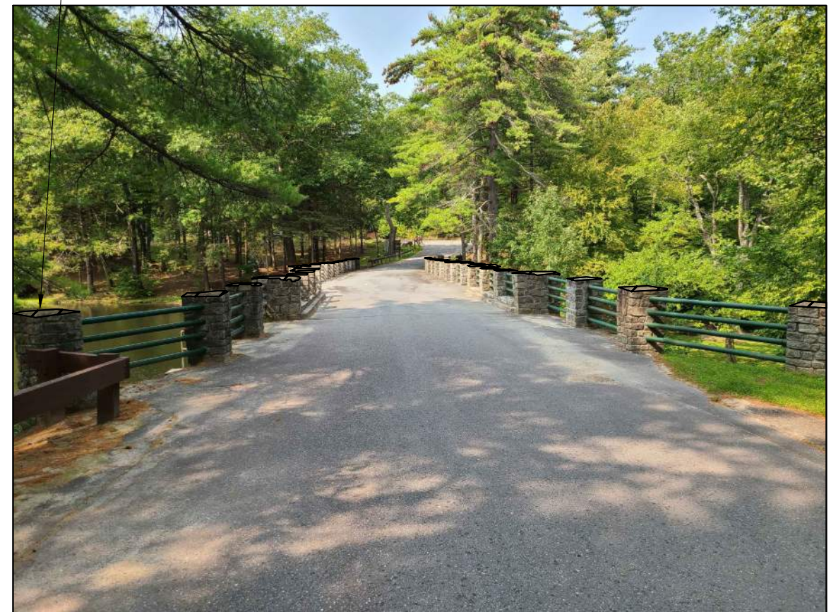
PHOTO 1 DAM AND BRIDGE LOOKING NORTHWEST ALONG HOSMER ROAD
