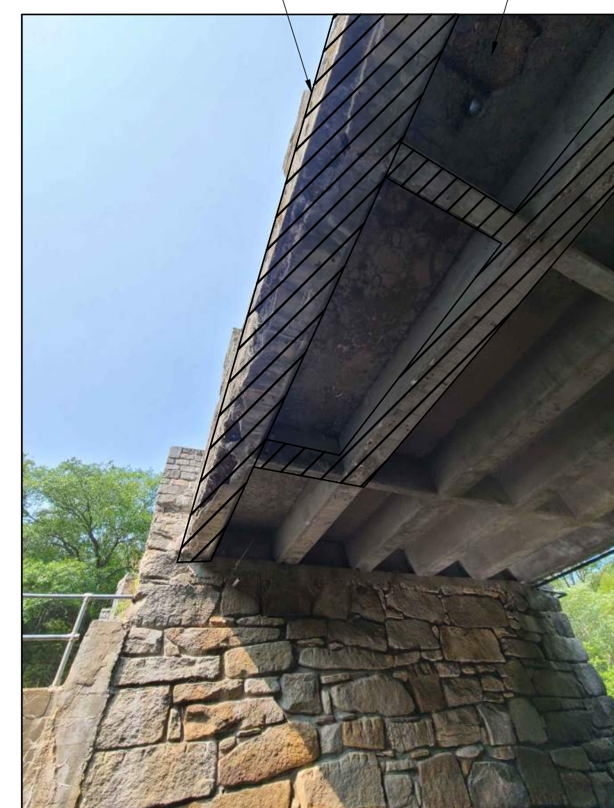
PHOTO 5 NORTHWEST BUTTRESS AND SOUTHERN SPANDREL BEAM
