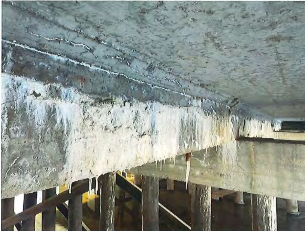
Photo 3: North deck fascia in span 3.
