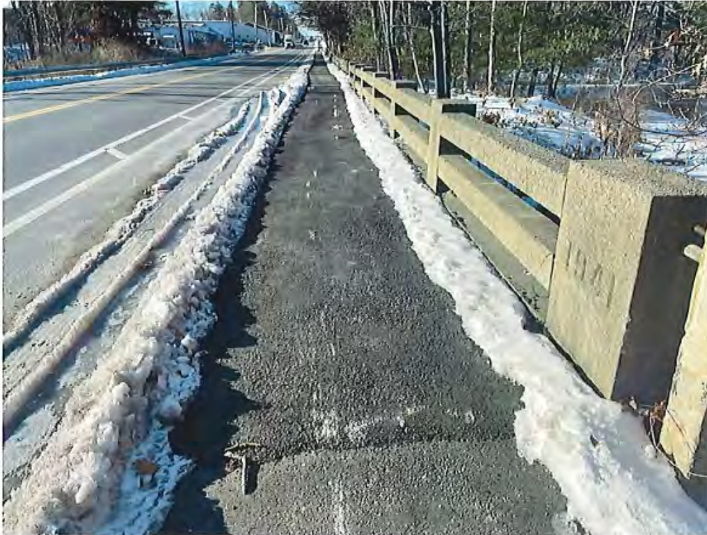
Photo 11: New north sidewalk pavement.
