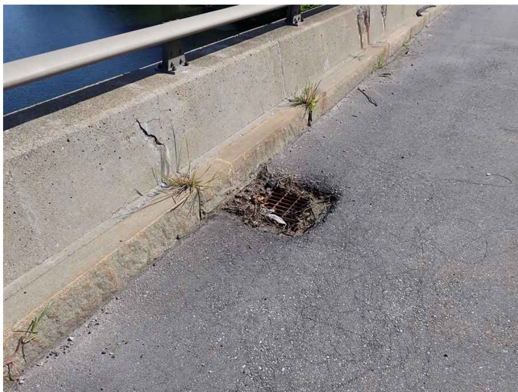
Photo 12: Span 4 north drainage grate, looking northeast. Typical condition.
