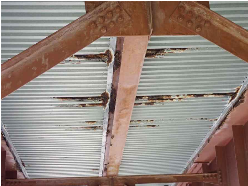
Photo 8: Span 4 bays 5 & 6 near west end, looking west.
