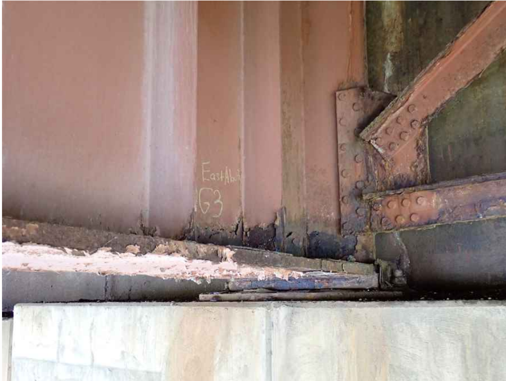
Photo 19: Span 4 girder 2 east end south face (east abutment).
