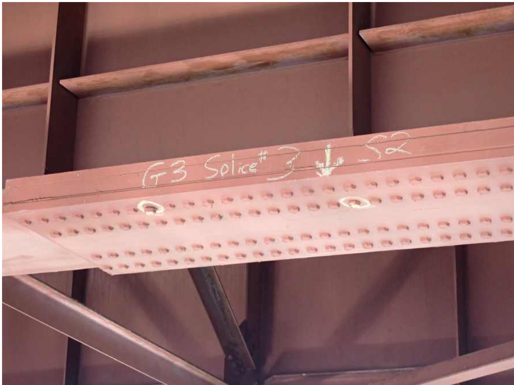
Photo 26: Span 2 girder 2 splice 3, looking northwest.
