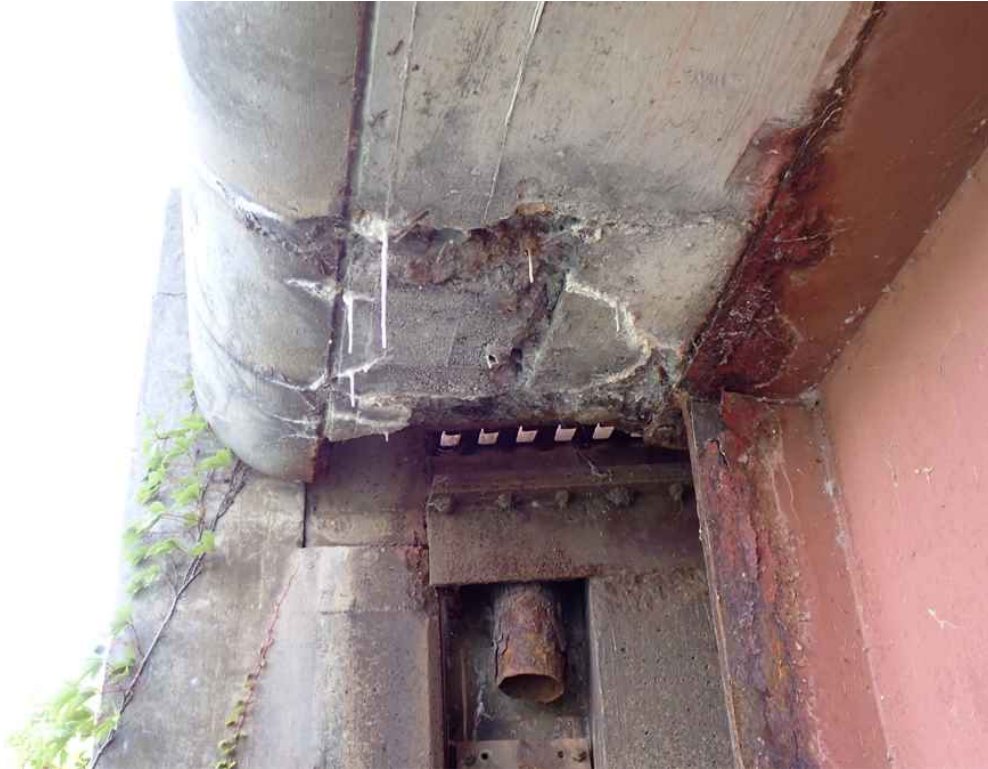
Photo 5: Span 4 north soffit east end, looking east. Note short drain.
