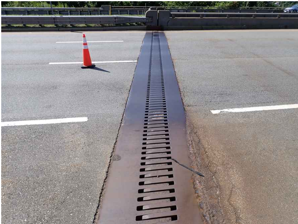
Photo 14: East abutment finger joint, looking south.
