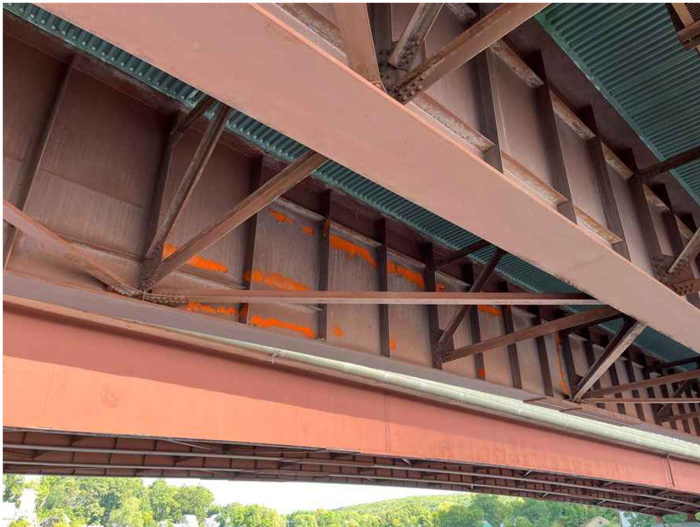
Photo 26: Span #2, girder #5 inside face.
