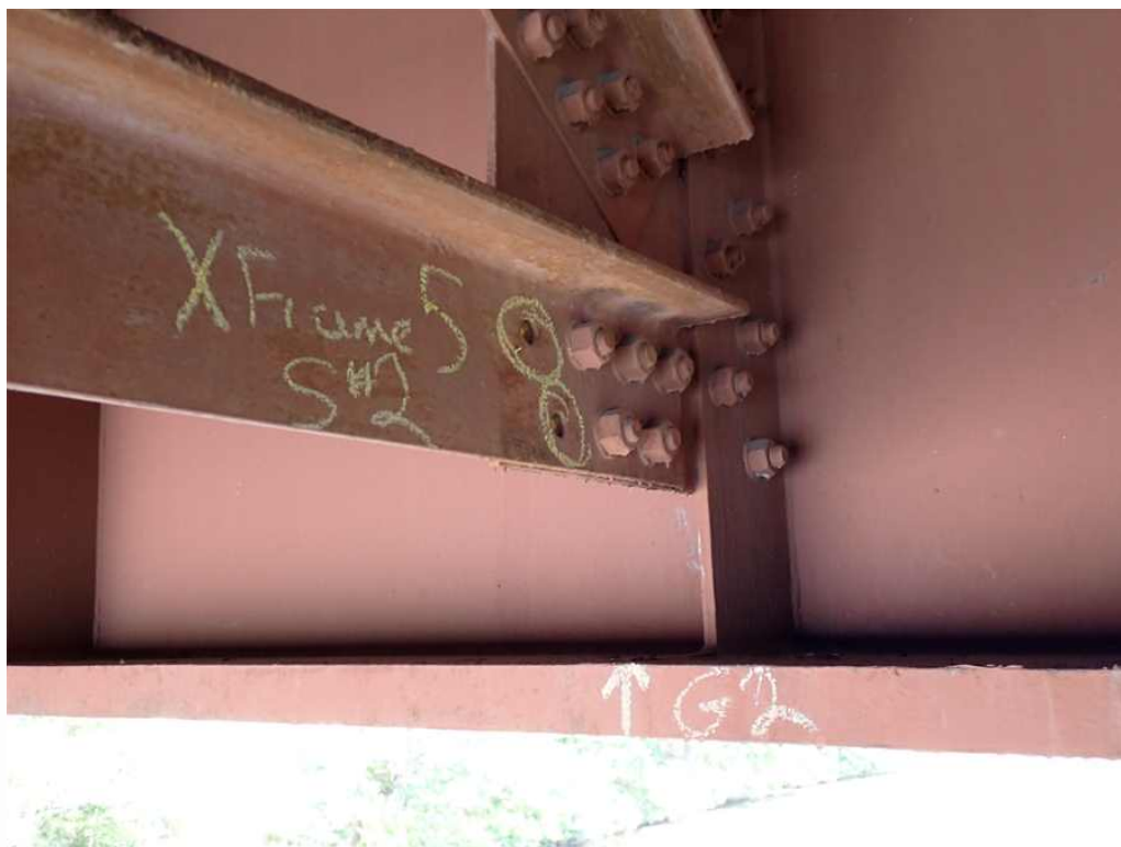
Photo 27: Span 2 girder 3 bay 5 cross frame 5 connection, looking northwest.
