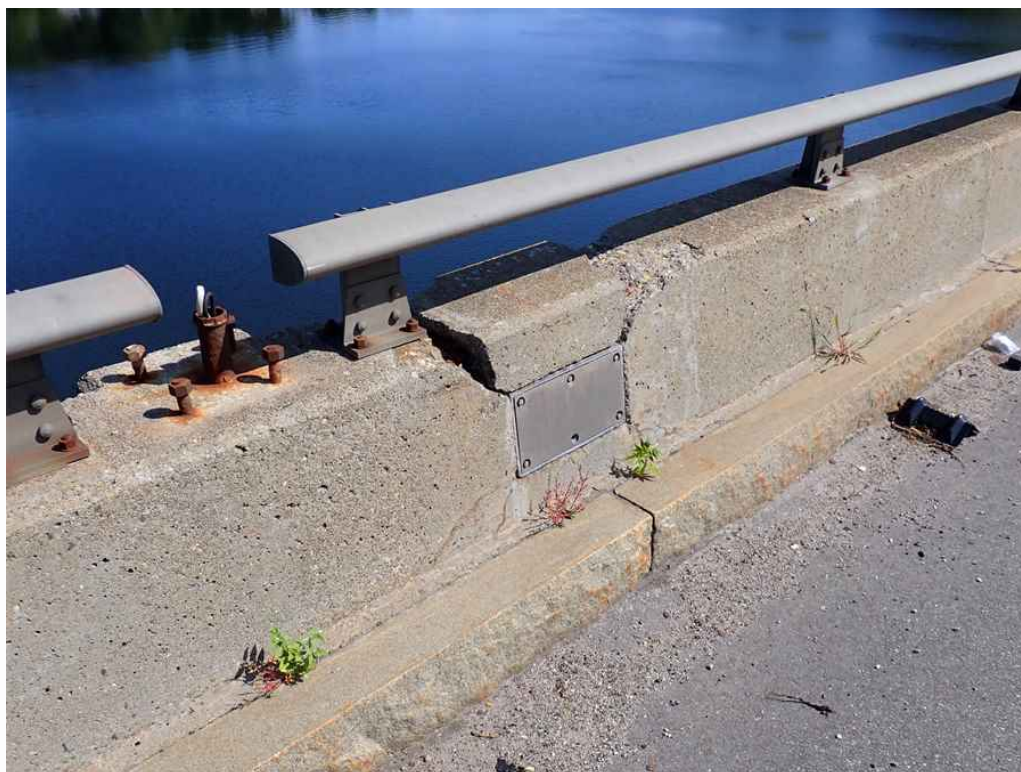
Photo 11: Span 3 north parapet near midspan, looking northeast.
