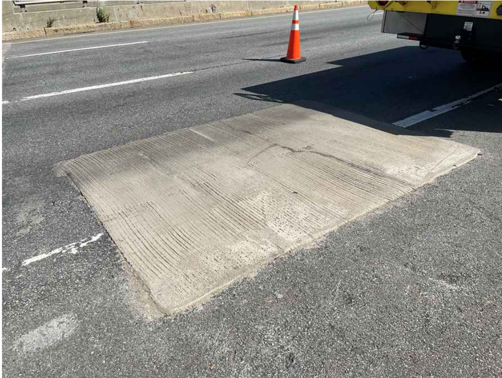
Photo 1: Concrete patch in span #1, right lane.
