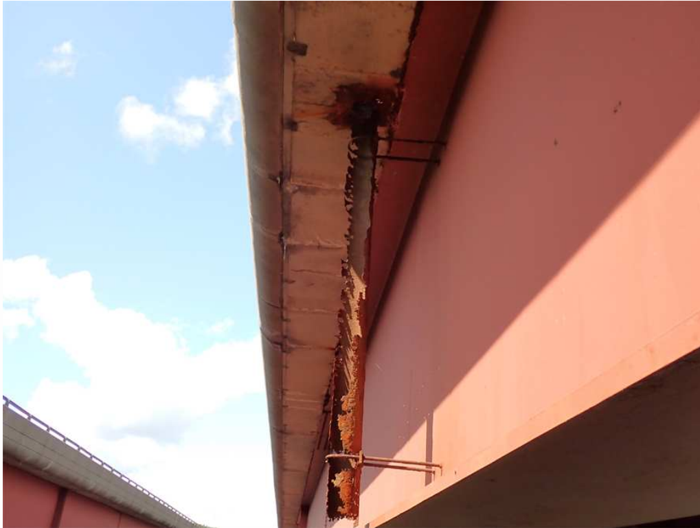
Photo 13: Span 4 midspan south scupper, looking west. Typical scupper condition outside span 1.
