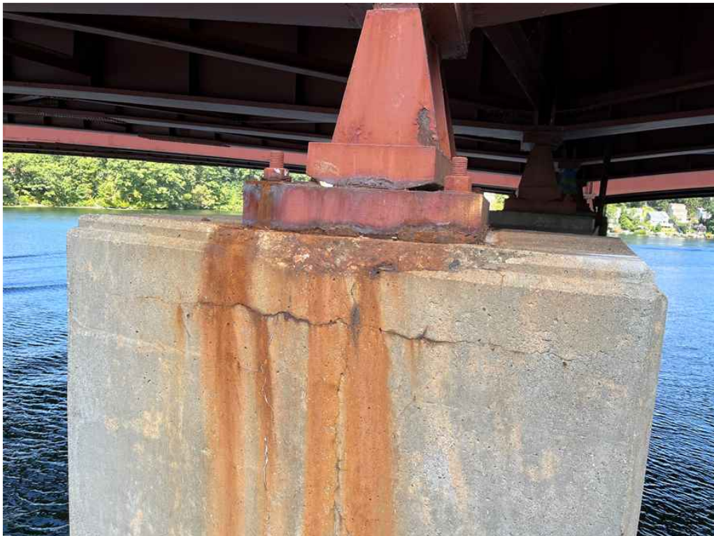
Photo 30: Pier #3 south face.
