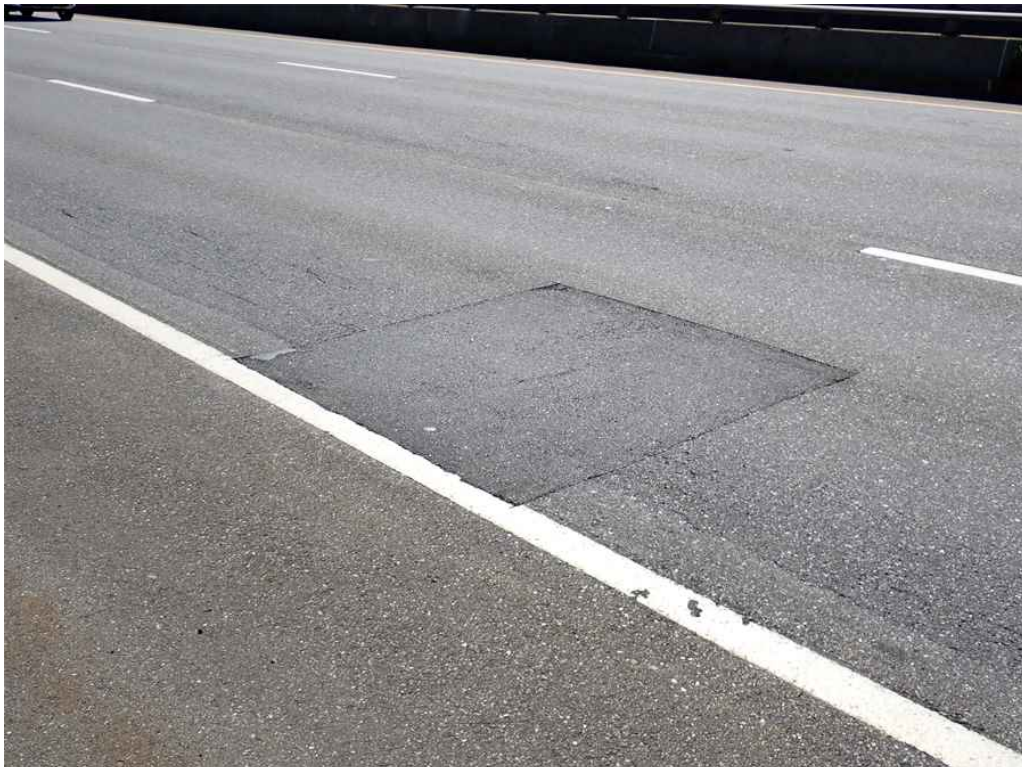
Photo 2: Wearing surface span 3 right lane near pier 3, looking southeast.
