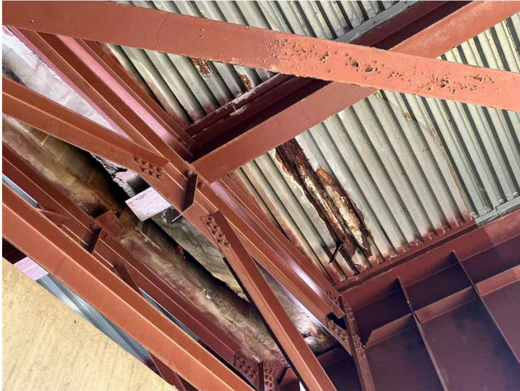
Photo 5: SIP forms in span #1, bays #5 and #6 at the east end.
