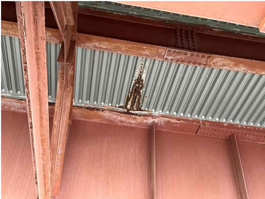
Photo 6: Bay #1, span #1 west of the splice.
