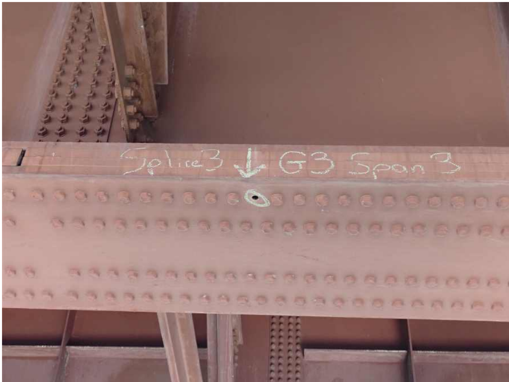
Photo 30: Span 3 girder 2 splice 3, looking north.
