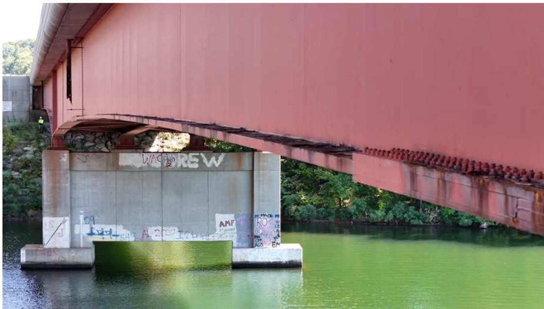
Photo 18: Span #3, girder #5, top face of bottom flange.
