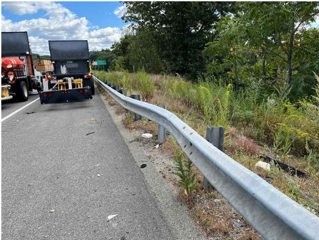
Photo 32: Southwest approach guardrail.
