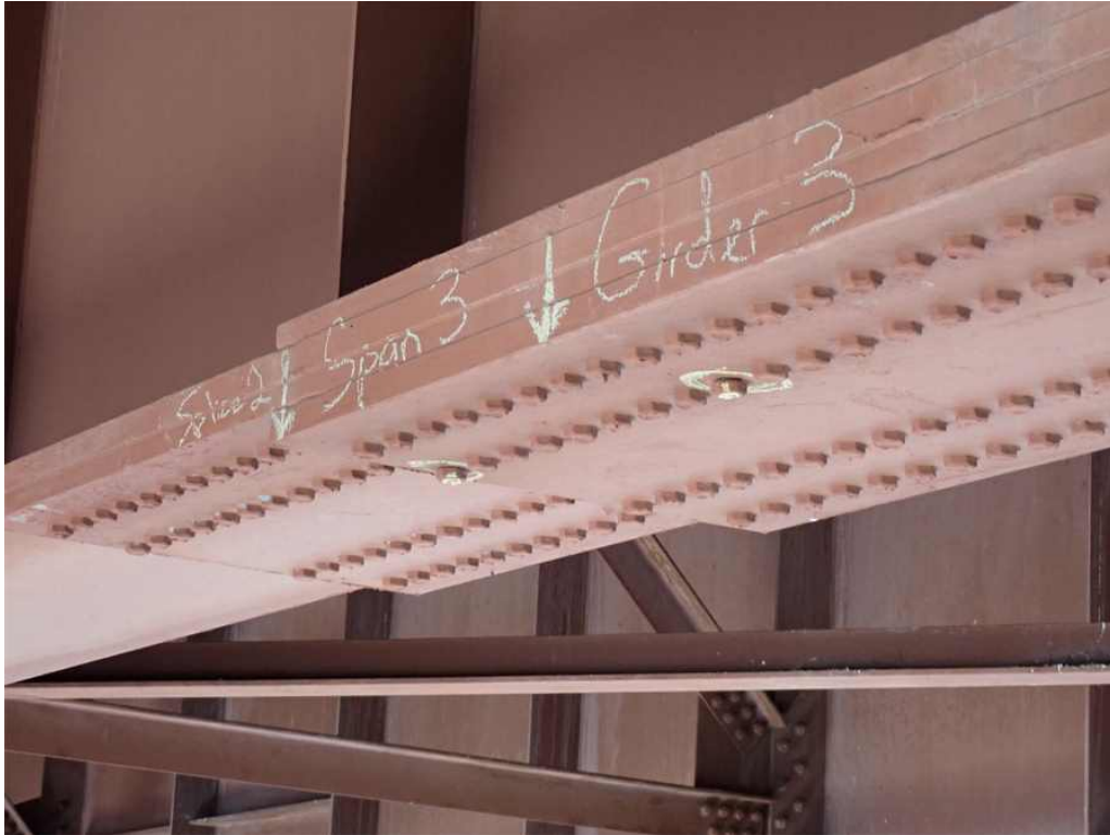
Photo 29: Span 3 girder 2 splice 2, looking northwest.
