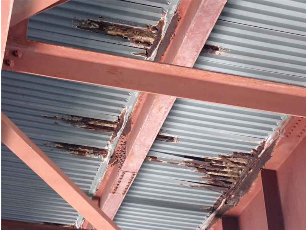
Photo 7: Span 2 bays 1 & 2 near midspan, looking northwest.
