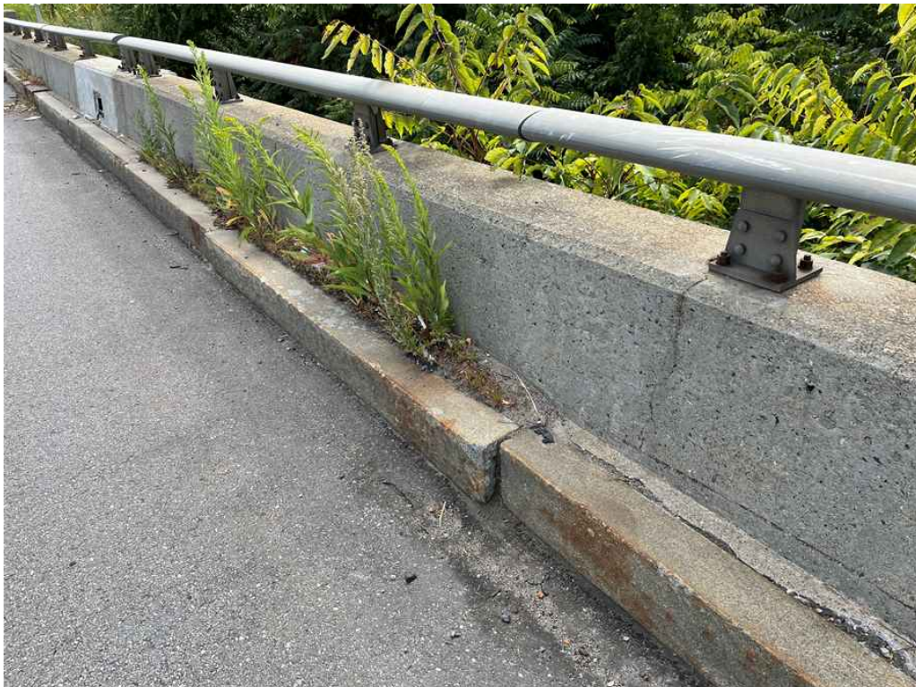
Photo 8: Typical condition of the curb. Span #4 shown.
