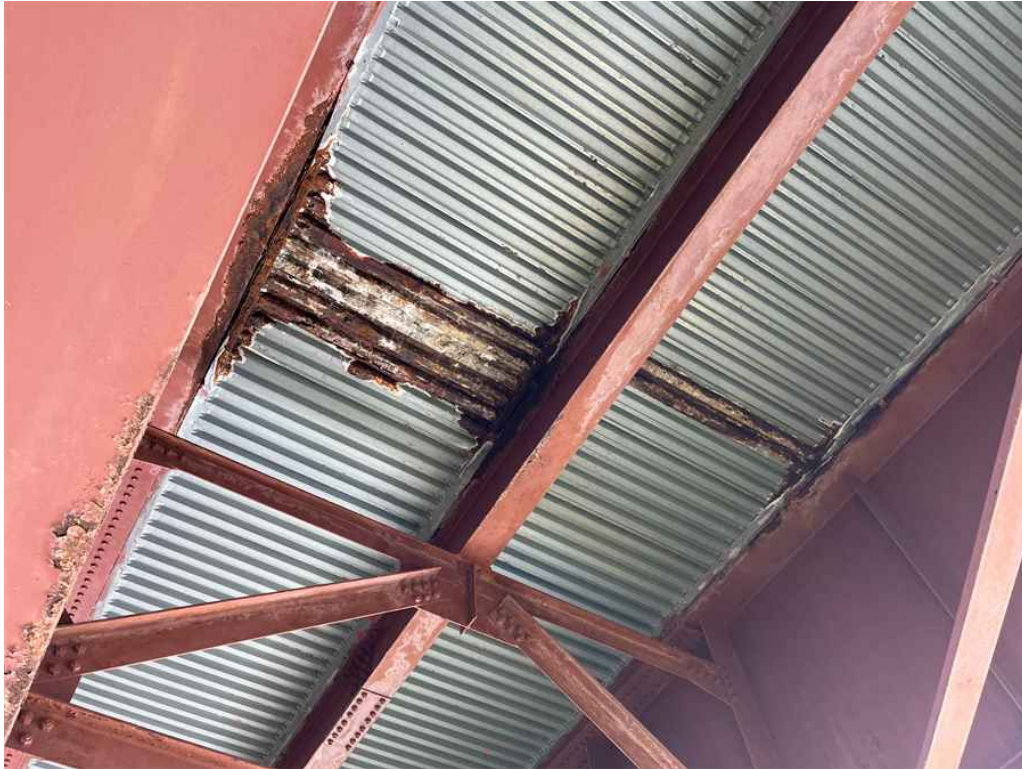
Photo 7: Bays #5 and #6 in span #2, west of the splice plate.
