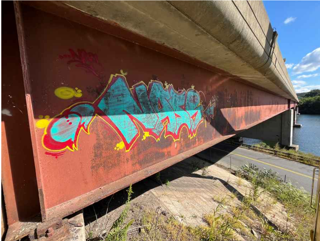
Photo 25: Span #1, girder #16 exterior face.
