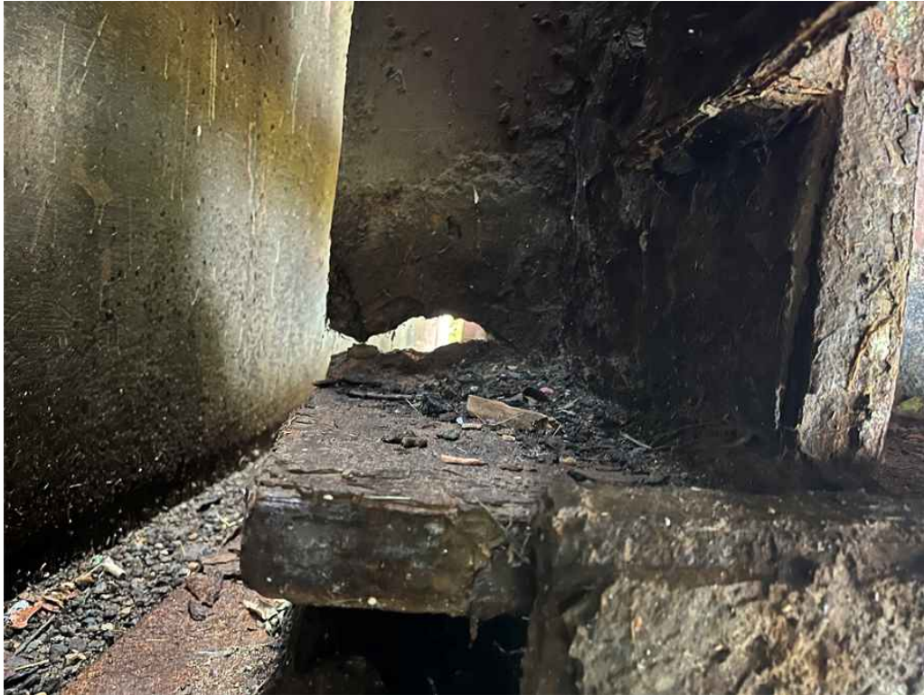
Photo 19: Span #4, girder #7 at the east end.
