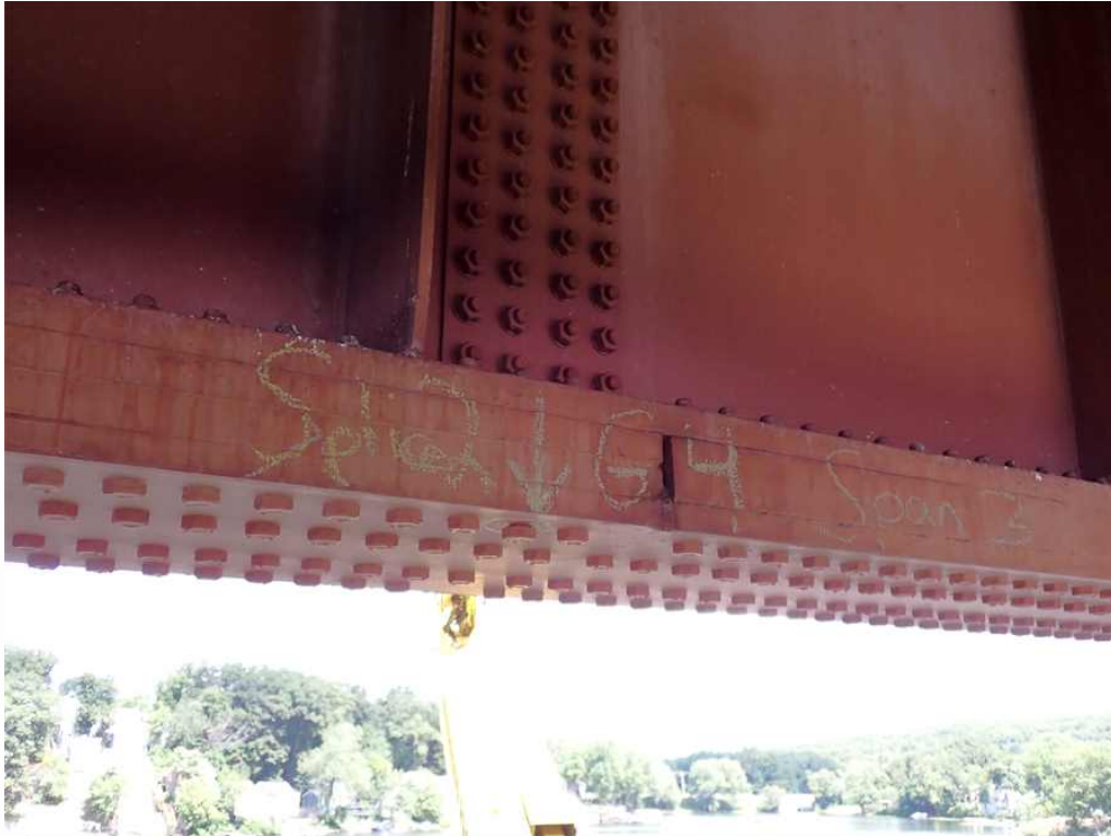
Photo 31: Span 3 girder 1 splice 2, looking northeast.
