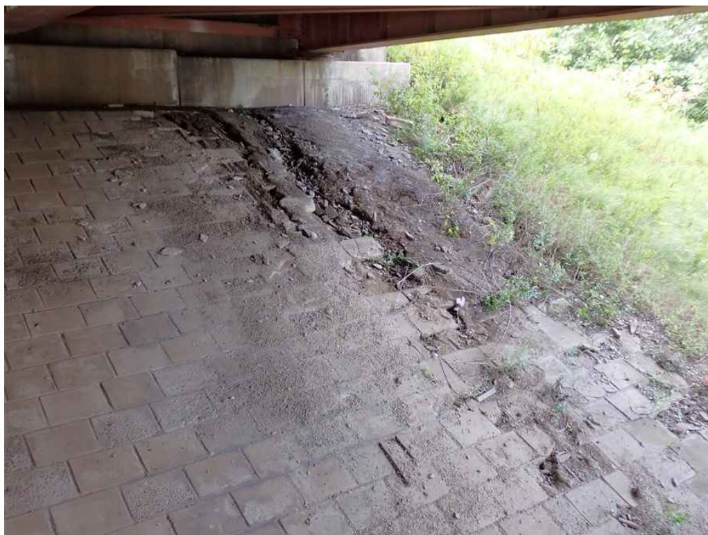
Photo 35: West abutment slope north end, looking northwest.
