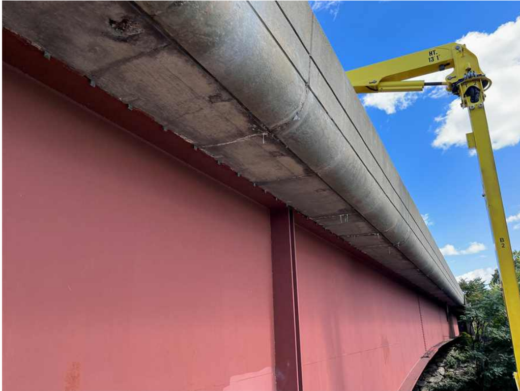
Photo 3: Spans #3 and #4 at pier #3.
