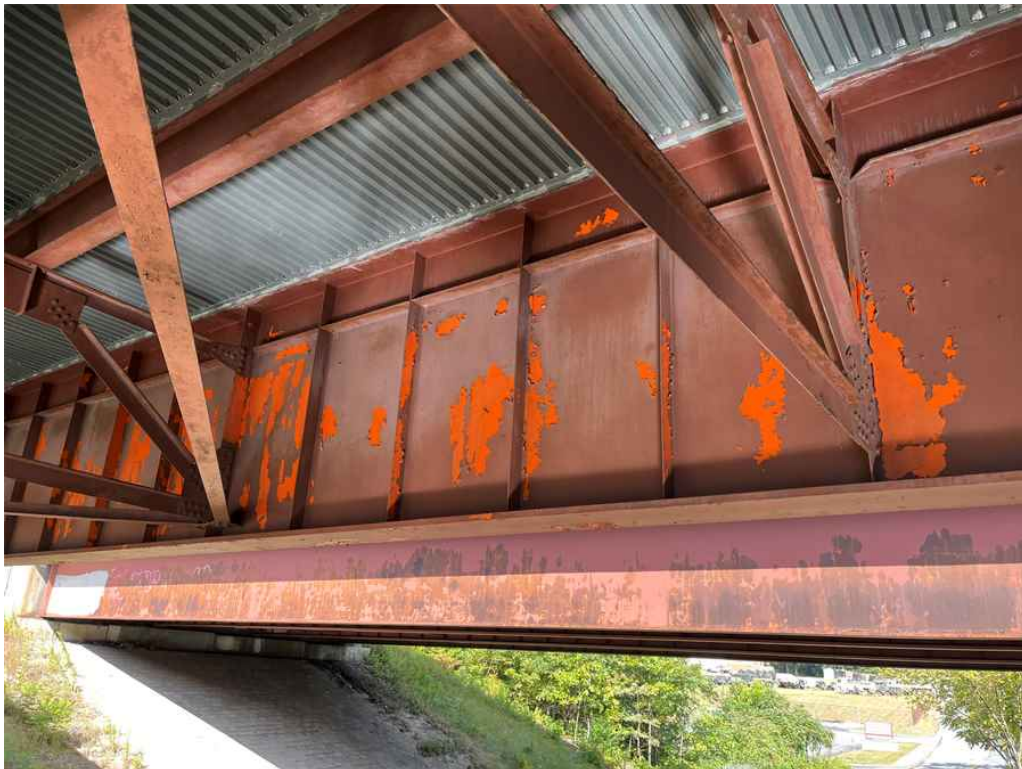
Photo 24: Span #1, girder #13 inside face.
