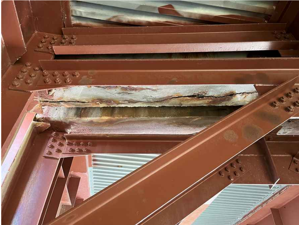
Photo 21: Concrete end diaphragm condition over pier #1.
