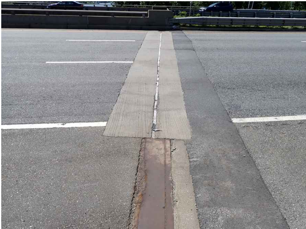
Photo 16: West abutment joint, looking south. Travel lanes removed/replaced since previous inspection.
