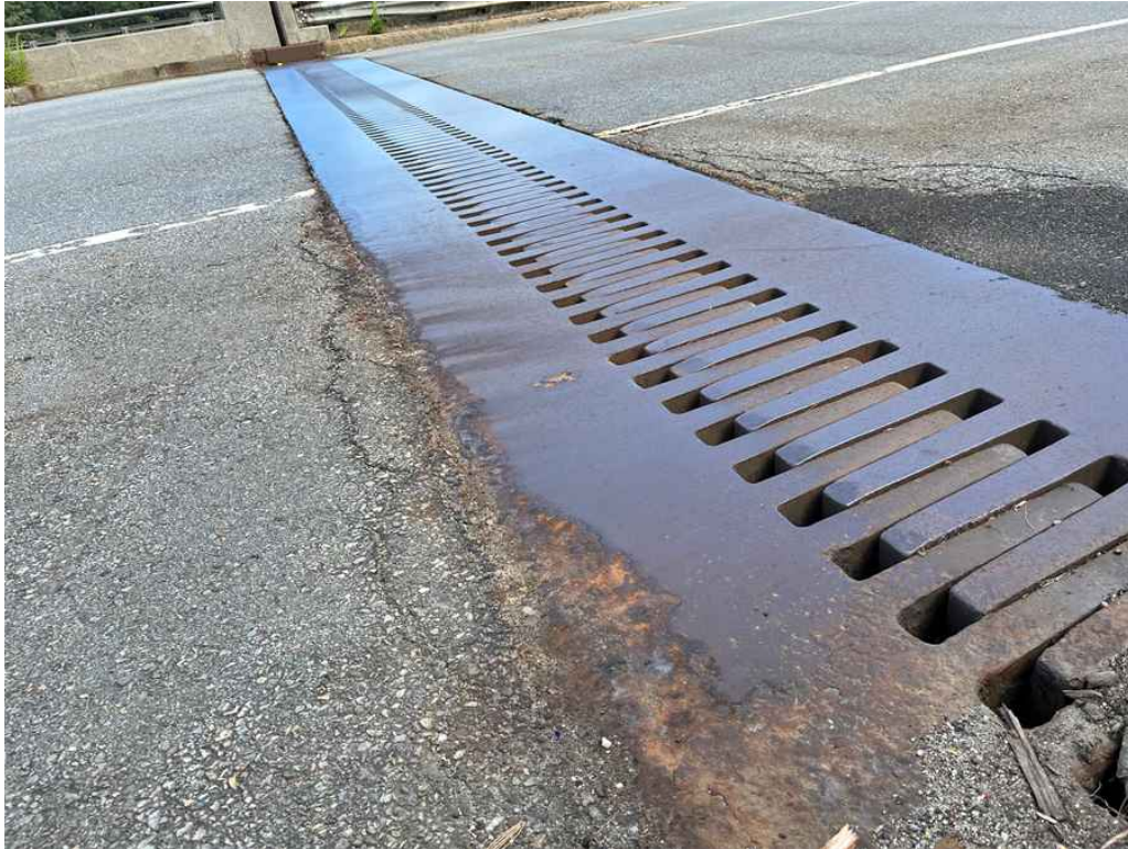
Photo 15: East finger joint at the south end.
