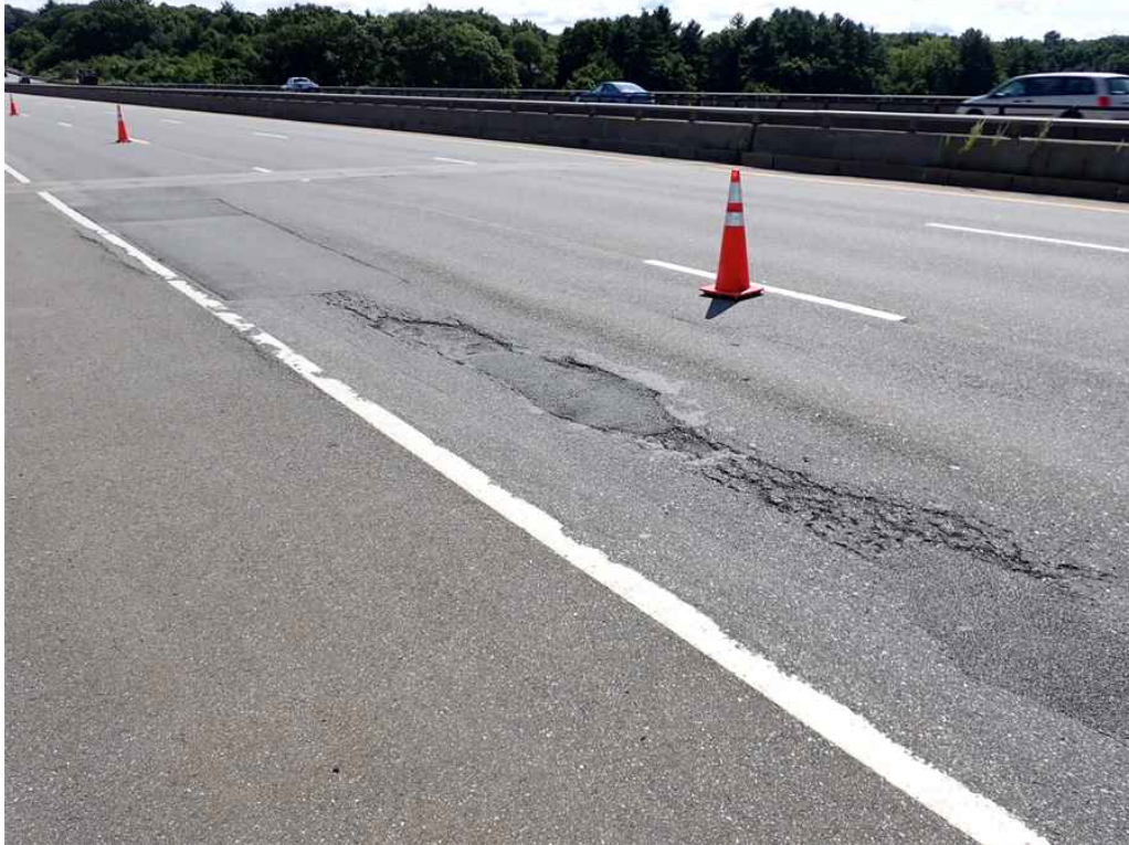
Photo 1: Wearing surface span 1 east end, looking southeast.
